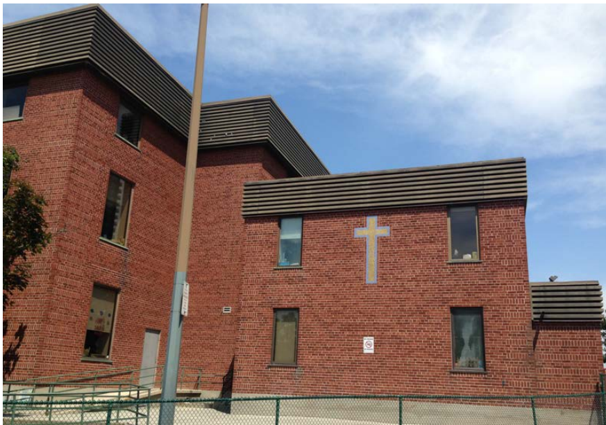
14. South and east elevations of the former school with the main block and the two storey entry wing. The metal cornices were added with the extension of the Columbus Centre (HPS, 2018)
