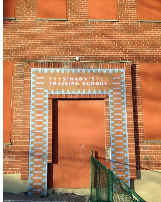
15. South elevation, of the main block of the former school looking toward the east corner showing the blocked in windows and the brick details of vertical headers on the corners suggesting giant piers, above left. (HPS, 2018)
