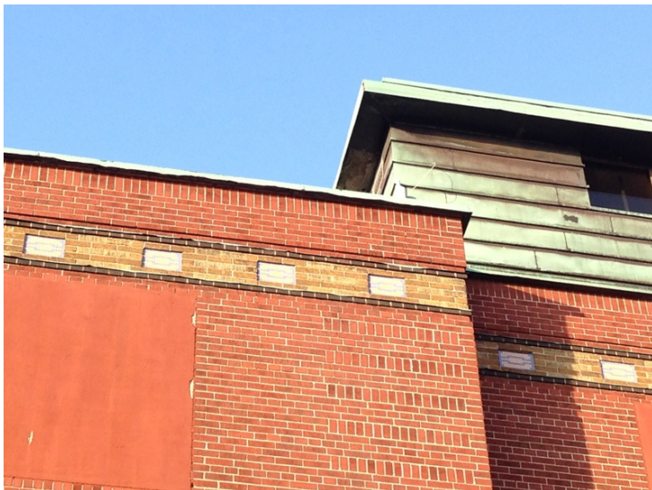
17. Upper level of the south elevation showing the brick detailing and the brick and tile frieze with the copper cladding of the service tower of the former school (HPS, 2018)
