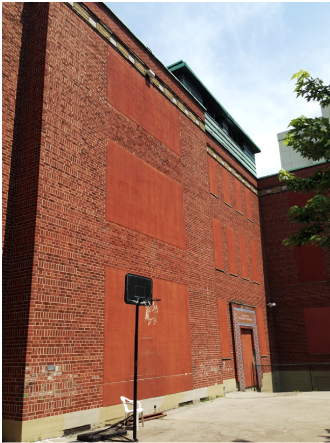
15. South elevation, of the main block of the former school looking toward the east corner showing the blocked in windows and the brick details of vertical headers on the corners suggesting giant piers, above left. (HPS, 2018)
