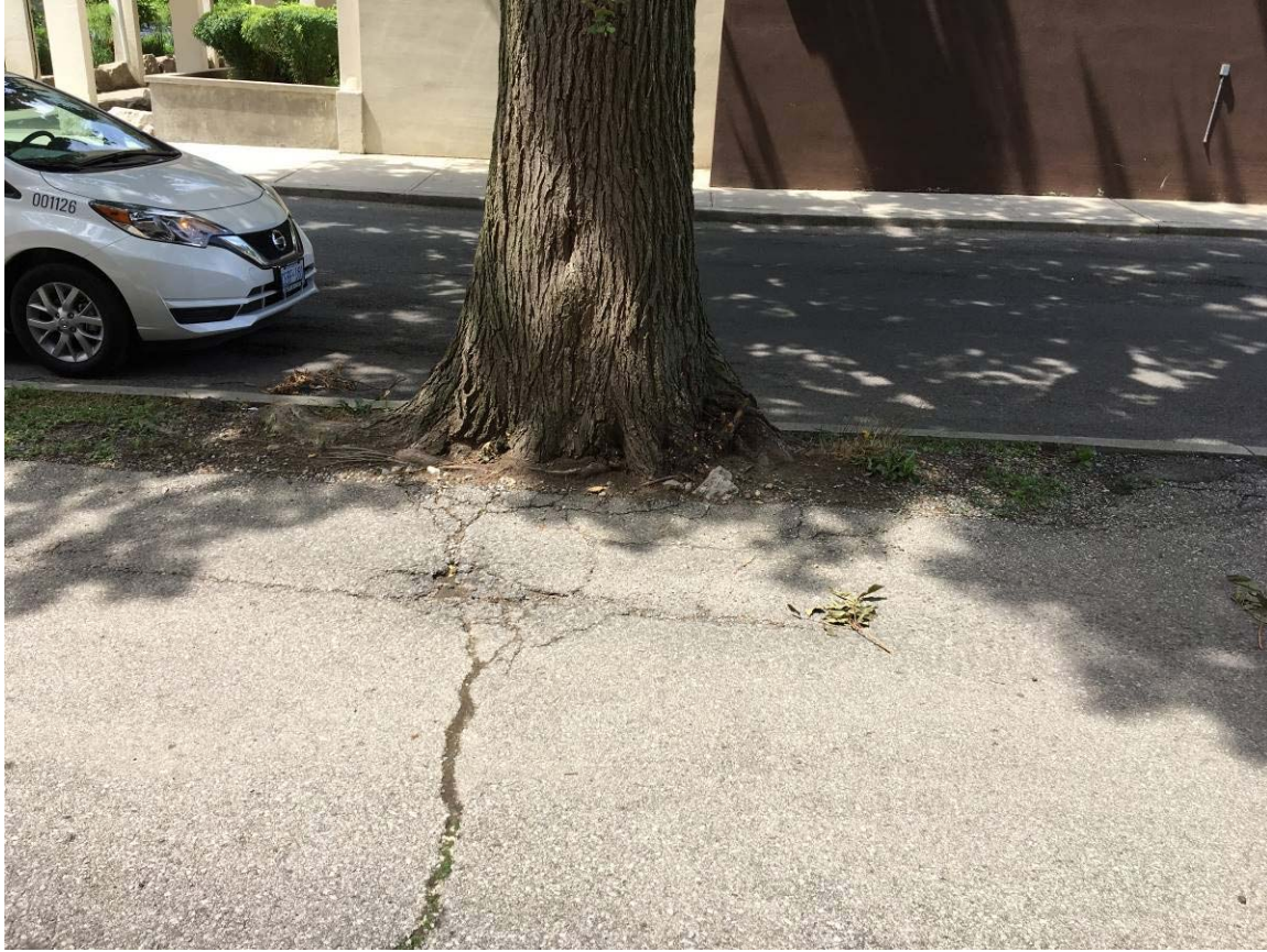
Attachment 3 – Photograph of the subject tree's trunk flair from the east looking west, showing the cracks of concern in the 168 Erskine Avenue driveway
