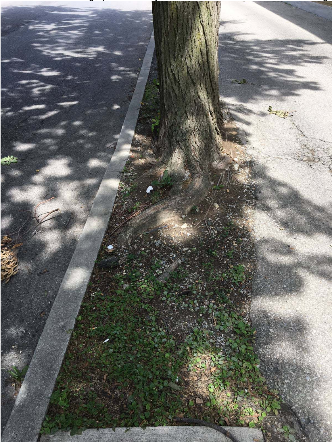
Attachment 2 – Photograph of the subject tree's trunk flair from the south looking north
