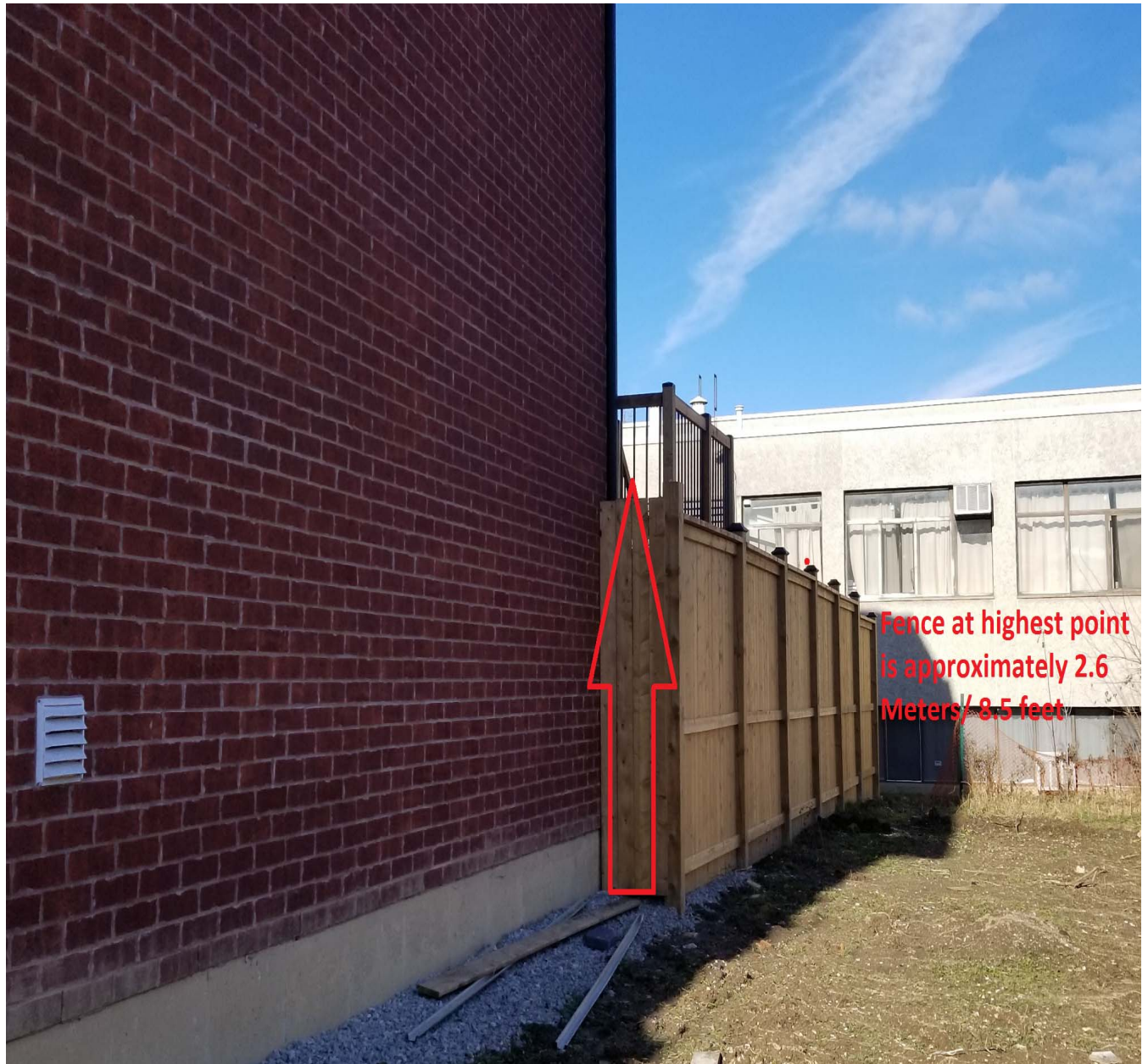
Attachment 4: View East side of property.
