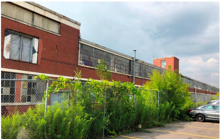
North elevation showing the raised east end and elevator towers in contrast to the horizontal ribbon windows of factory sash glazing (HPS, 2019)
