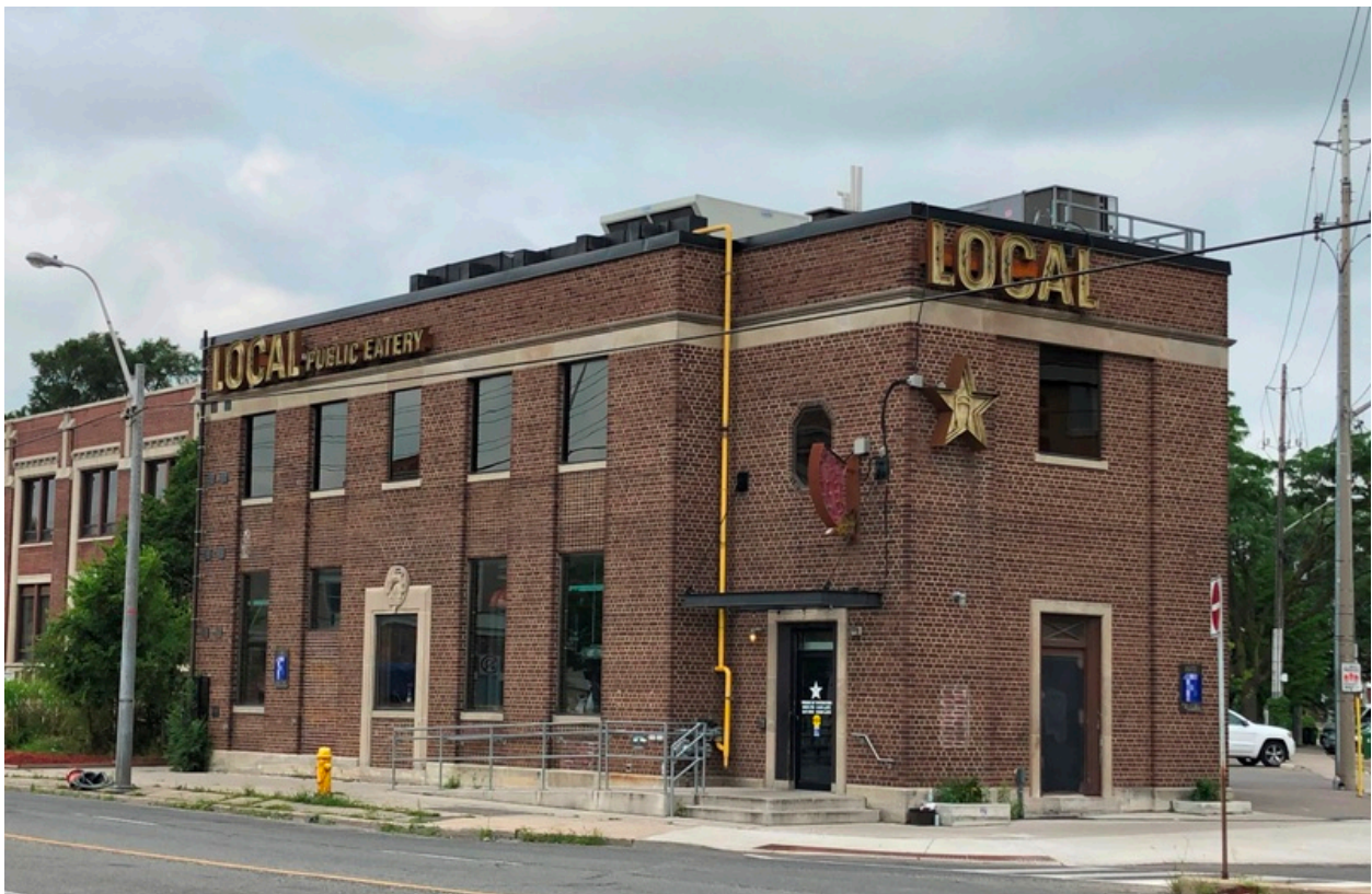
180 Laird Drive, originally the Imperial Bank of Canada, 1941 principal (east) and north elevations (HPS, 2019)
