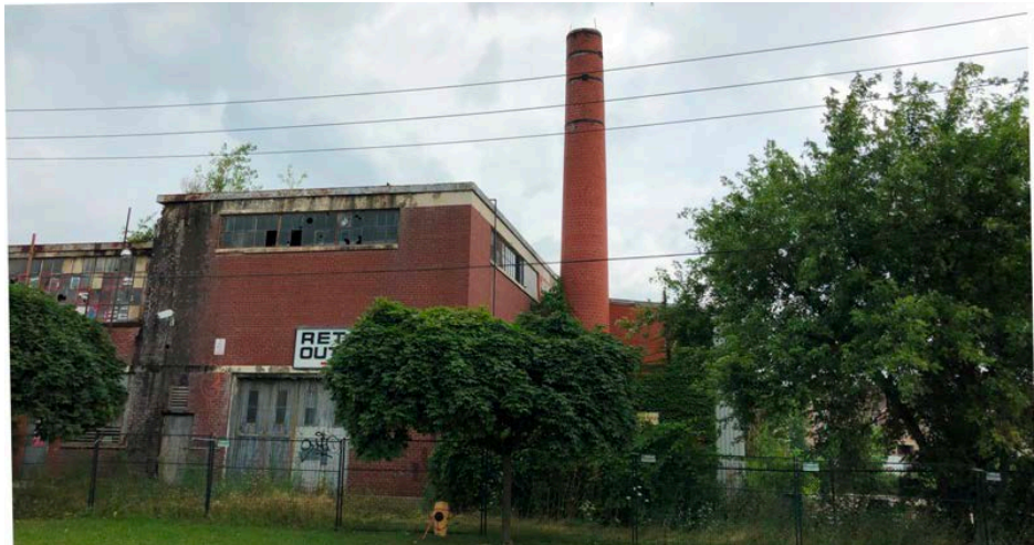
South and east elevations with the raised east end and later additions behind chimney (HPS 2019)
