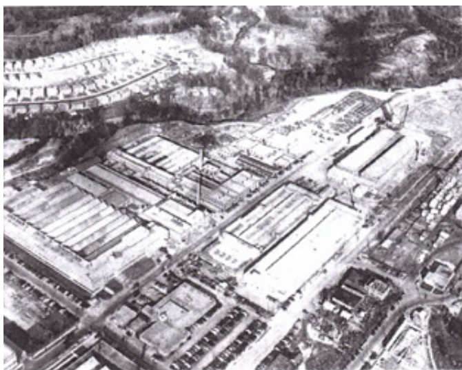
Research Enterprises Ltd (REL) at Leaside, over Brentcliffe Road. Eglinton Avenue East has not yet been extended over the Don Valley. Rykert and Thursfield Crescents can be seen in the background. 1944.
