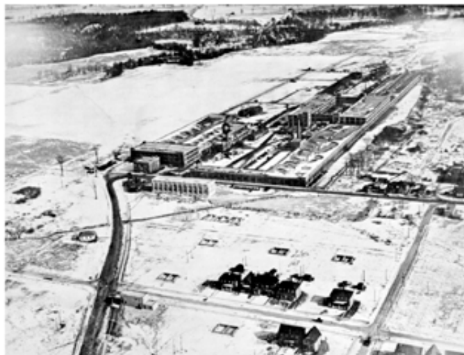
10. 1931 Aerial Photograph looking north east at the junction of Laird and McRae Drives with the Durant Motor Complex and in the foreground the few houses that had been constructed on the west side of Laird Drive by this date. The single storey white-clad, hipped roof on the north side of McRae Drive is the first Imperial Bank of Canada, which was replaced in 1941 by the a new building at 180 Laird Drive (Rempel, p. 35)
