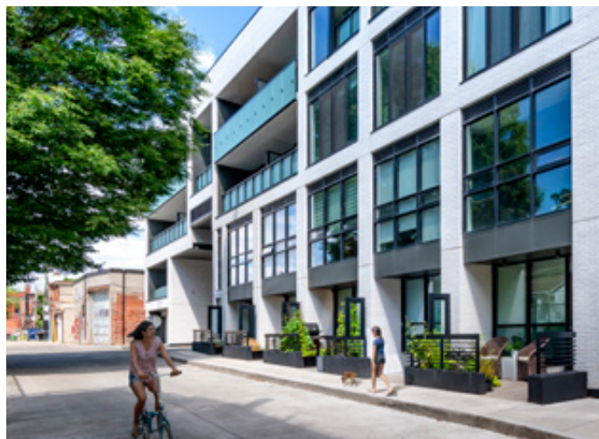
Mid-rise buildings along Laird Drive will positively interface with adjacent residential neighbours, and ensure service accesses are designed as high quality extensions of the public realm.
