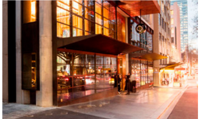
A high quality designed retail frontage in Melbourne, Australia incorporates fine details and canopies to delineate retail frontages. Mullions break large expanses of glazing, and could help buildings fit in with the industrial aesthetic of the adjacent Leaside Employment Area.
