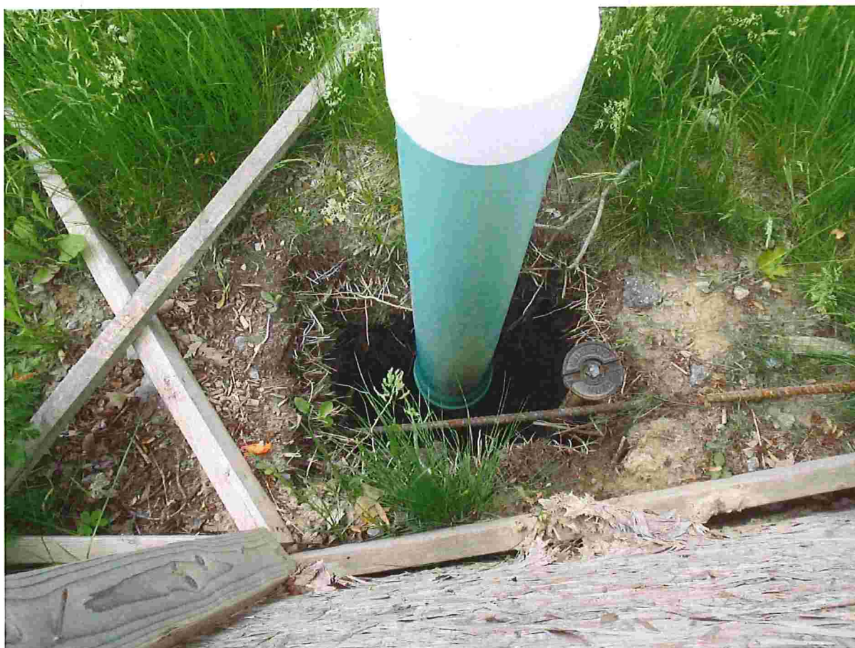
Pic 3. Waste water sewer and water services installation in mTPZ of tree. Note exposed roots left unpruned in exposed pit. Work performed by City contractor.
