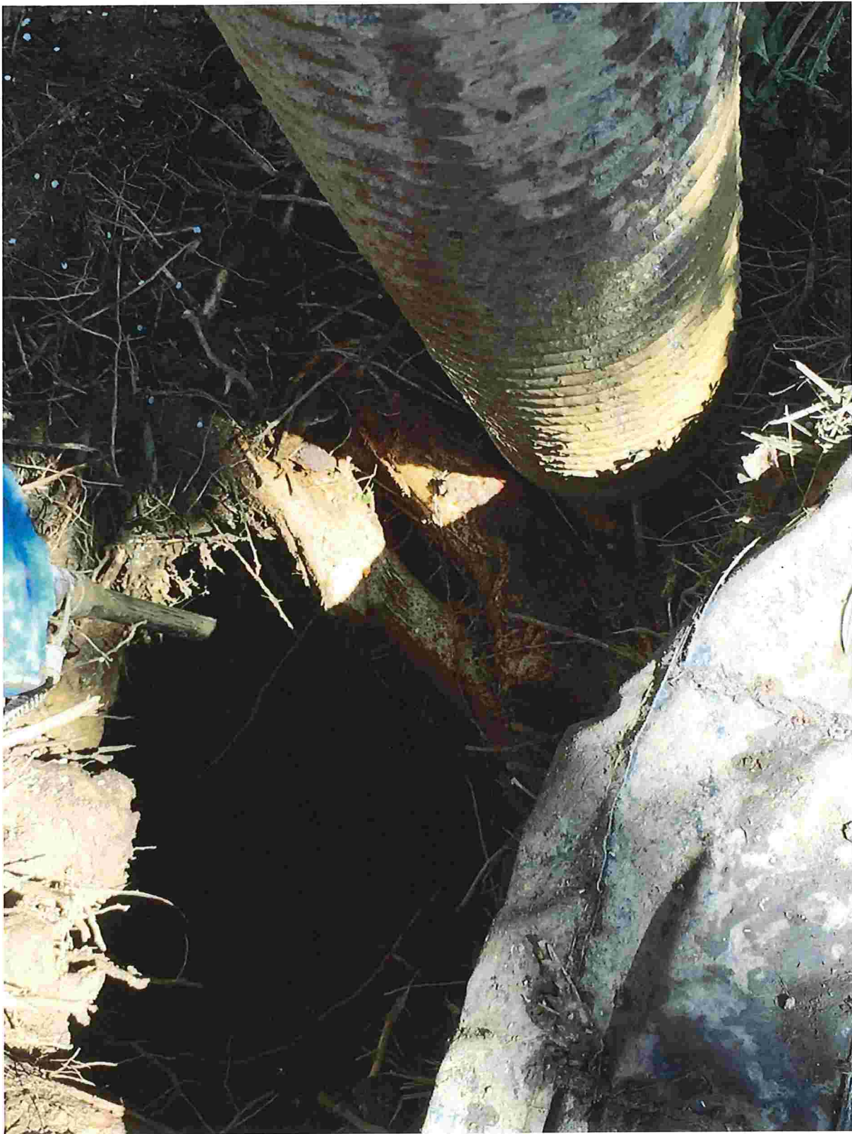
Pic 2. Tree 1. Vertical excavation by City to install clean out pipes for services. Note extensive structural roots in center of picture.
