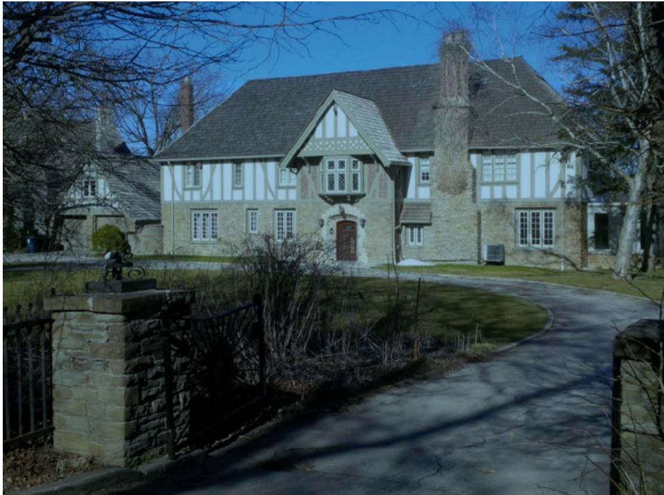
Photograph of 35 Kingsway Crescent, principal (south) elevation. (Neil Park, Etobicoke History Society, 2018)
