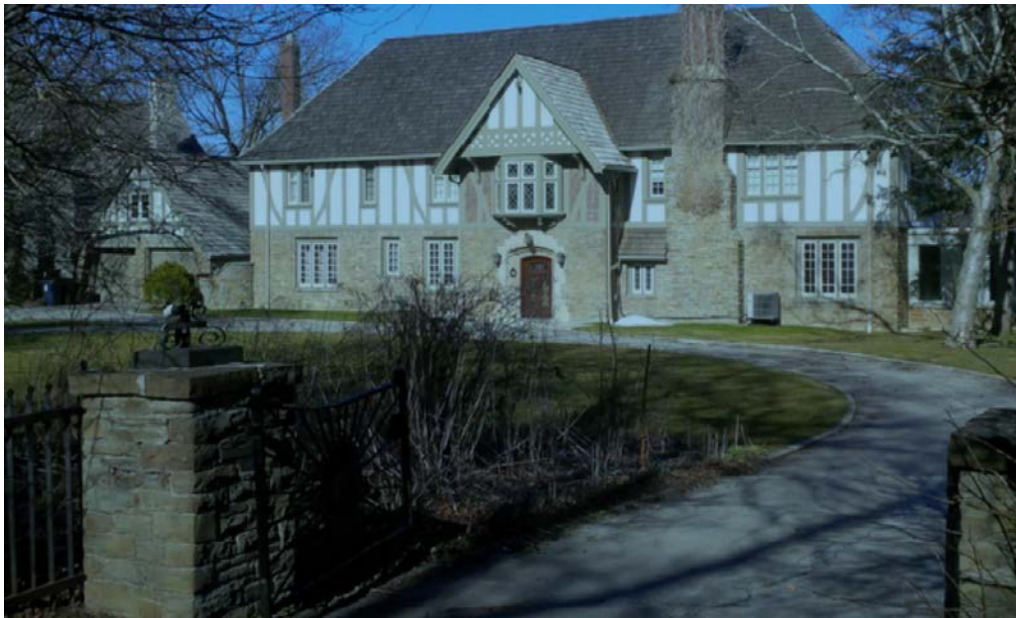
12. Pearce house, west elevation, 2018 showing the gate posts and sunroom extension at the south end of the house (right hand side of photograph) (Neil Park, Etobicoke History Society, 2018)
