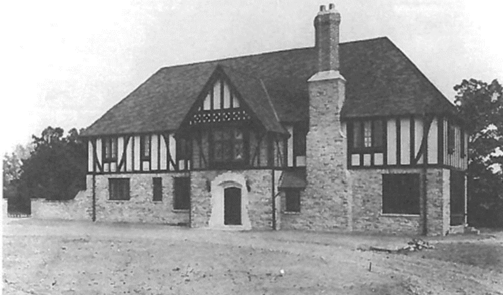
Photograph of the Pearce House shortly after its completion in 1929 (Metro Toronto Reference Library [MTRL] T34713)
