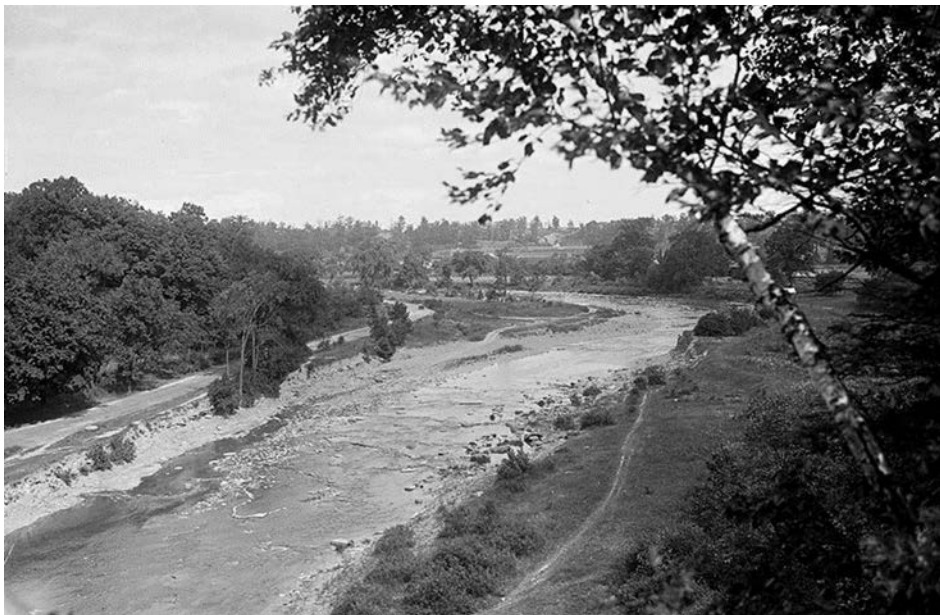
7. Photograph of the ridge where 35 Kingsway Crescent is located and showing the Humber river and the grand riverside boulevard planned by R. Home Smith and now known as Home Smith Park Road. (City of Toronto Archives [CTA] Fonds 1231, Item 1650, James Salmon Fonds)
