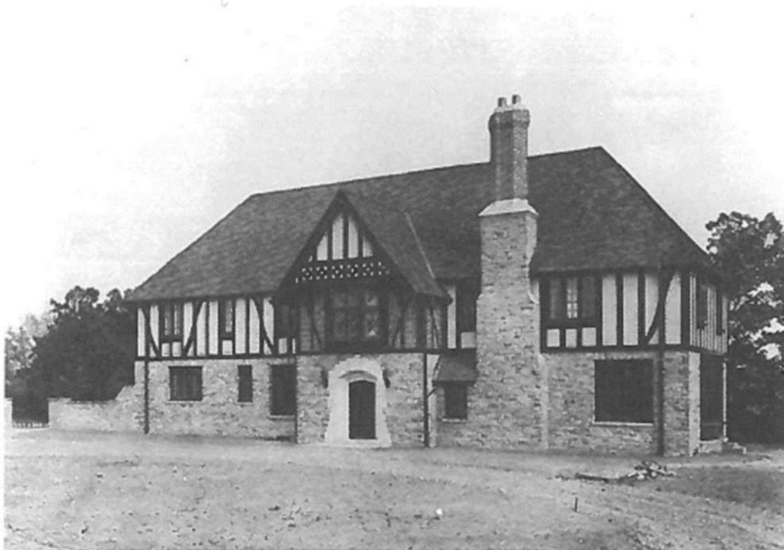
10. Pearce House shortly after completion in 1929 showing the principal, west, elevation (Metro Toronto Reference Library [MTRL] T34713)
