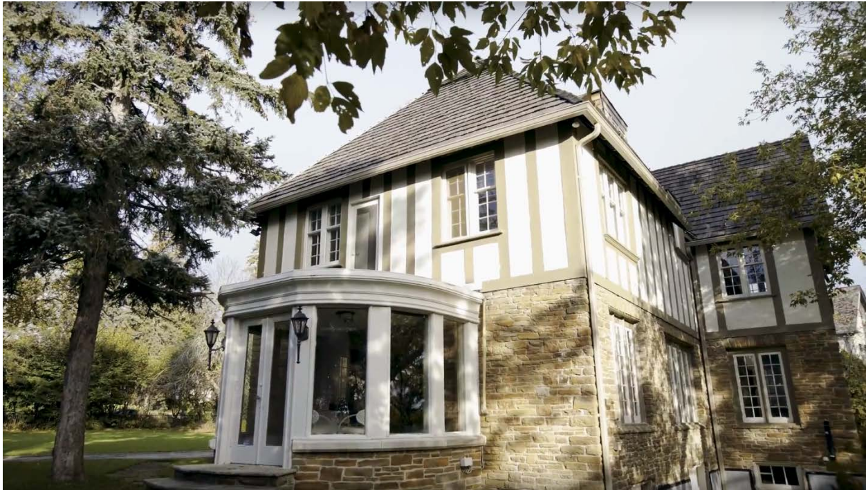
15. View of the south and east elevations showing the 1960 sun room extension. (Birdhouse Media, 2017)
