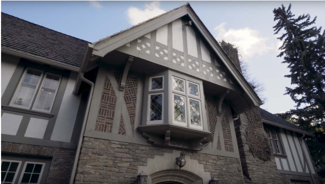
14. Photograph showing the bay window with its leaded and stained glass, the red brick nogging and the brackets support the jettied gable (Birdhouse Media, 2017)
