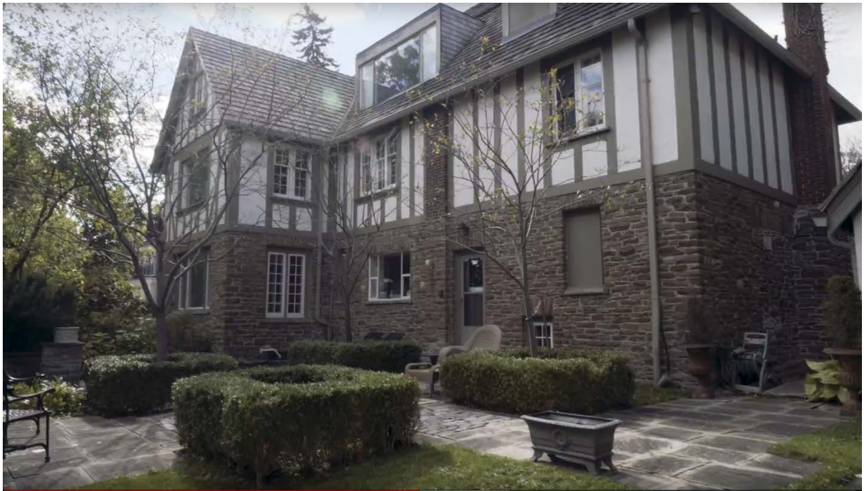
16. View of the east and north elevations with terraces (Birdhouse Media, 2017)
