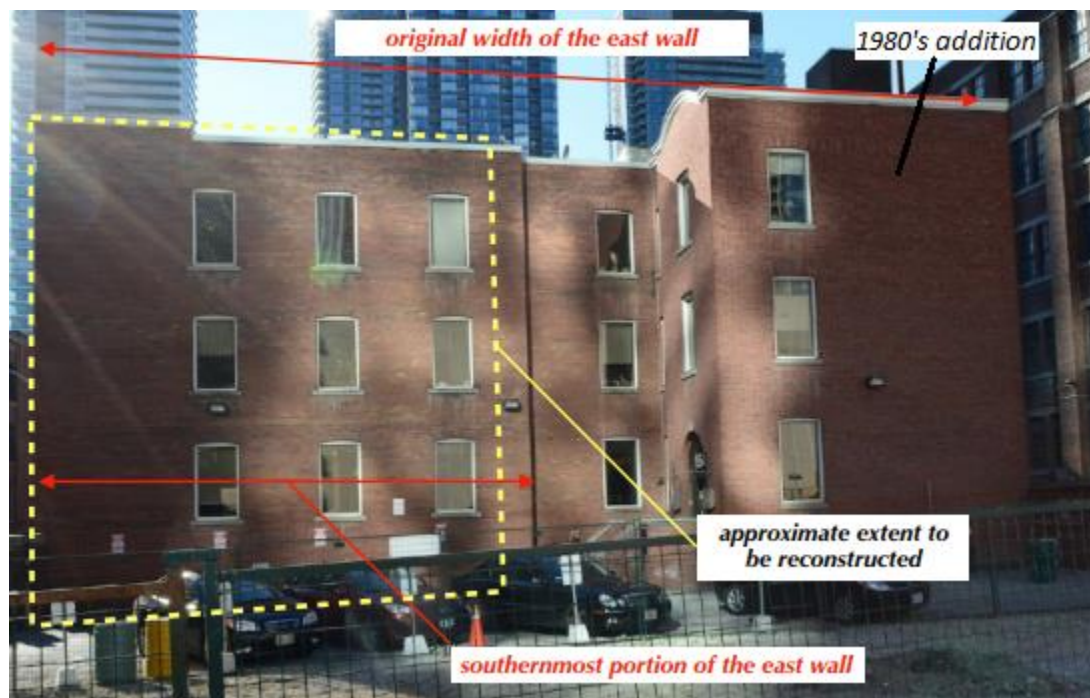
Extent of east wall (158 Pearl St) reconstruction
