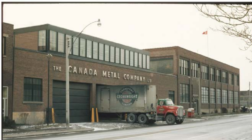
31. Canada Metal Company, detail of archival photograph showing the Shipping Building (F), 1946-9 with the shipping bays and the 1967 office extension at the second floor. (CTA Fonds 200, Series 1465, File 384, [1970-1985])
