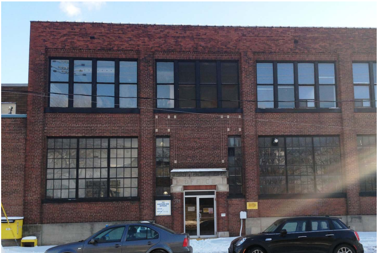
40. Main Building (A), principal (north) elevation, east end with entrance showing the factory sash glazing at the ground floor and double paned sash above (HPS, 2018)
