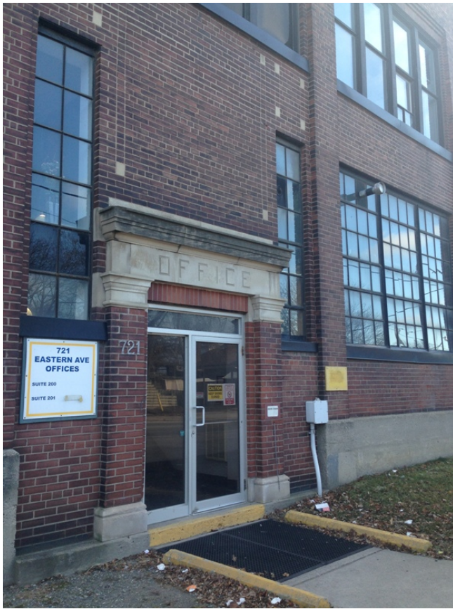
41 and 42. Main Building (A), Entrance Bay showing the concrete base beneath the piers (left) and the principal entrance on Eastern Avenue (right) (HPS, 2019)
