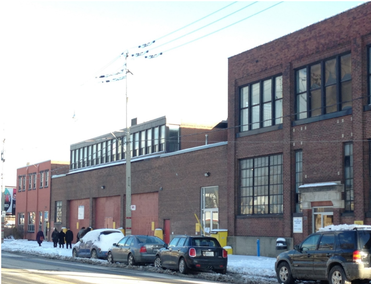
36. Principal (north) Elevations of Canada Metal Company showing the Comfort Building (E), far left, Shipping Building (F), 1946-9 with its upper level offices, 1967, centre, and the Main Building (A) at the right. (HPS, 2018)
