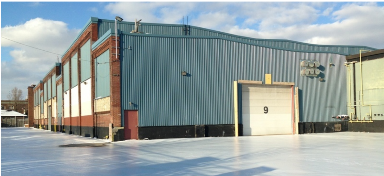
19. Photograph showing the side (west) elevations of the Main Building (B + C) and the rear (south) elevation of C which faced the railway line on Keating Street, later, Lakeshore Boulevard (HPS 2018)
