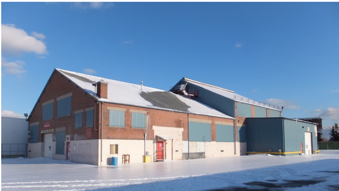
34. Oxide Mill Building (I): north and west elevations, demolished 2018 (HPS, 2018)
