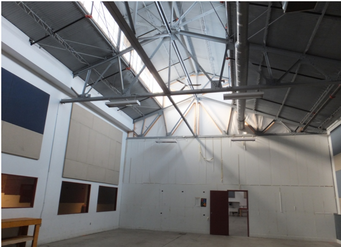
23. Building G, showing the internal space and metal structure (HPS, 2018)
