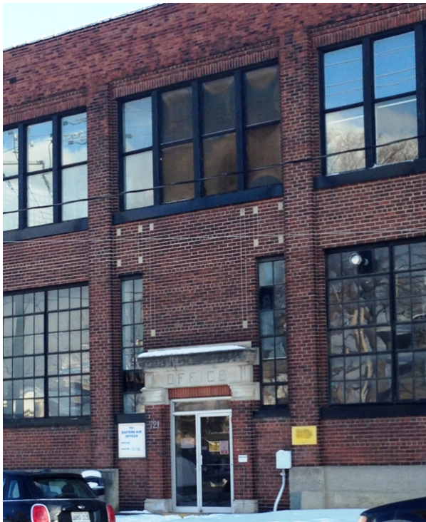
Photograph of the Main Building (A), main entrance on the principal (north) elevation (HPS, 2018)
