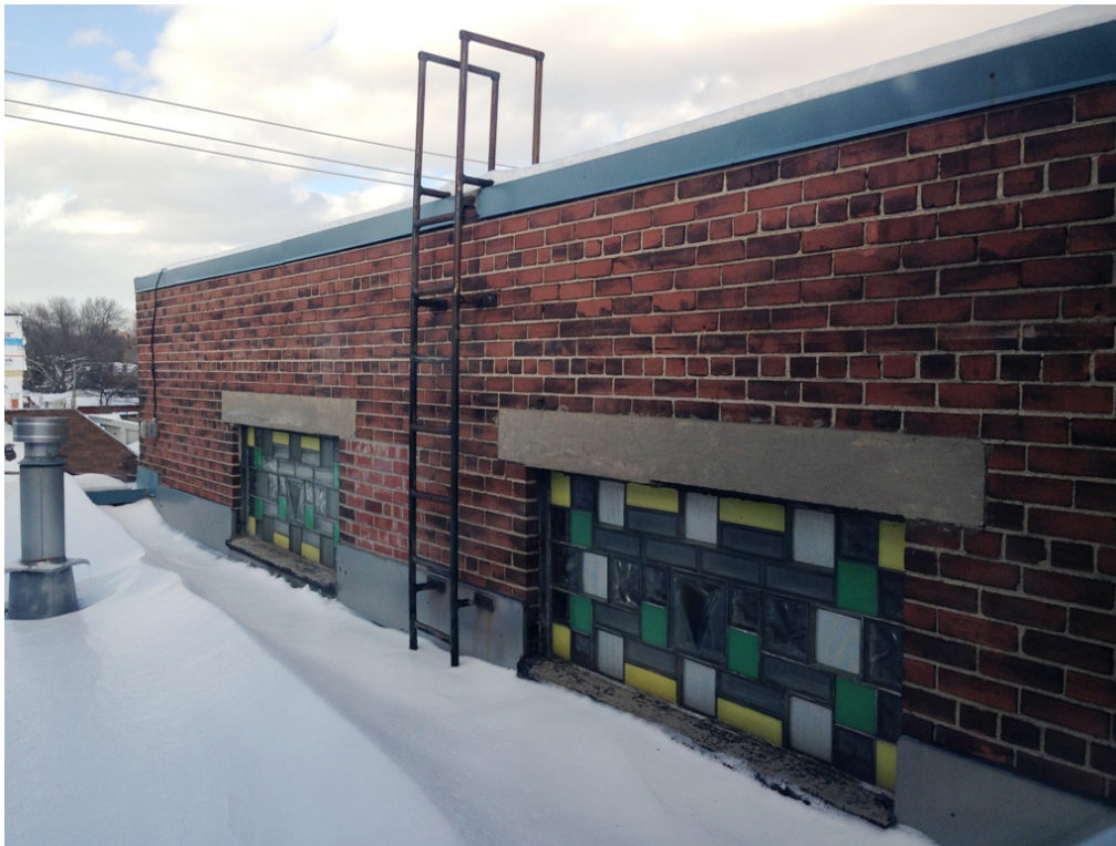
28. Exterior View of the upper side (west) elevation of Building E showing the location of the coloured glass block panels (HPS, 2018)
