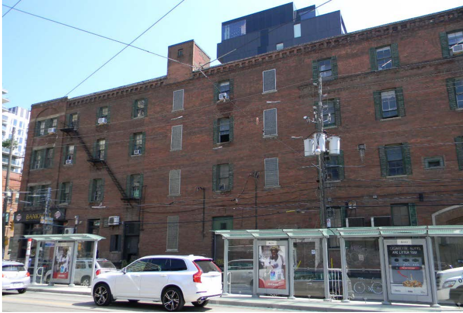
6a. West elevation on Bathurst Street, showing the north end near King Street West
