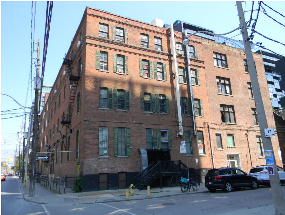
6b. South elevation on Stewart Street, with the south end of the west (Bathurst Street) elevation on the left
