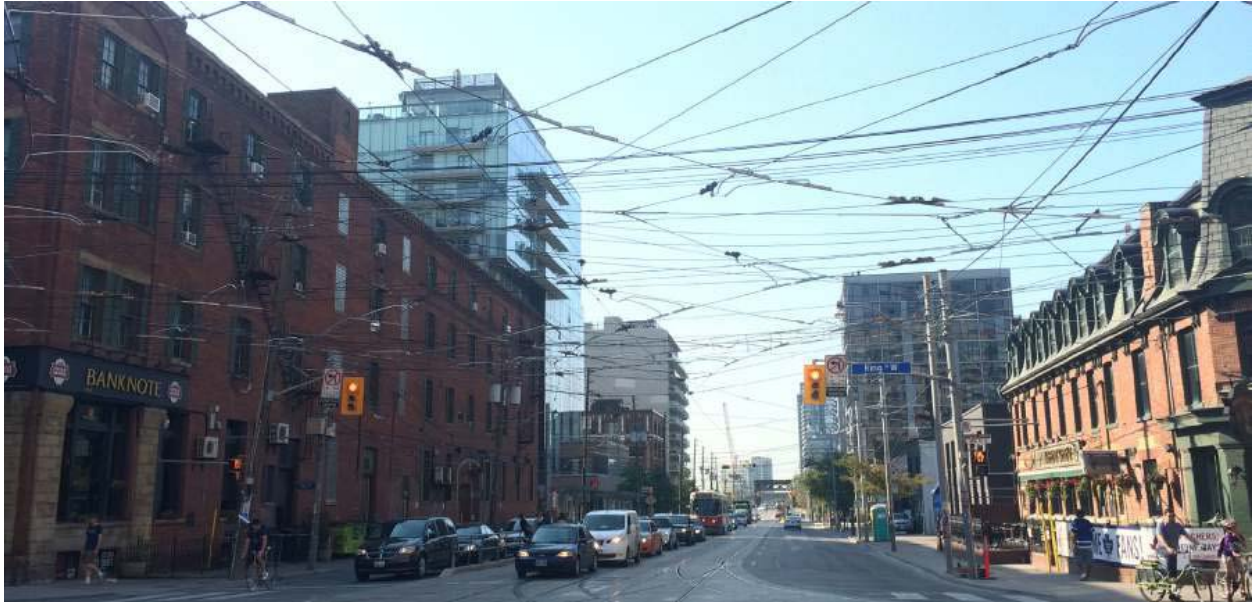
663 King Street West – Looking at the west façade along Bathurst Street
