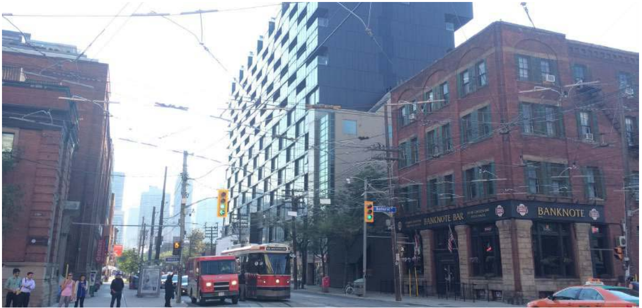
663 King Street West Looking south east towards the north façade at King Street West and the north portion of the Bathurst Street facade
