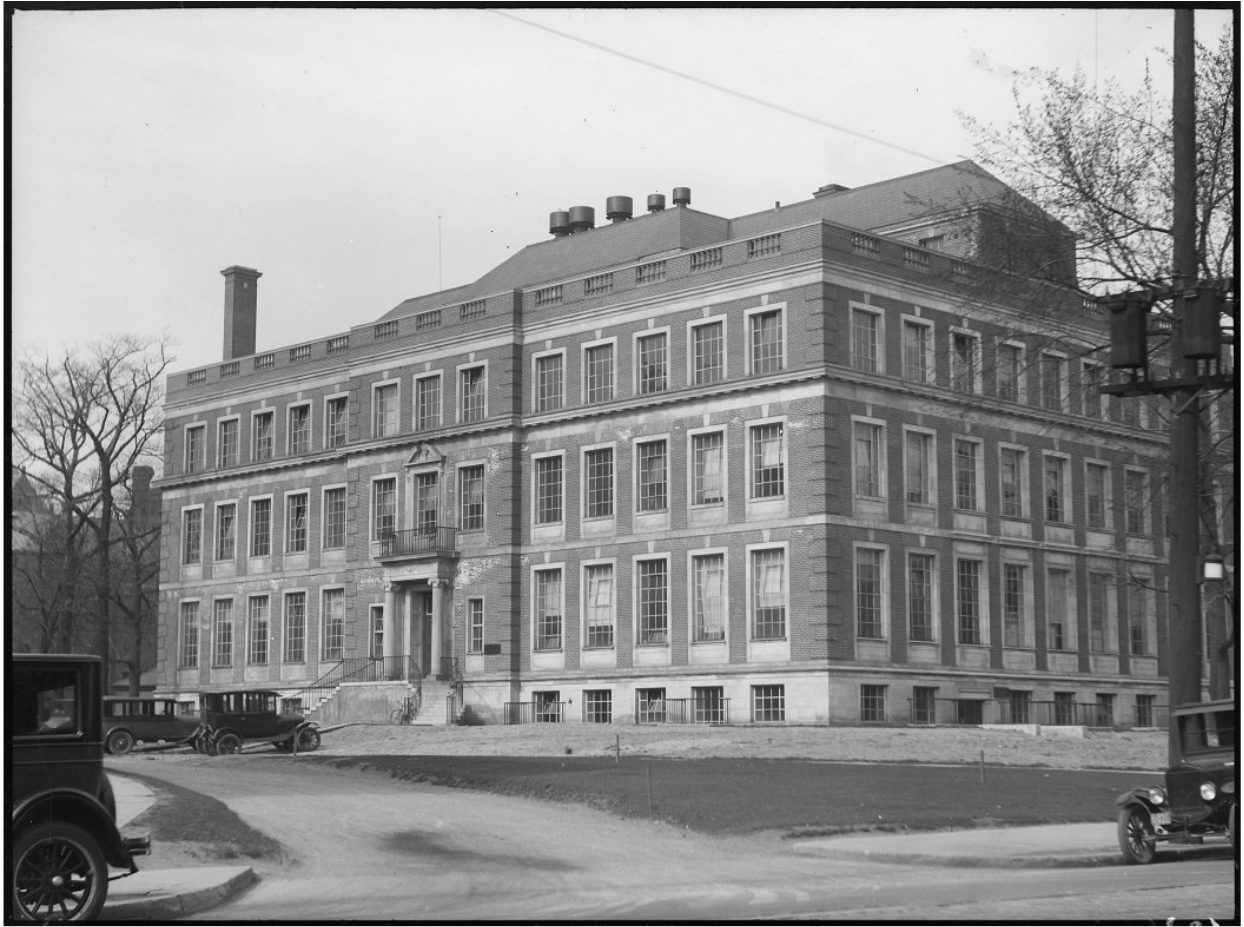
Photo shortly after construction - Note divided lite windows on both west and south facades
