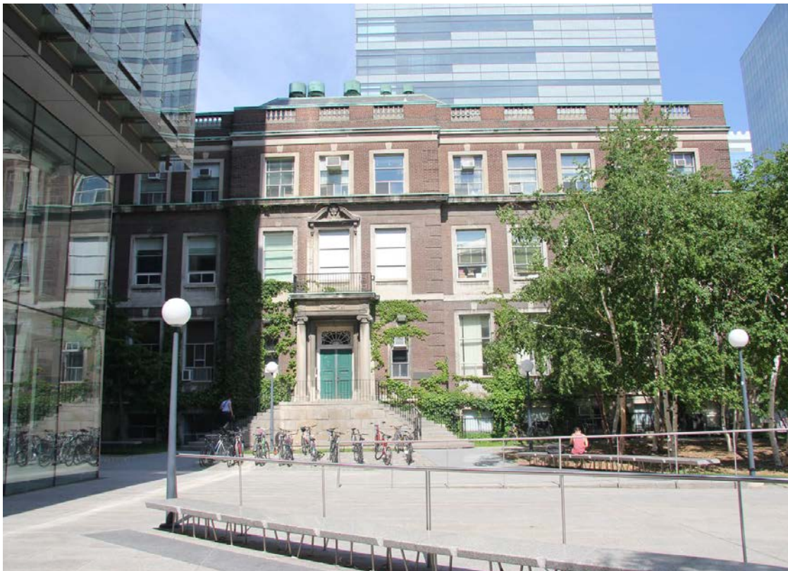
West Elevation (Primary) of 150 College Street
