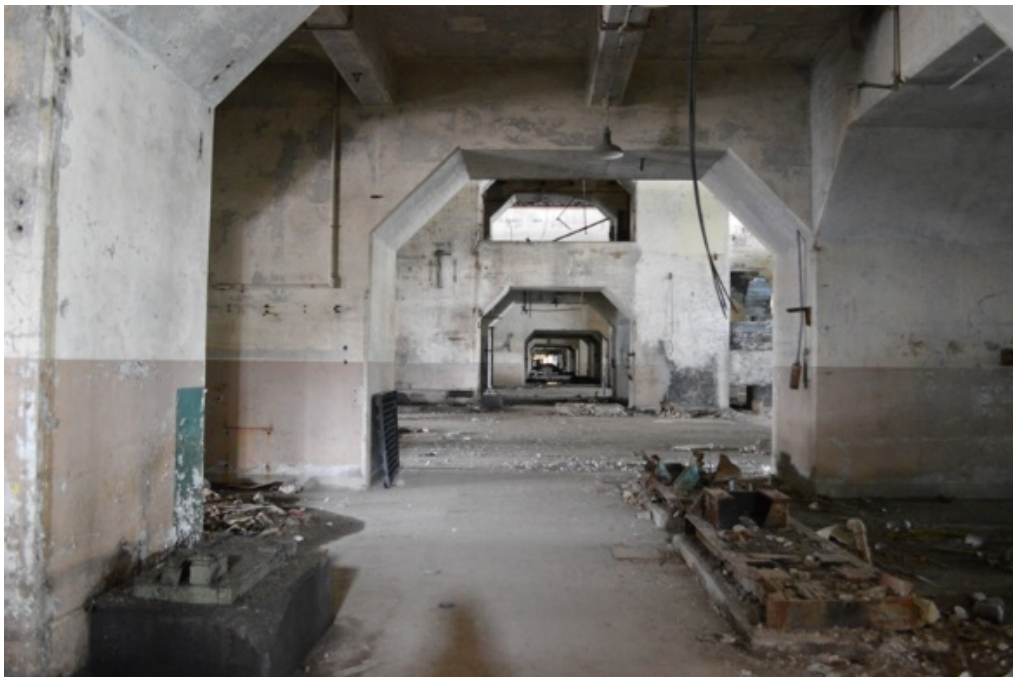
39. Interior View of the Turbine Hall looking from west to east through successive structures constructed to support 8 turbines (SIPA, 2014)
