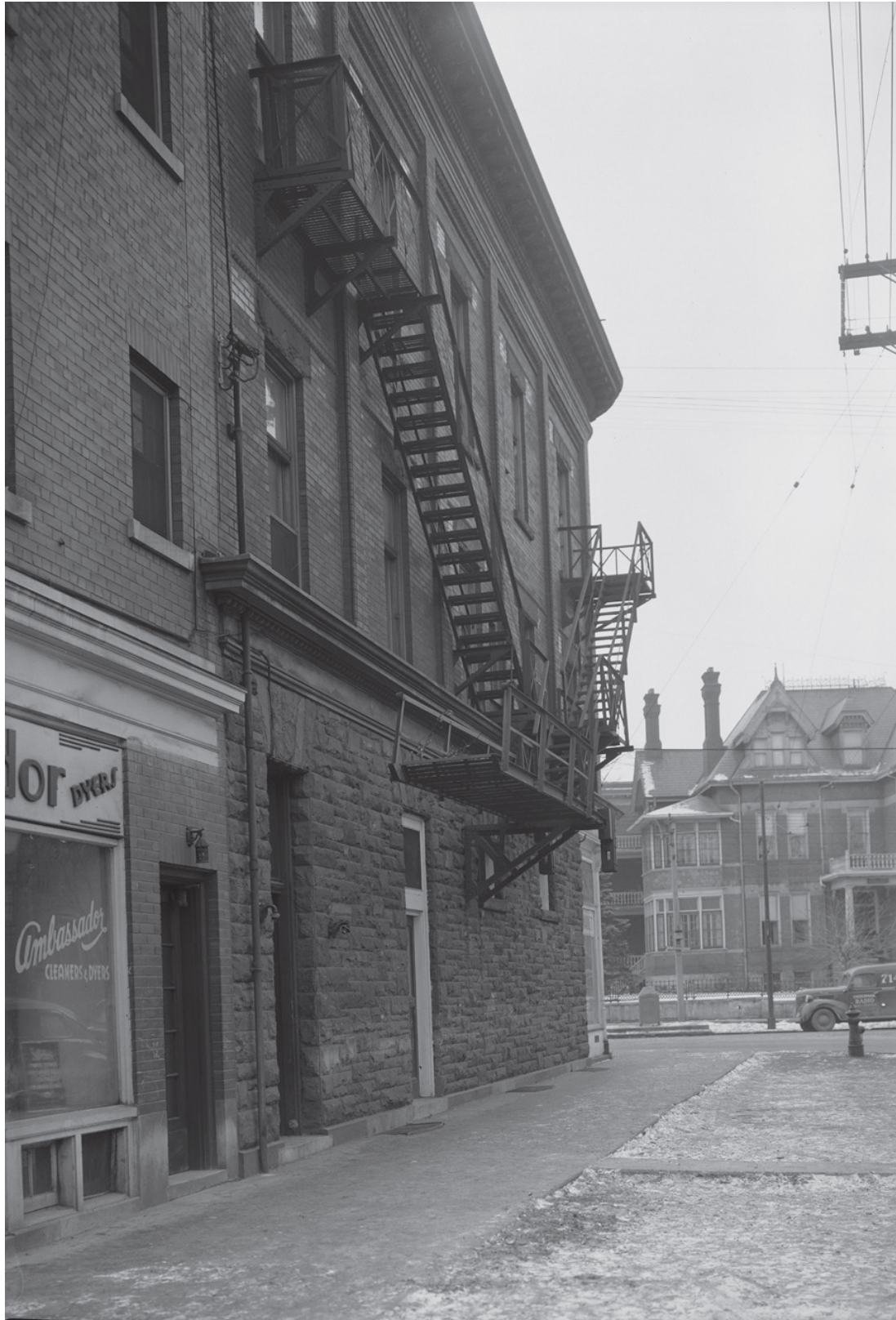
North elevation of the Thomas Cruttenden building, January 15, 1942. City of Toronto Archives, Fonds 200, Series 372, Subseries 1, Item 1600
