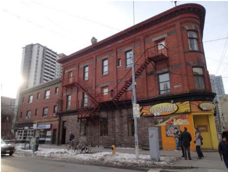
North Elevation of the Thomas Cruttenden building (ERA Architects Inc.)
