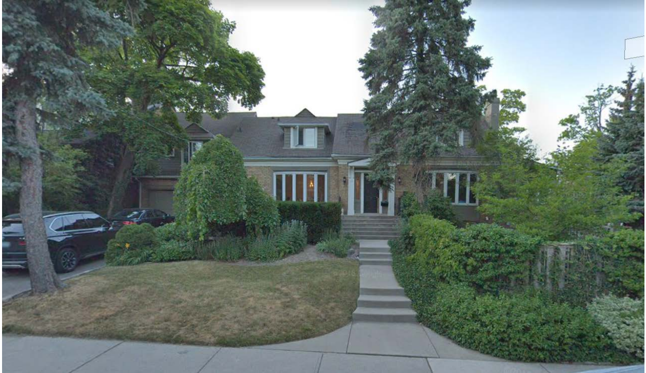
Contextual view (looking north) of the existing house to be demolished at 210 Douglas Drive
