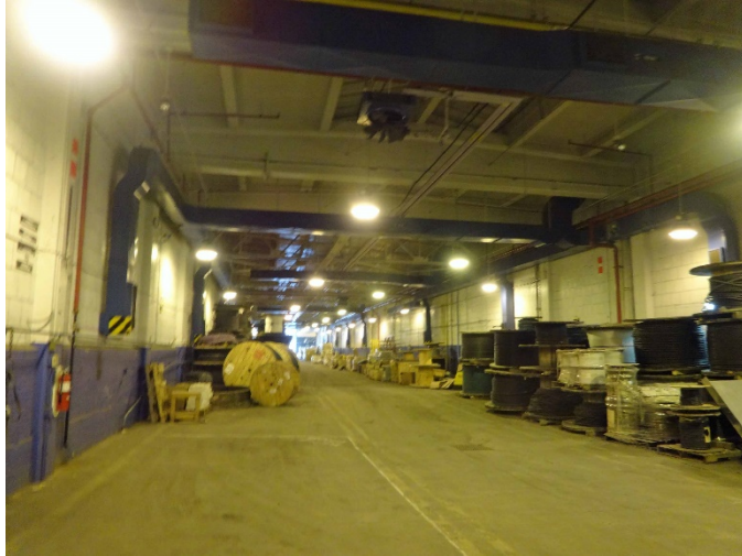
9b. interior bay with covered skylight
