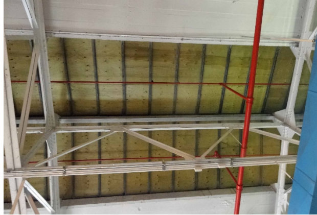
9d. covered skylight (detail)
