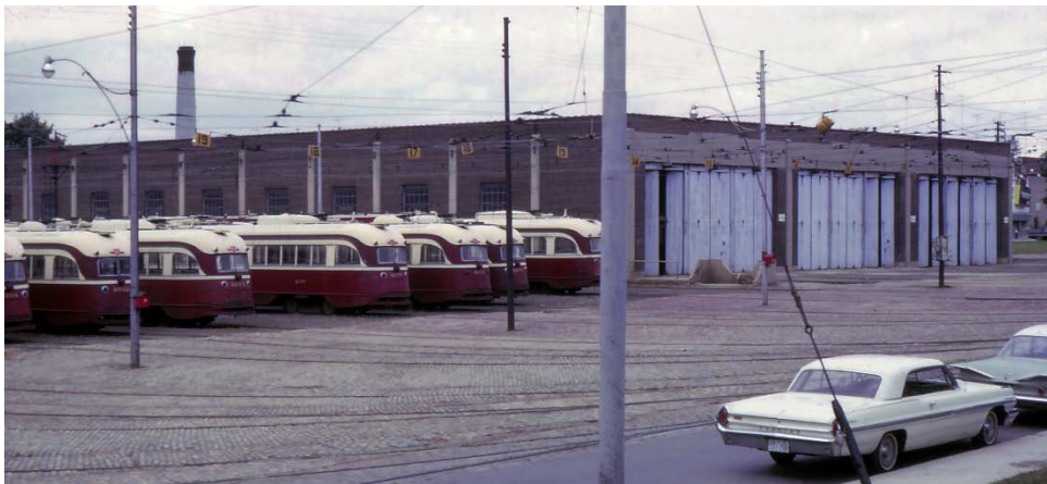
7b. 1966 view from Hillingdon Avenue with the folding wood doors on the east elevation (right)
