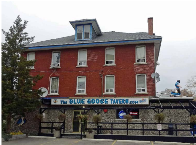
4a. west elevation on Blue Goose Street
