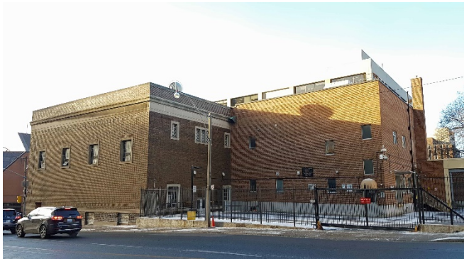
4b. East (left) and north elevations (with Eglinton Control Centre on the right)
