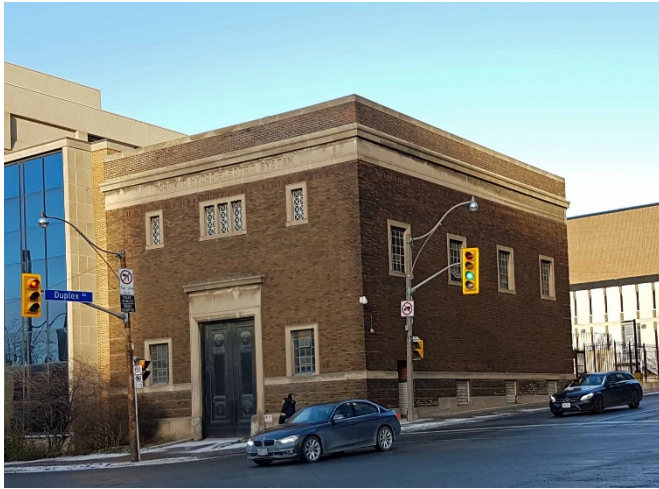
4a. Principal (left) and east side elevations
