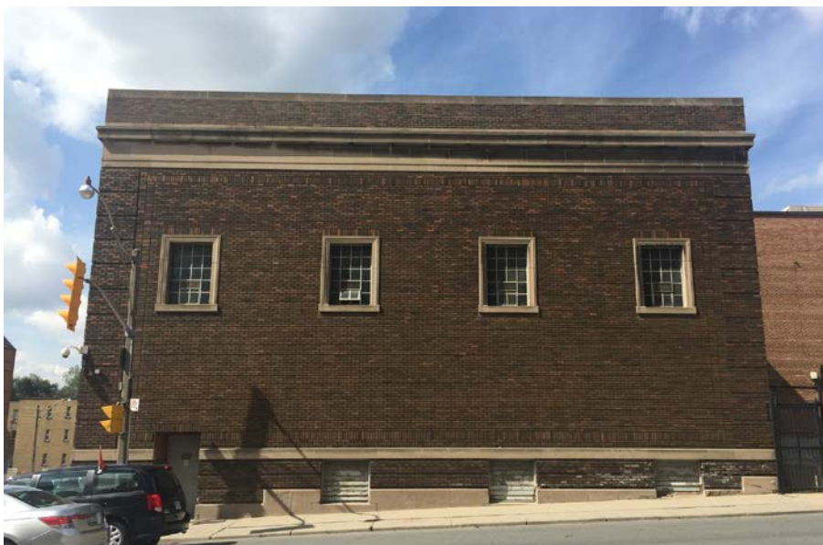
50 Eglinton Avenue West (Source: ERA Architects) East Elevation (current)
