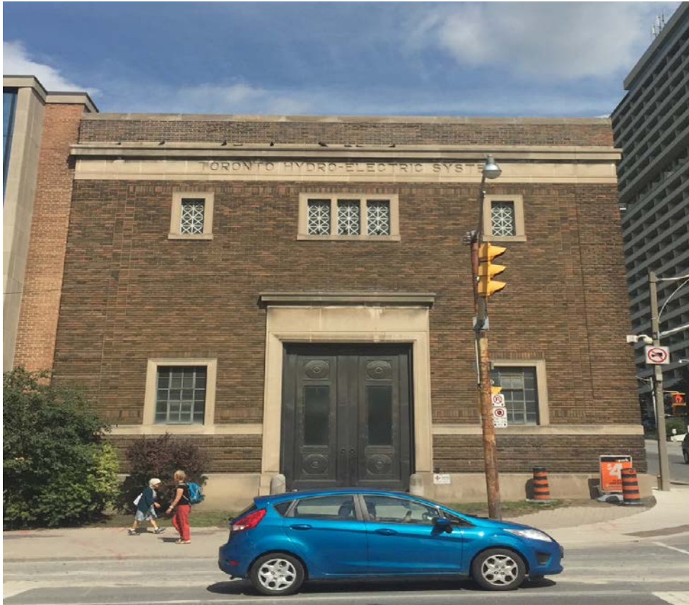
50 Eglinton Avenue West (Source: ERA Architects) - South Elevation (current)
