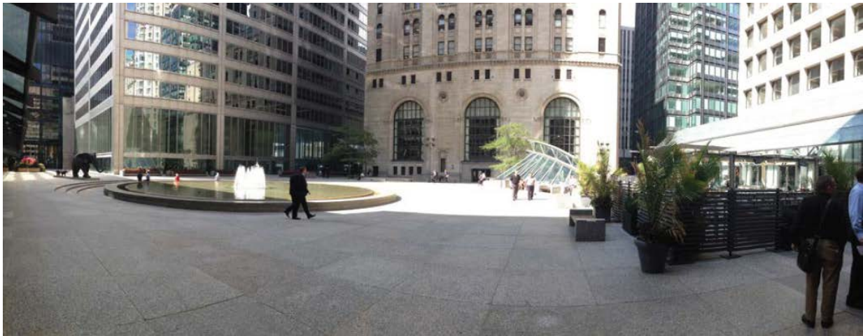
The Commerce Court North and West buildings as seen from within the courtyard (ERA Architects)
