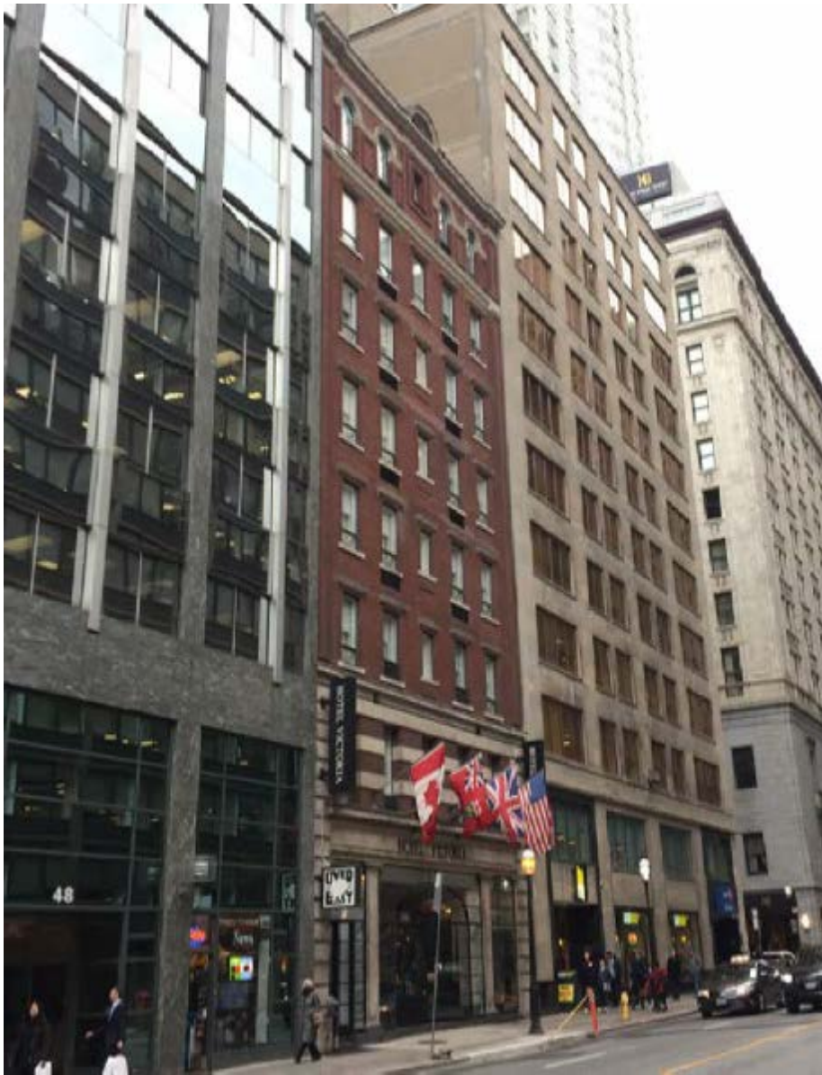
56 Yonge Street, the Hotel Mossop facing northwest (ERA Architects)
