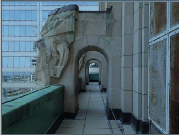
Promenade along south edge of 32 nd floor (ERA, 2017).
