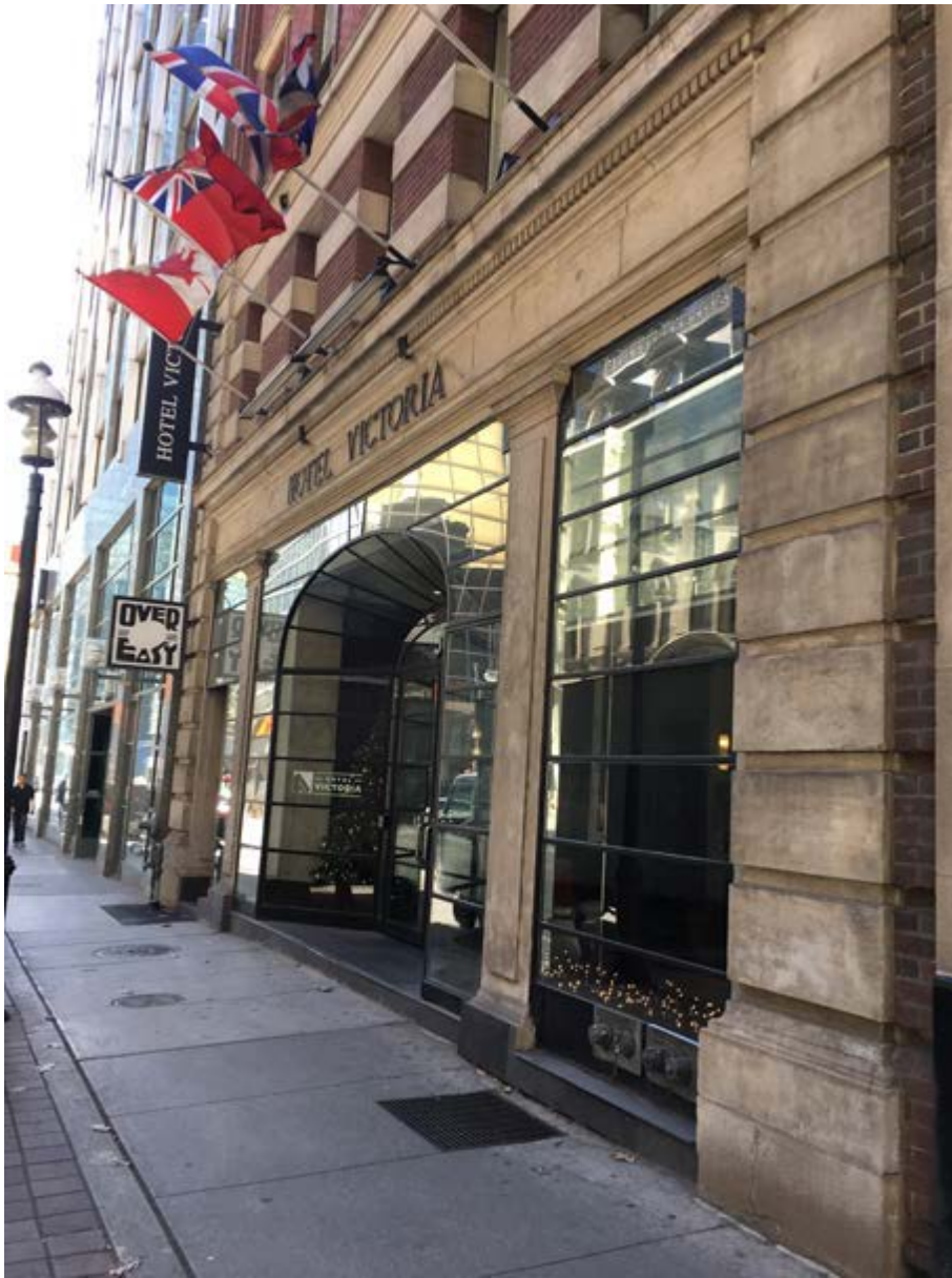
Streetfront view of the 56 Yonge Street, the Hotel Mossop facing southwest (ERA Architects)
