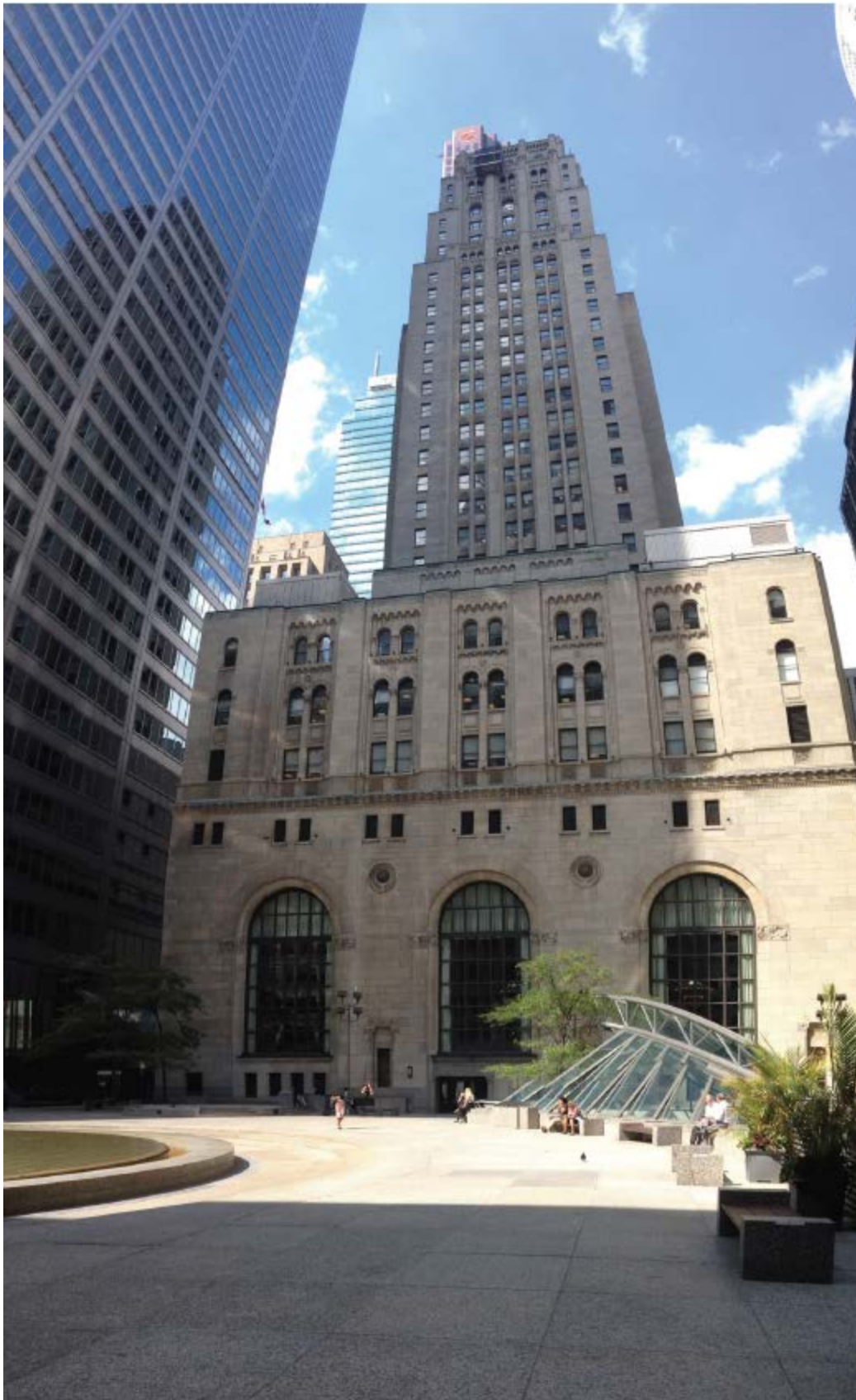
Commerce Court North looking north from within the courtyard (ERA Architects)
