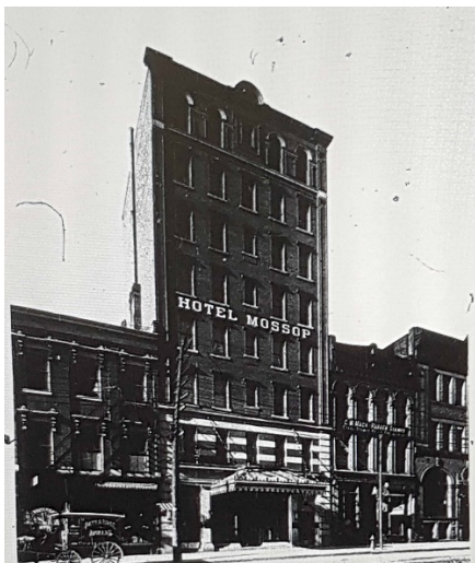
Hotel Mossop, Toronto, which, both externally and internally, is of absolute fireproof construction. It stands on a foundation of 78 concrete walls, carried down to bed-rock, the first foundation of its kind to be installed in Toronto. J. P. Hynes, Architect.
