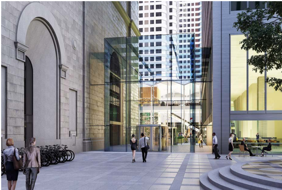
Proposed glazed link between the Commerce Court North and Commerce Court West Buildings (facing south)
