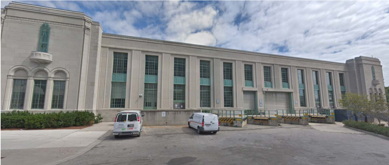
View of west façade of the Automotive Building showing the service entrances to the building and the twelve two-storey window bays. The proposed pedestrian bridge will extend from the second storey of the window bay furthest to the right.
