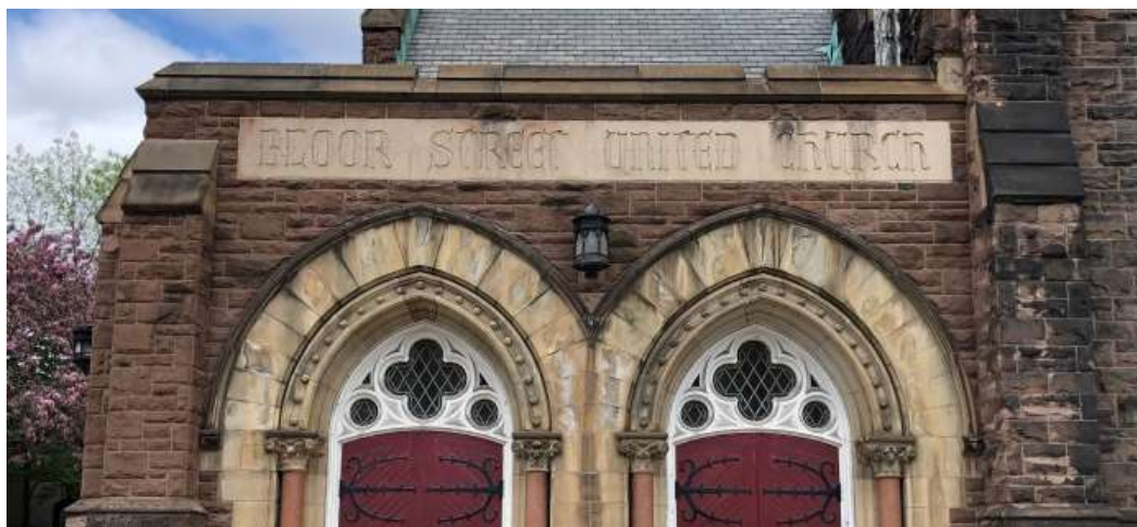
32. Entry porch with the 1956 addition of the words "Bloor Street United Church" on the stone band above the principal entry (HPS, 2019)
