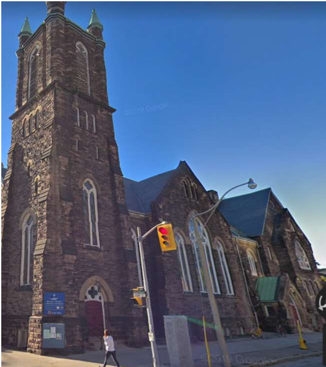
300 Bloor Street West – Huron Street/east façade
