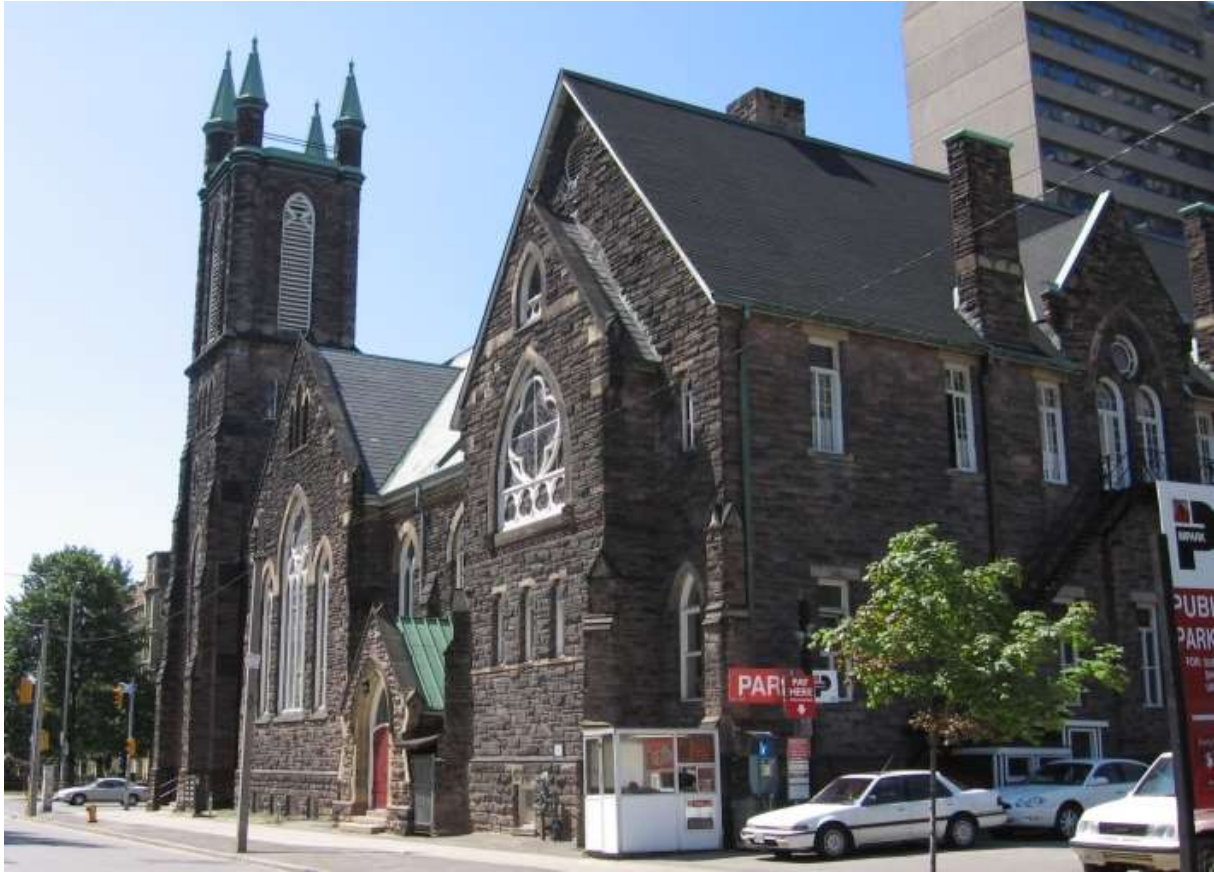
18. East elevation of the Church (left) and the original church (right) which was converted for sole use as a Sunday school following the church expansion in 1889. The new entrance added in 1927 following the widening of Bloor Street is located between the church and Sunday school (HPS, 2005)
