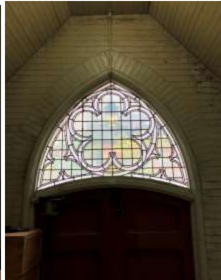
10. View of the stained glass rose window of the east elevation of the 1886-1888 building which has been partly obscured by the introduction of the attic storey above and the second floor following the church expansion in 1889-1890 (HPS, 2019)
