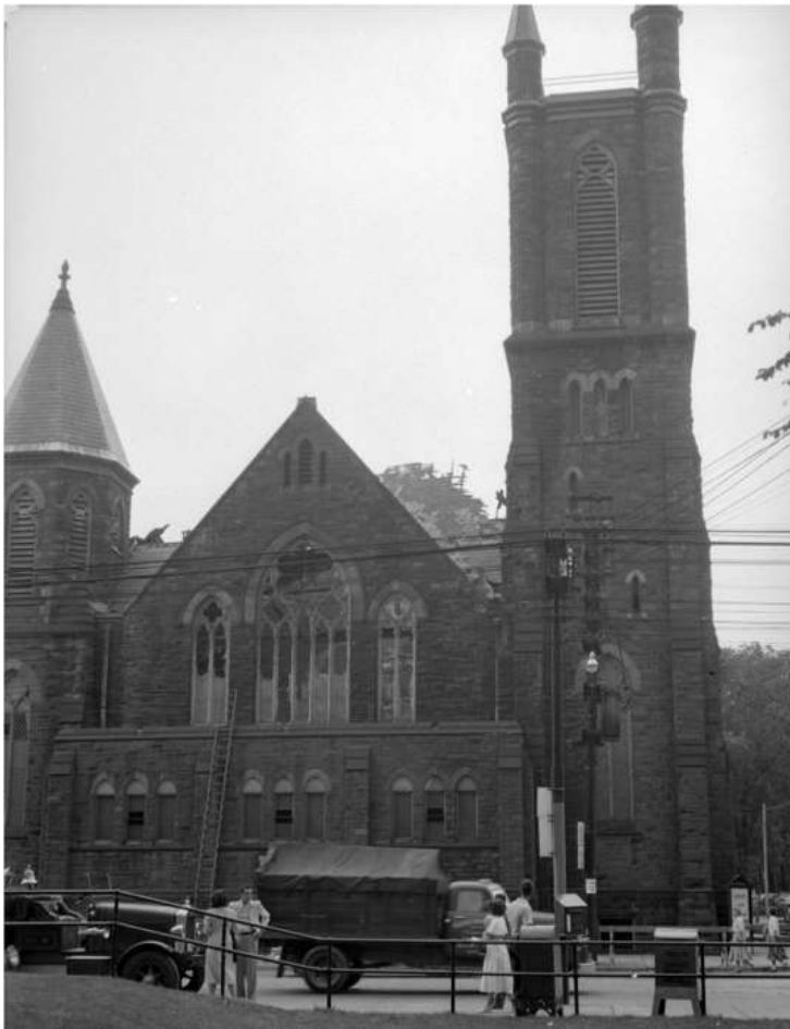
30. "Aftermath of the Fire" at Bloor Street United Church, August 1954 – the photograph shows the damage to the stained glass windows. (TPL, James Victor Salmon collection, S1-2029A)
