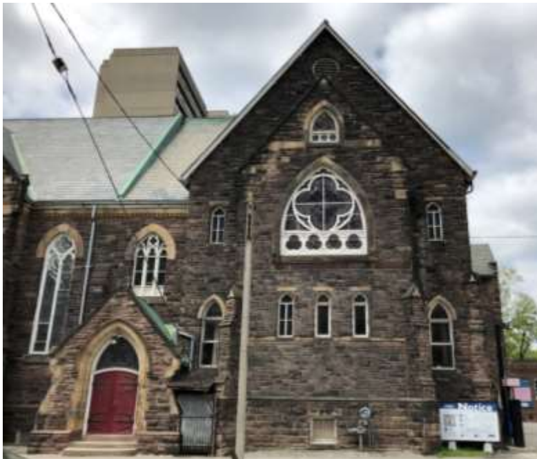
5. East Elevation of the Church and Sunday school (1886-1888) with new entry porch to the left added with the church in 1889-1890. The original 1888 roofline is indicated by the lower gable above the lancet window. The roof was raised in 1889-1890 with the addition of the new church creating a second storey and is shown in the broader, higher roof. (HPS, 2019)
