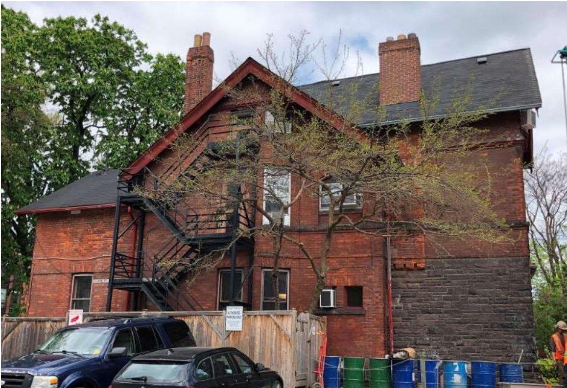
65. Side (south) elevation, 478 Huron Street (HPS, 2019)
