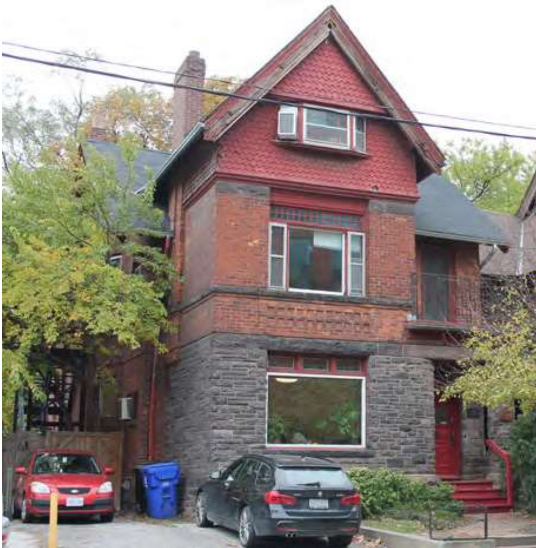
478 Huron Street, Pidgeon House – Principal (East) Elevation
