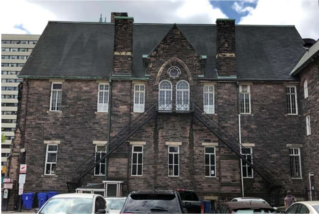
7. North Elevation of the first Church and Sunday school with the second storey addition added in 1889-1890 and the 1909 extensions to the right (HPS, 2019)
