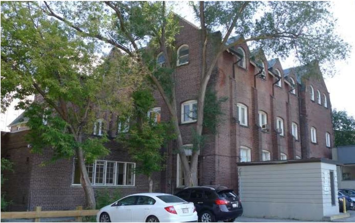
23. 1909 Sunday school extension, north and west elevations with later single storey extension for kitchen and nursery (HPS, 2015)
