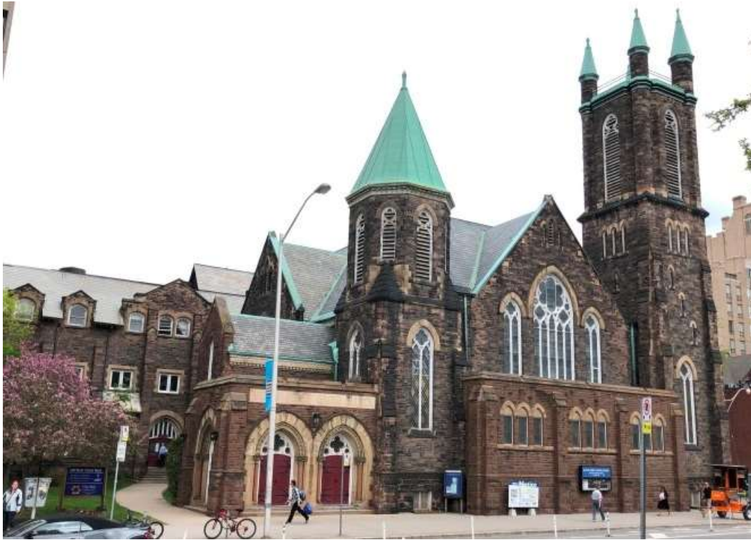
26. Photograph of the south elevation of the church facing Bloor Street West, showing the 1927 changes to the church elevation when Bloor Street was widened and the stairs were removed. The narthex with the three sets of three arched windows was extended moderately and the three original stone archways with their red stone columns were relocated to a single storey entry at the left. The landscaped courtyard and 1909 Sunday school can be seen at the far left and rear of the photograph. (HPS, 2019)
