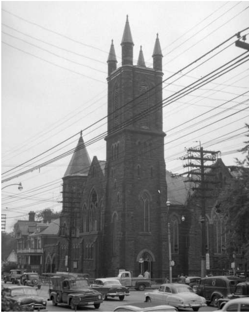
31. "Aftermath of the Fire" at Bloor Street United Church, August 1954 – the photograph shows the damage to the roof and the stained glass windows. The photo also shows the removal of the steps on Bloor Street and the replacement of the three arched openings with the row of 9 arched windows following the widening of Bloor Street in 1927. The arches can be seen in the single storey pavilion which was relocated to the west. (TPL, James Victor Salmon collection, S1-2029B)
