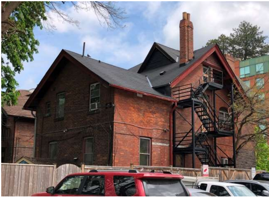
66. Rear (west) and side (south) elevations, 478 Huron Street (HPS, 2019)
