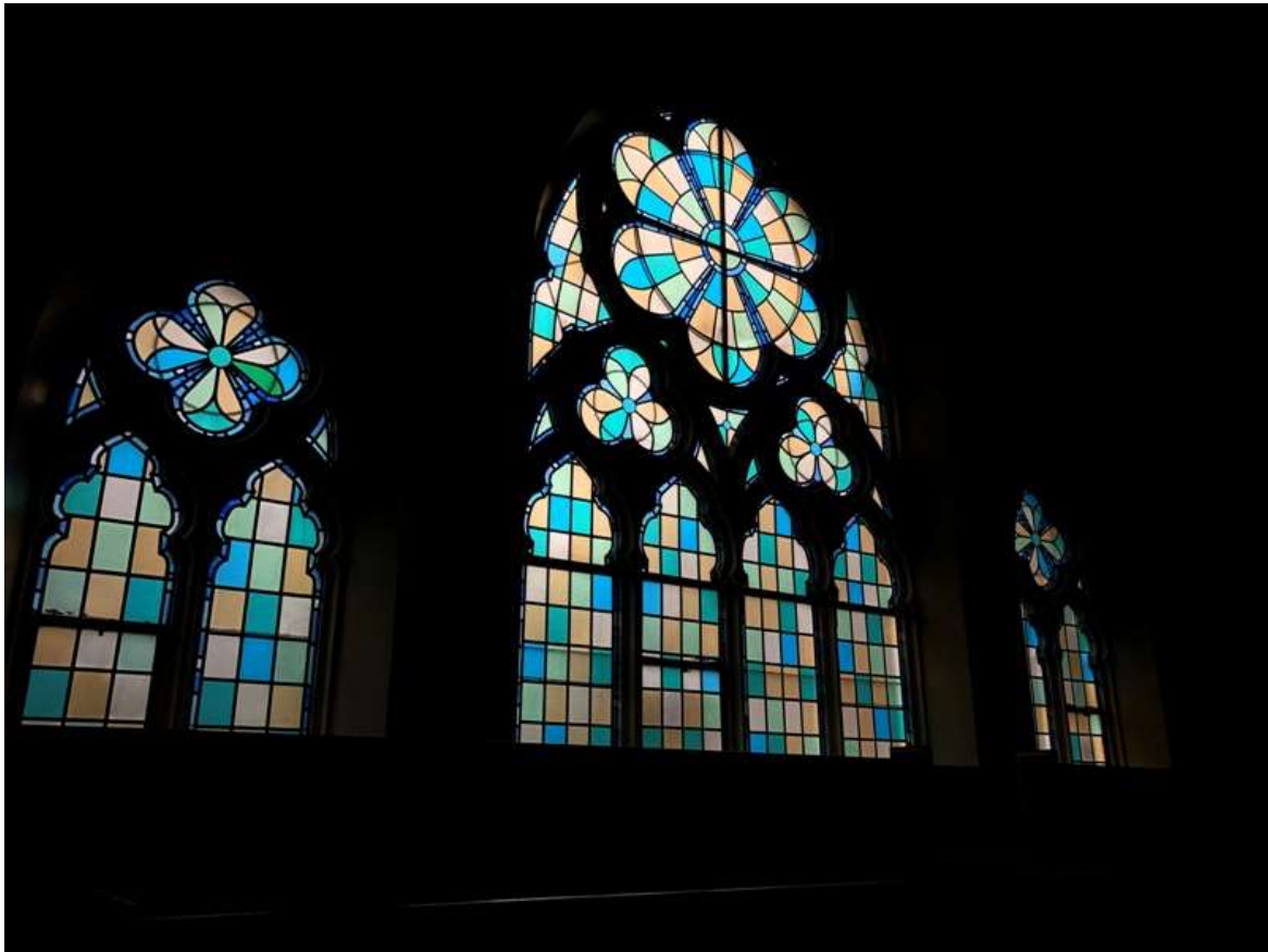
44. View of the three west windows, repaired following the 1954 fire (HPS, 2019)
