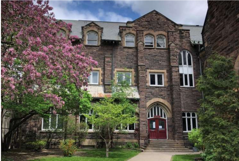
20. 1909 Sunday school extension, south elevation facing the landscaped courtyard and Bloor Street (HPS, 2019)
