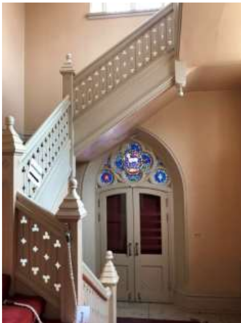
55. East Tower stairs showing original 1889-1890 handrails (HPS, 2019)
