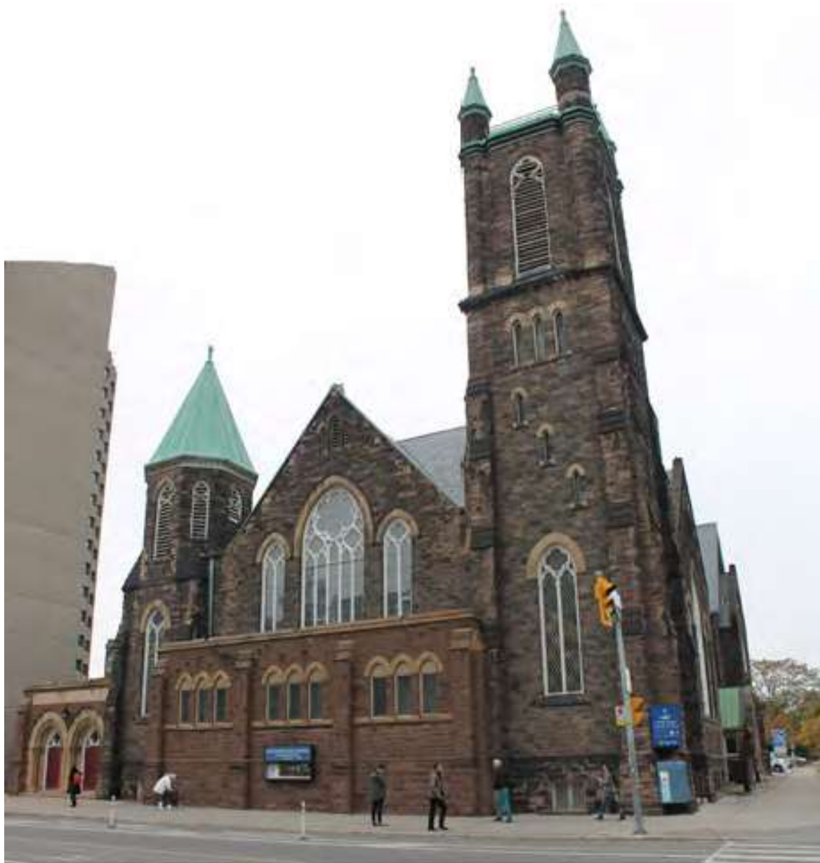
300 Bloor Street West – Looking towards the Bloor Street West/south façade
