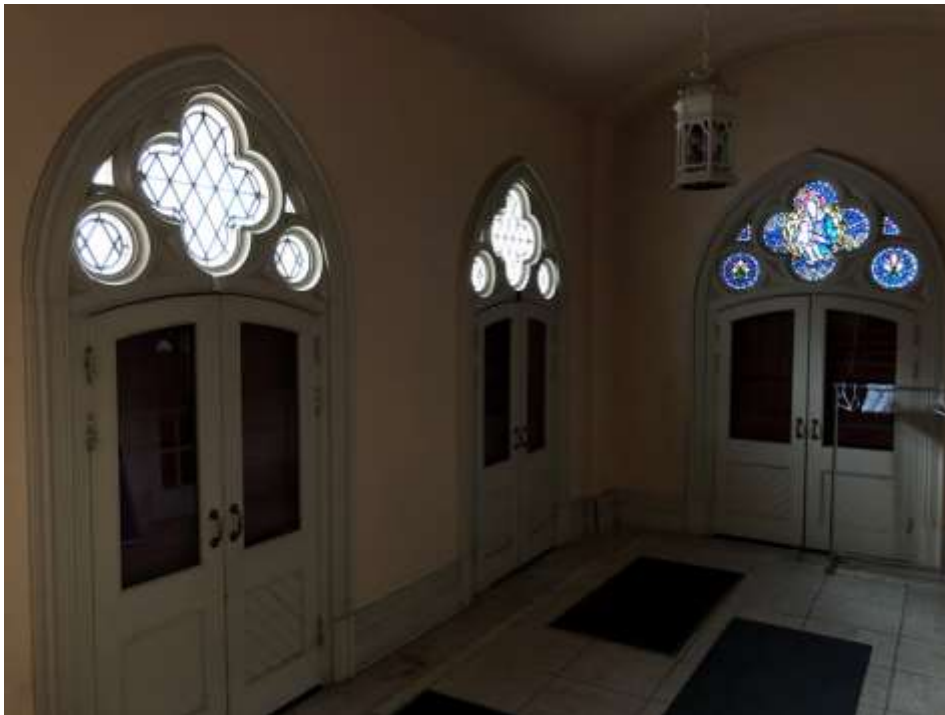
57. Interior of the West Entry porch with the relocated archways with their stained glass leaded and stained glass transoms (HPS, 2019)
