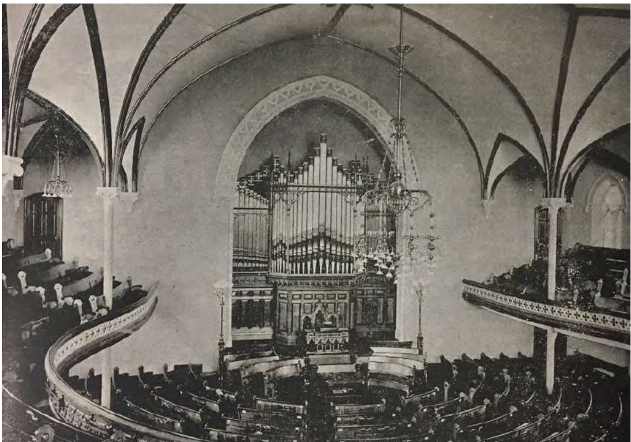
39. View of the interior facing north towards the organ and pulpit showing the auditorium style of the church hall with the u-shaped upper gallery, 1891 (Dominion Illustrated)
