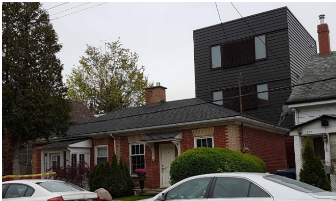
Current Photographs, 719-721 Richmond Street West, 2019 (Heritage Preservation Services)
