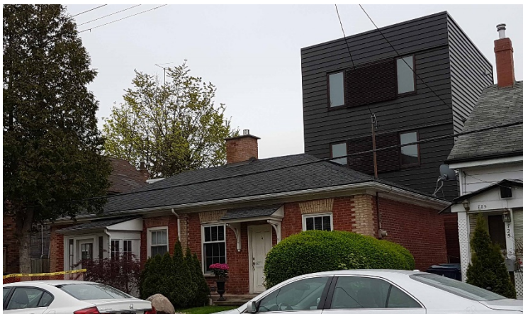
8e. 719 (left) and 721 Richmond Street West, 2019: showing the properties following restoration, with the rear (south) addition on 721 Richmond (right)
