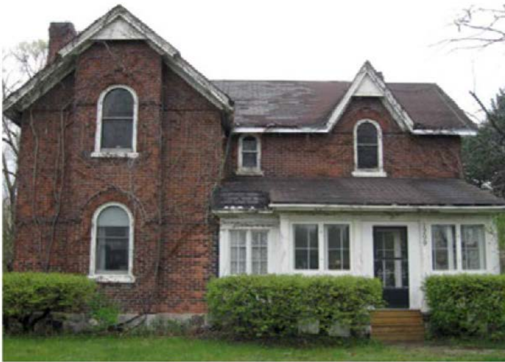
View (facing east) of the existing property's primary west elevation, including the one-storey sunroom.
