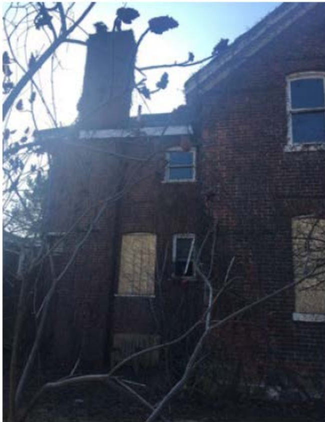
Partial view of the property's northern elevation.
