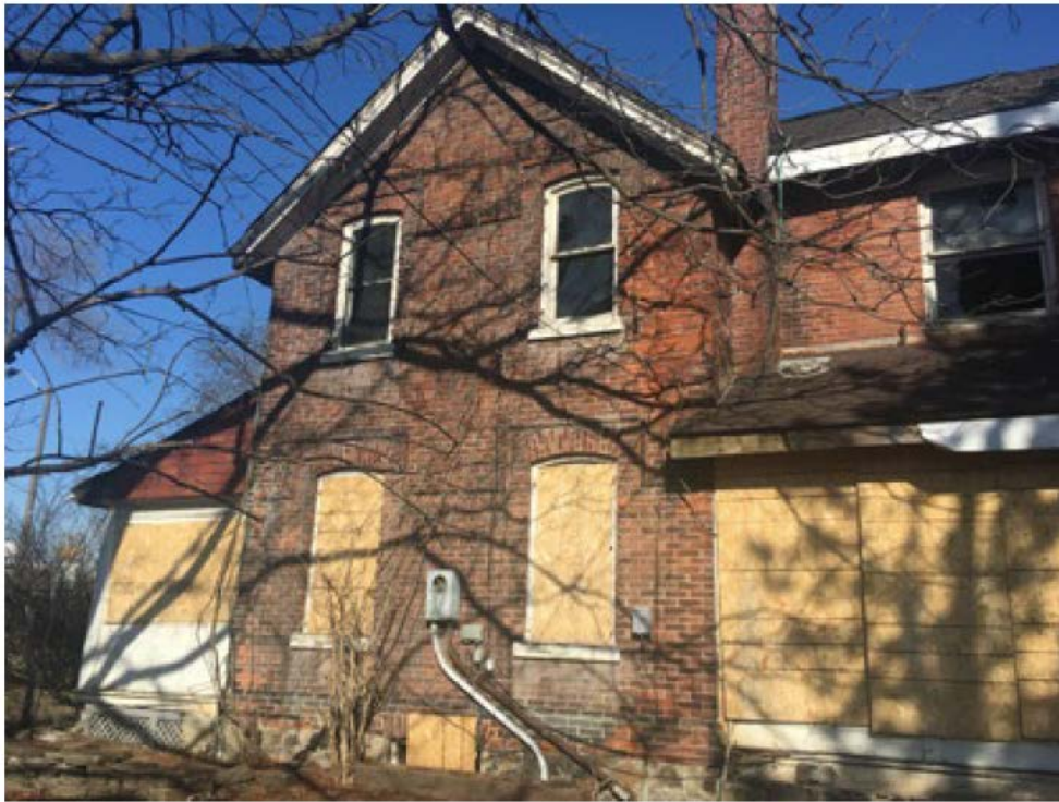
View (facing north) of the south elevation of the existing property.
