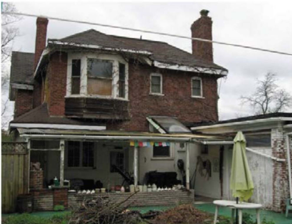
View (facing west) of the east elevation of the existing property.
