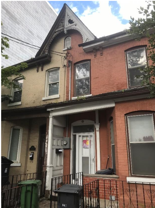
8a and b. Photographs showing the principal (west) elevations at 143(b) and 145(a) Portland Street, including the decorative wood bargeboards in the central, share cross-gable: Heritage Planning, 2019.
