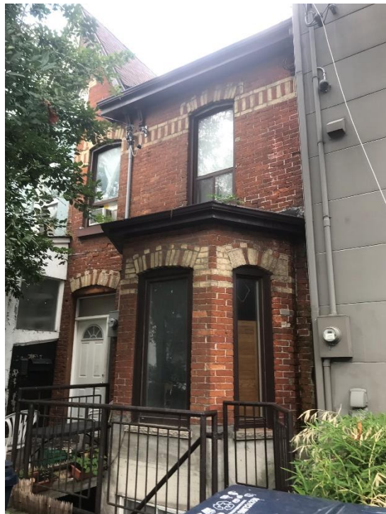
8c and d. Photographs showing the principal (west) elevations at 139(d) and 141(c) Portland Street, including the original polychromatic brickwork at 139 (the same brickwork at 141, 143 and 145 is currently covered with paint): Heritage Planning, 2019.
