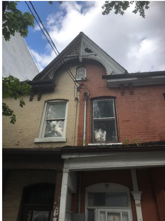
8a and b. Photographs showing the principal (west) elevations at 143(b) and 145(a) Portland Street, including the decorative wood bargeboards in the central, share cross-gable: Heritage Planning, 2019.
