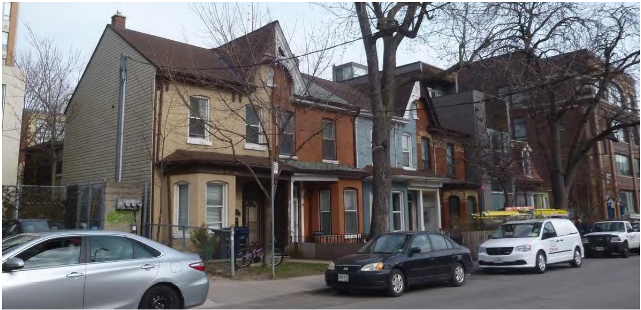
4. Photograph looking southeast and showing 145 Portland Street, at left, which forms the north anchor of the surviving two pairs of historic row houses built together in 1881: ERA, 2016.
