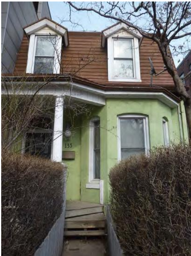
5. Photograph of the Second Empire style dwelling at 135 Portland Street with the prototypical Mansard roof (currently clad with siding): ERA, 2016.
