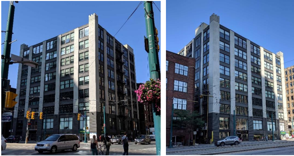
7a. and 7b. 96 Spadina Avenue: east and north elevations facing Spadina and Adelaide (left) and east elevation on Spadina (right)
