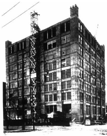
4b. Darling Building, Construction magazine, 1908
