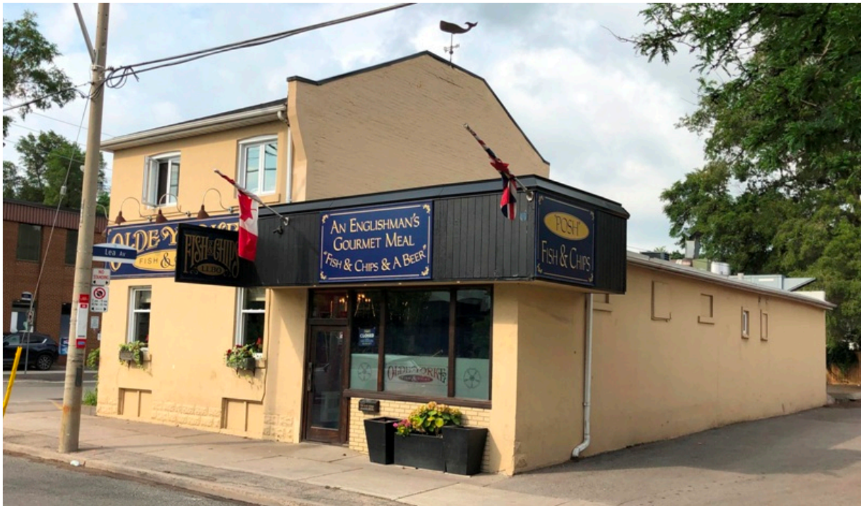
96 Laird Drive, east and north (side) elevations showing the original Osmond's Restaurant (left) with the extension to the north on Laird (HPS, 2019)
