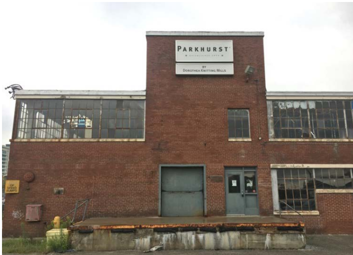
20 Research Road, west elevation (north end) showing the asymmetrical composition of the elevator tower and its 'punctured' window in contrast to the ribbon windows which wrap around the rest of the building (HPS, 2018)
