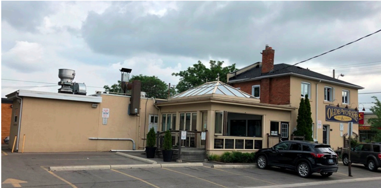
96 Laird Drive, south and west elevations showing the original Osmond's Restaurant (right) with the extension to the west with the hipped roof skylight and the c1942 north extension behind (HPS, 2019)
