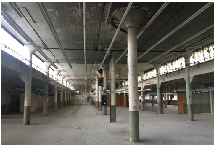
20 Research Road, Interior View of the Second Floor showing the concrete structure with the mushroom columns and the glazed roof monitor (left) and detail of the factory sash glazing (right) (HPS, 2018)
