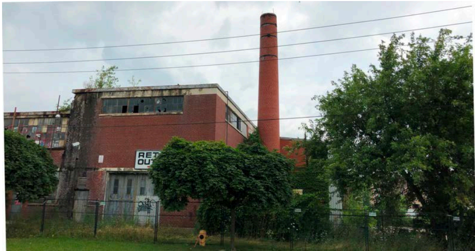
South and east elevations with the raised east end and later additions behind chimney (HPS 2019)
