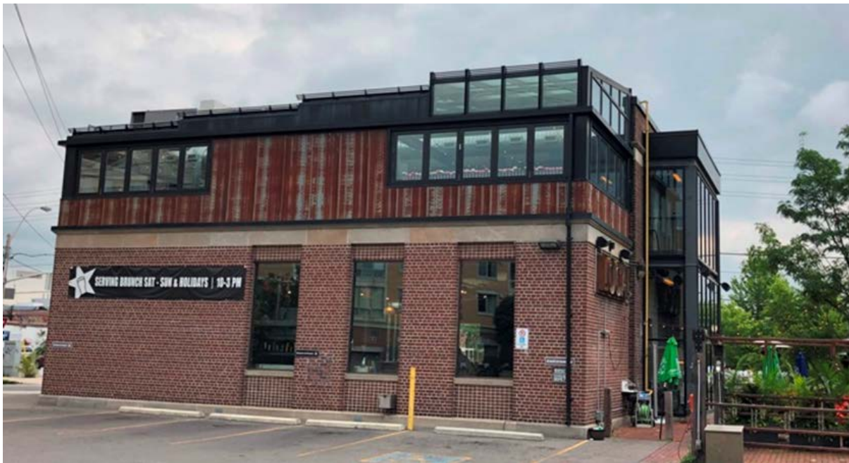
Rear (west) and side (south) elevations showing the 1961, first floor extension of the bank which matched the original materials and details and the 2013 extensions at the second floor and the glazed stair case on the south elevation (HPS, 2019)
