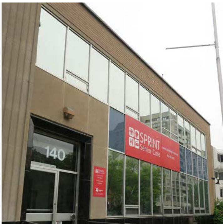
Front Façade close-up
