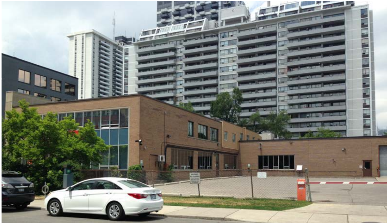
140 Merton Street: photograph showing the east side of the property as it faces the street. Note at the rear of the original building, the second-storey addition constructed in 1985 indicated by the different coloured brick, as well as the single-storey addition, at the rear of the parking lot completed in 1973. (HPS, 2016)
