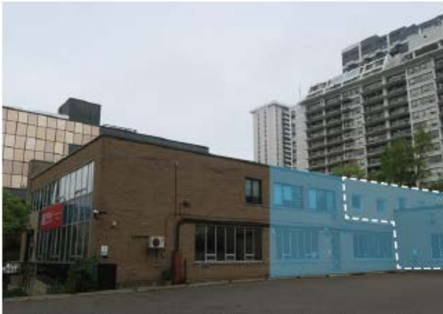
East elevation, with area of removal in blue, excluded additions in white dashed line (ERA, 2019).
