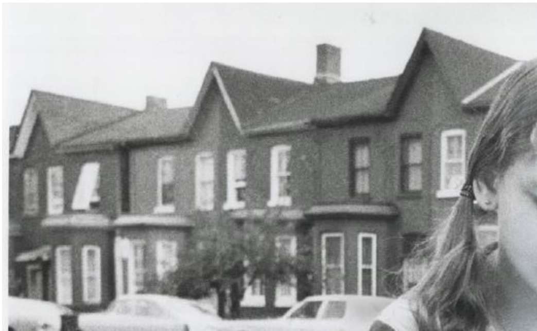
11. Archival photo from 1973 showing 65-73 Niagara Street with, likely original, double-hung sash windows on the main and upper storeys, as well as 65-69 being covered with paint, which has since been removed to reveal and display the original, decorative red and buff brickwork typical of Late Gothic Revival styling (City of Toronto Archives)
