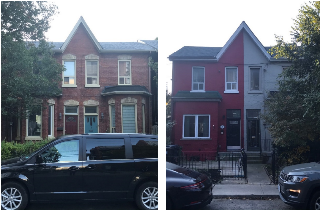
12a and b. (Left) 63-65 Niagara Street, showing the original polychromatic brickwork on the principal (north) elevation and the hexagonal single-storey bay windows flanking the side-by-side entrances under the central cross gable. This paired and mirrored organization and massing is evident in all ten of William H. Essery's properties at 55-73 Niagara Street. (Right) William L. Essery's five properties display the same organization and massing, the only difference being the shape of the single-storey bay, which is rectangular in shape and only contains window openings in the north side of the bay. (Heritage Planning, 2019)
