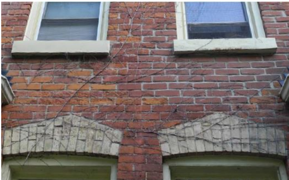
13. Current photograph showing the polychromatic brickwork with its buff brick detailing and unusual headers comprised of a segmental arch that terminates in a point at the keystone. (Common Bond Collective, 2018)
