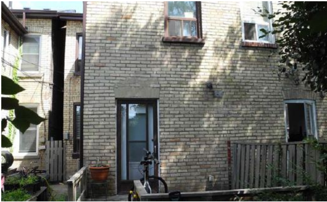
14. Current photograph showing the buff brick rear (south) elevation at 65 Niagara Street. (Common Bond Collective, 2018)
