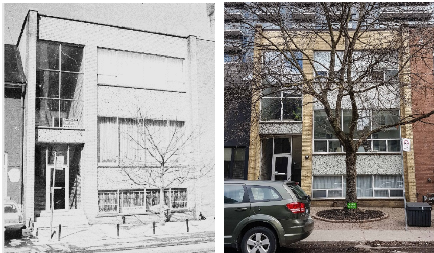
6b. 12 Camden Street: 1973 (left) and 2019 (right)
