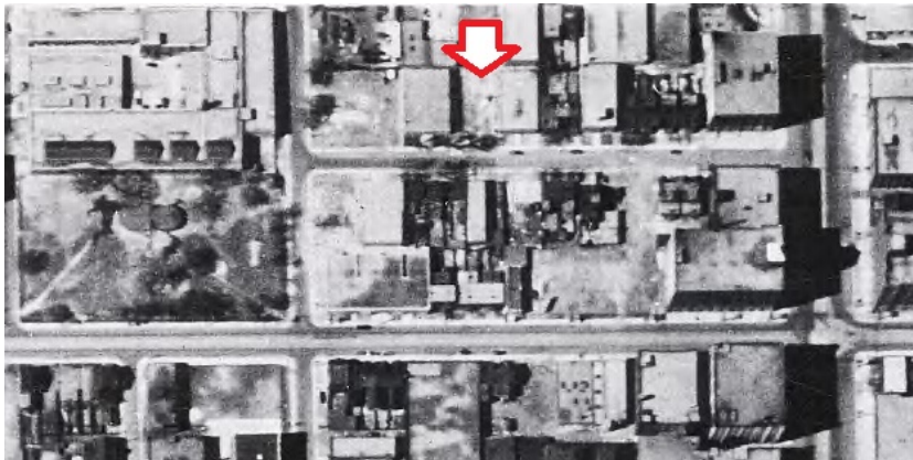
3b. Aerial Photograph, 1950: showing the vacant subject property
