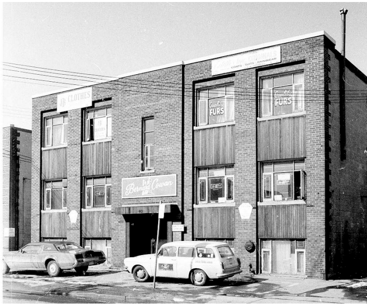
4a. 38 Camden Street, 1973
