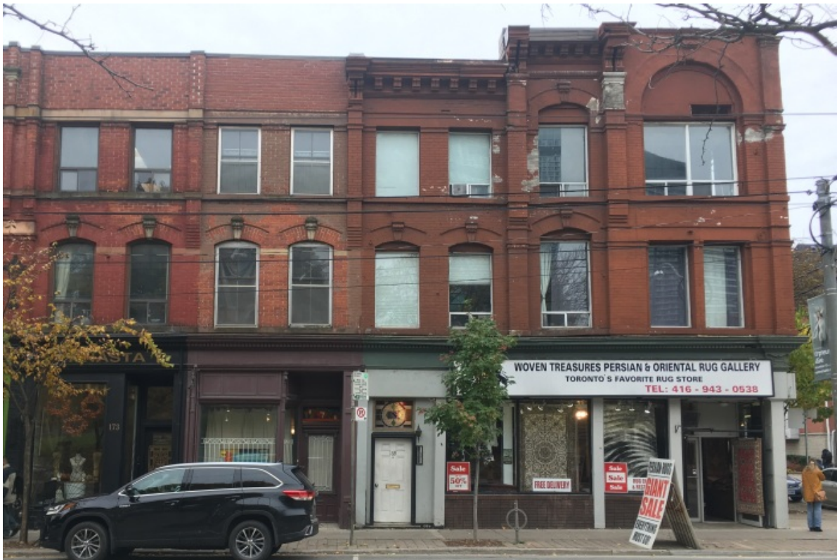
16. Photograph of the properties at 167 (169), 171 and 173 Queen Street East, principal (north) elevations (HP, 2019)
