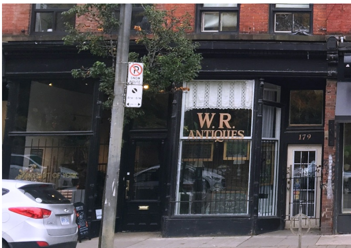
21. 179-181 Queen Street East, shopfronts showing the original pattern of the recessed entrances with the bay window, its decorative colonettes and the cornice and entablature above. (HP, 2019)
