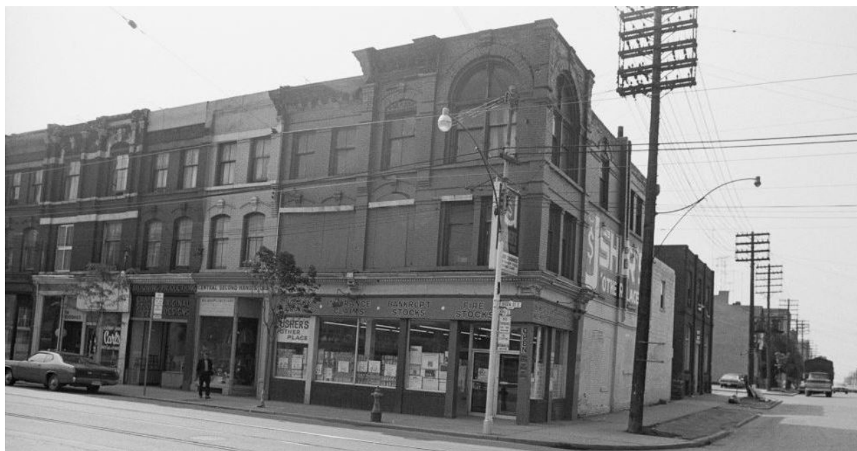
Above: Thomas J. Wilkie Block at 167-185 Queen Street East, principal (south) and side (west) elevations (City of Toronto Archives, [CTA] Fonds 2032, Series 841, File 271, Item 29) Cover: 167-185 Queen Street East (Heritage Planning [HP] 2019)
