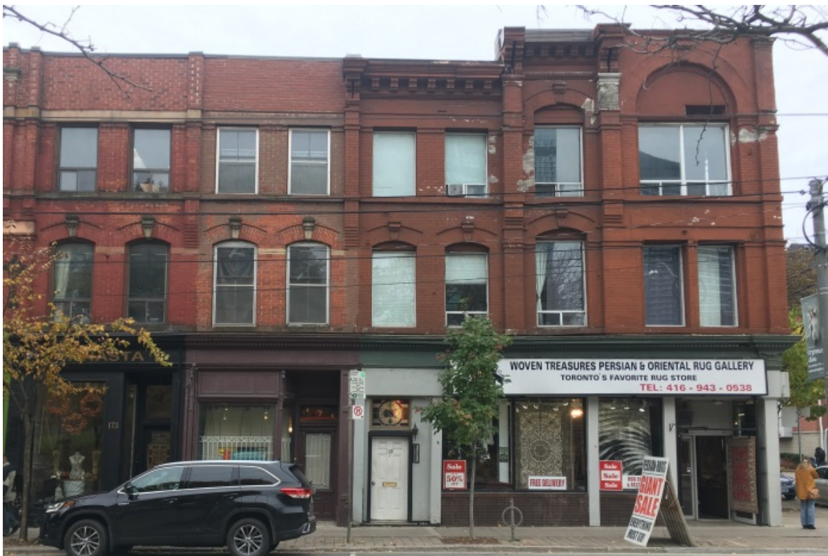
Photograph of the properties at 167 (169), 171 and 173 Queen Street East, principal (north) elevations (HP, 2019)
