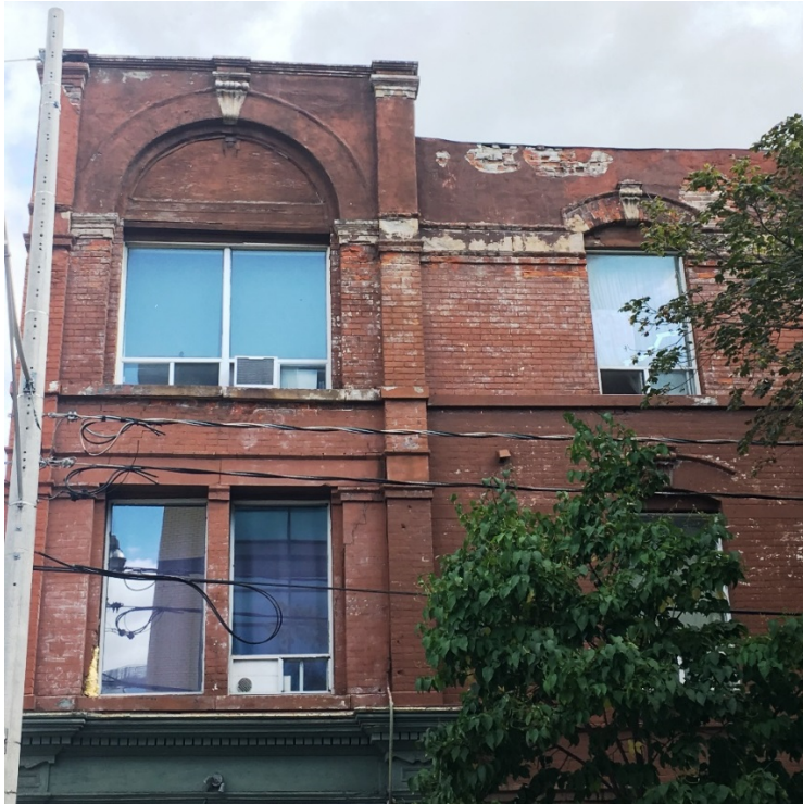
24. 167 Queen Street East, side (west) elevation details facing George Street (HP, 2019)
