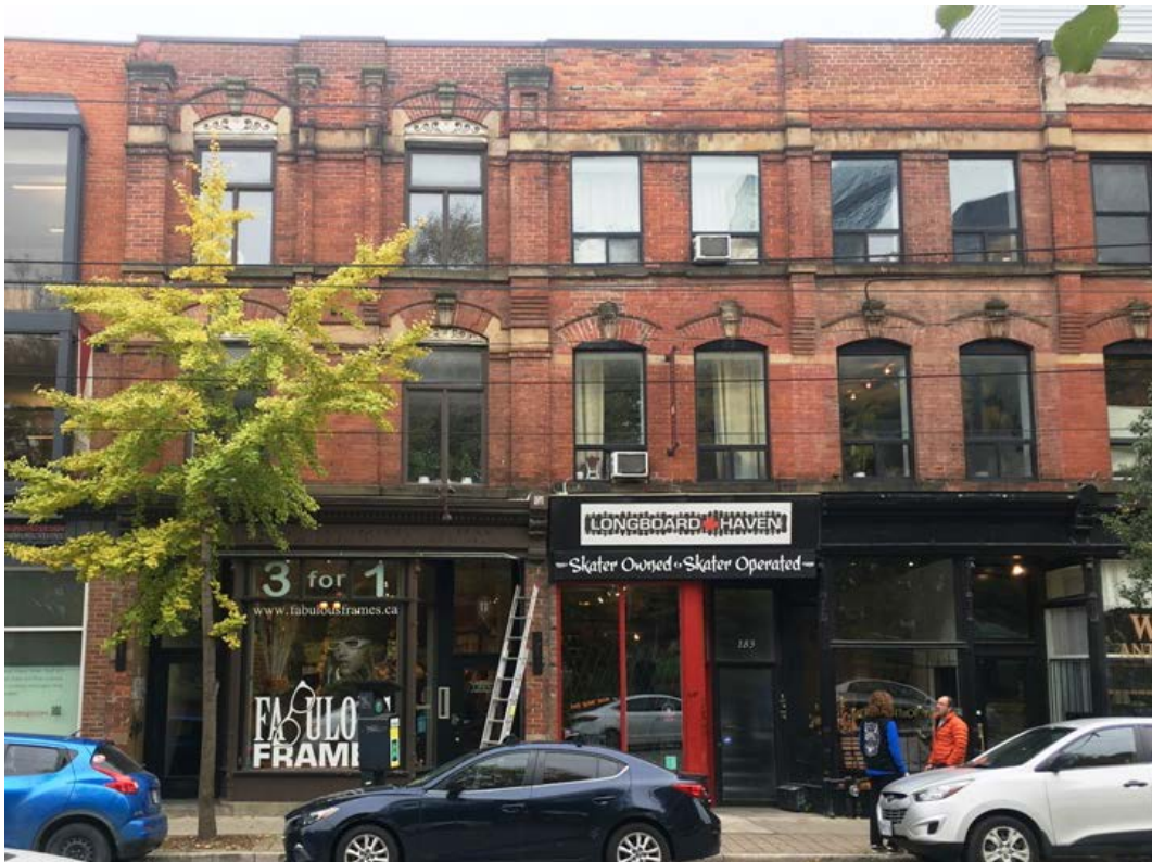
Photograph of the properties at 181-185 Queen Street East showing the principal (north) elevations (HP, 2019)
