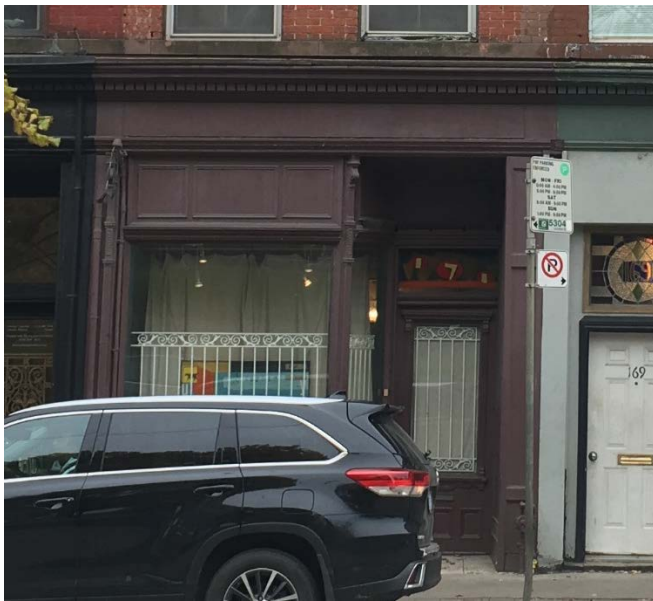
20. Shopfront at 171 Queen Street East showing the original design with the recessed entrance, the wood mouldings on the door and the bay window and the entablature and cornice with the dentil course (HP, 2019)
