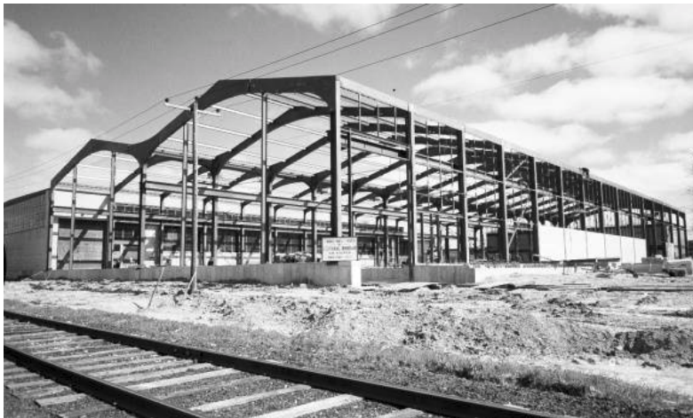
81 Barber Greene Road, 1957 view of the structural frame of the shed (CAC)
