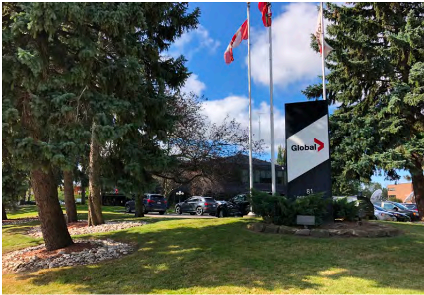
81 Barber Green Road looking north-west across the landscaped setting to the former office-manufacturing complex, now Global Television office and studios (HPS, 2019)
