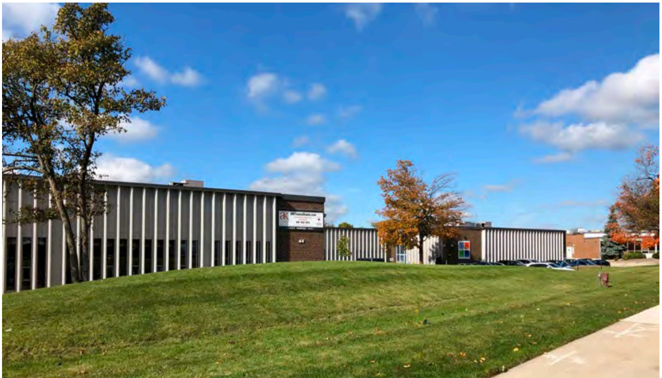
44-52 Prince Andrew Place, principal (east) elevations (Heritage Planning, 2019)
