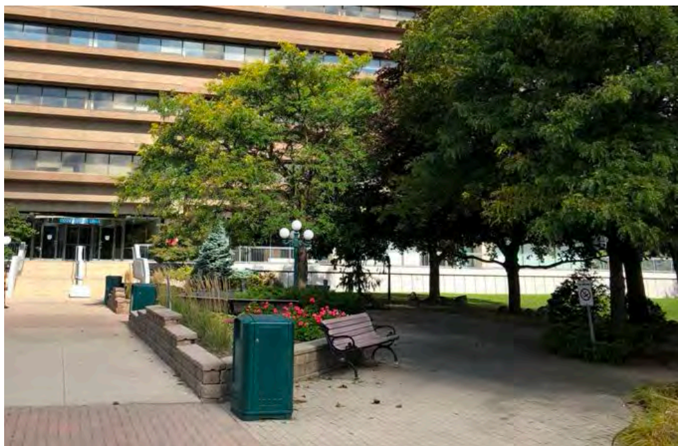
Two views of 100 Wynford Drive showing: the six-storey building on a raised platform in a deep landscaped set back from Wynford Drive (top), the planting area (altered since the original) between the side walk and the building (bottom) (Heritage Planning, 2019)
