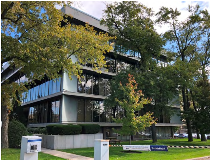
West elevation showing the recessed basement (HP, 2019)
