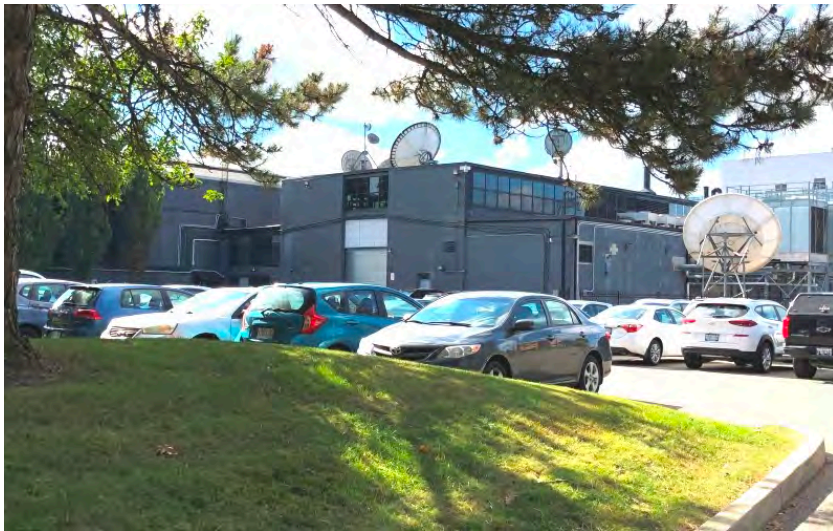
Barber Greene of Canada Ltd., showing the first 1954 structure with the north-east (front) and north-west (side) elevations in the mature landscape setting (HPS, 2019)
