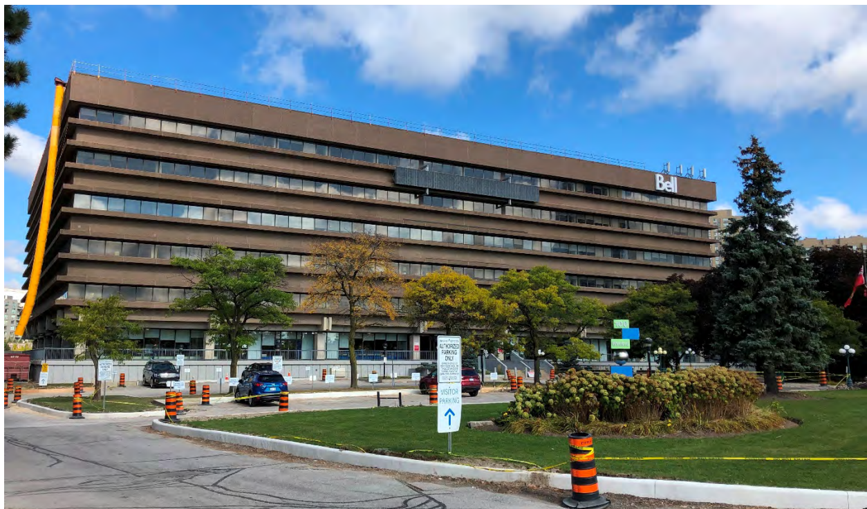
100 Wynford Drive: principal (south) elevation and landscaped setting with arrival driveway (Heritage Planning, 2019)
