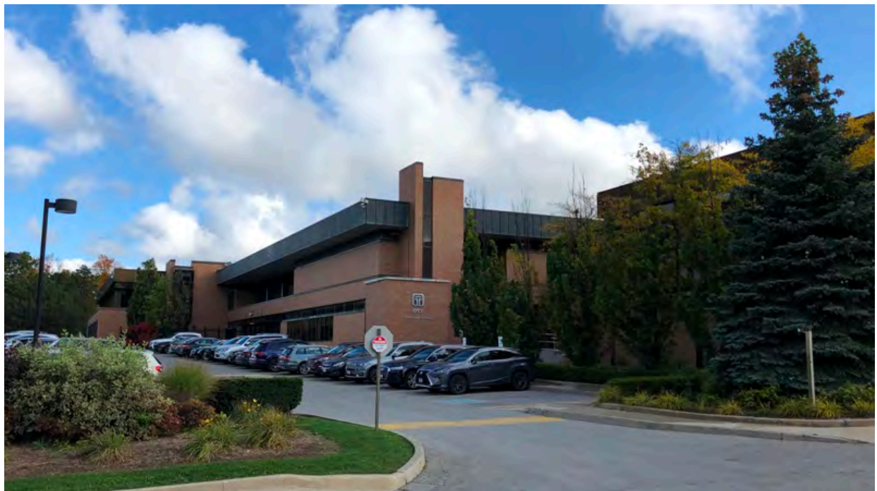
1123 Leslie Street, showing the principle west and south elevations (HP, 2019)
