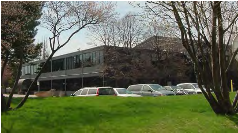
View of the office component building with the shed beyond showing the north-east (front) with new canopy at the entrance and north-west (side) elevations (HPS, 2004)
