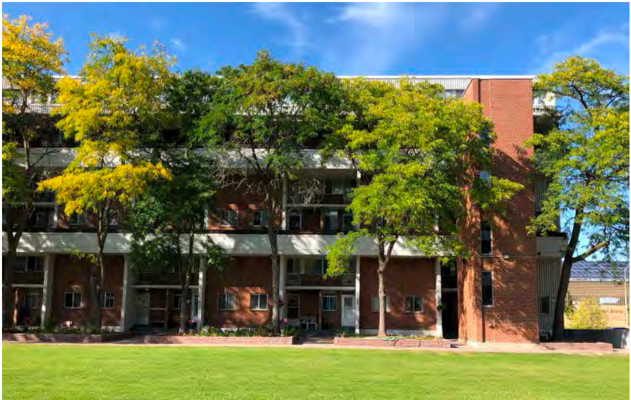
95-155 Leeward Glenway, north-east block, south elevation facing the playground, showing the 3 levels of two storey stacked houses the concrete sheer walls and walkways with brick cladding and the access stairs at the end of the block (HP, 2019)
