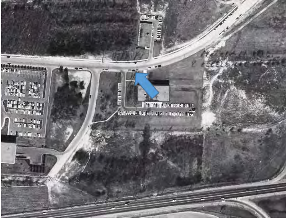
Aerial view 1967 looking north showing the extent of landscaping surround the property at 39 Wynford Drive and the allocation of the parking on the west side and south rear. (ASI)
