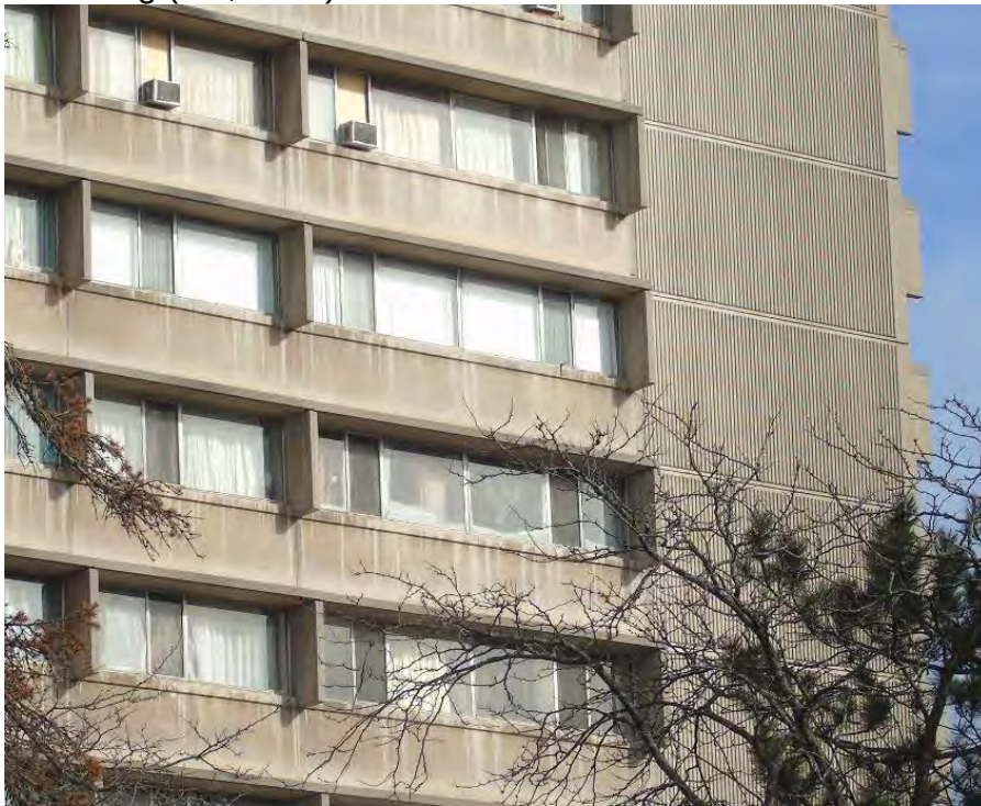
95-155 Leeward Glenway: showing the concrete details with the striated surface, smooth surface beneath the window and the projecting hoods over the windows (ASI, 2018)
