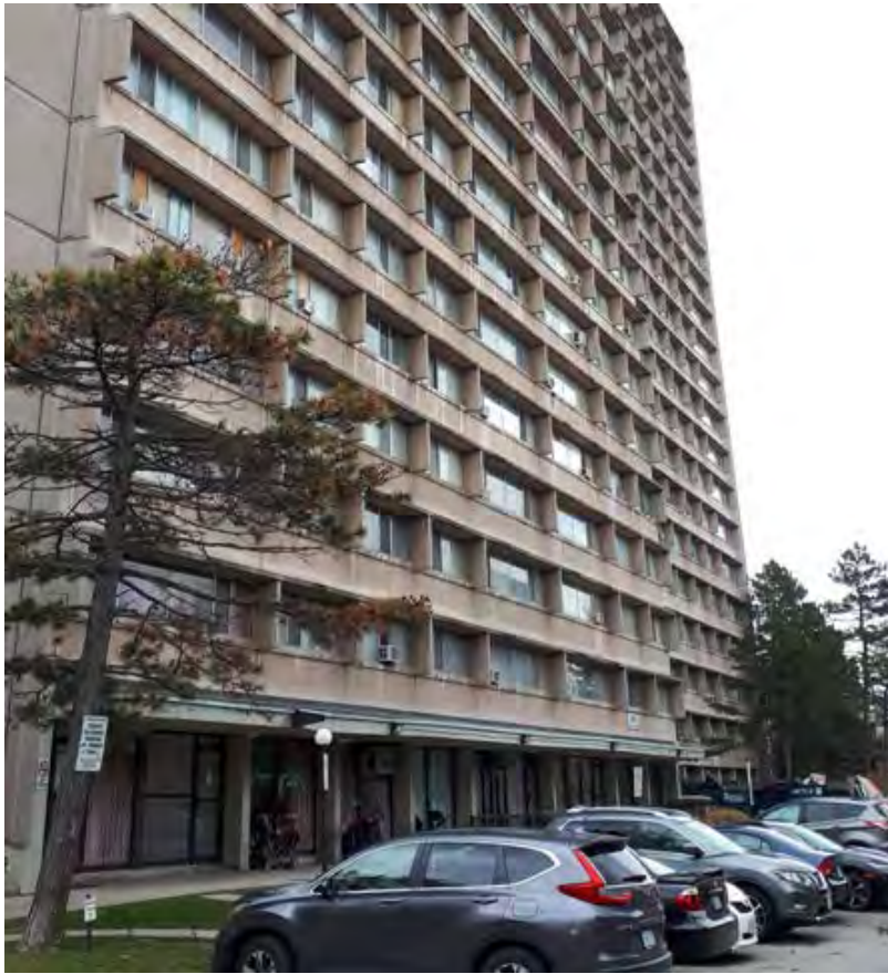
95-155 Leeward Glenway showing the base of the tower with the full-height glazing at ground floor level on the east side (HP, 2019)
