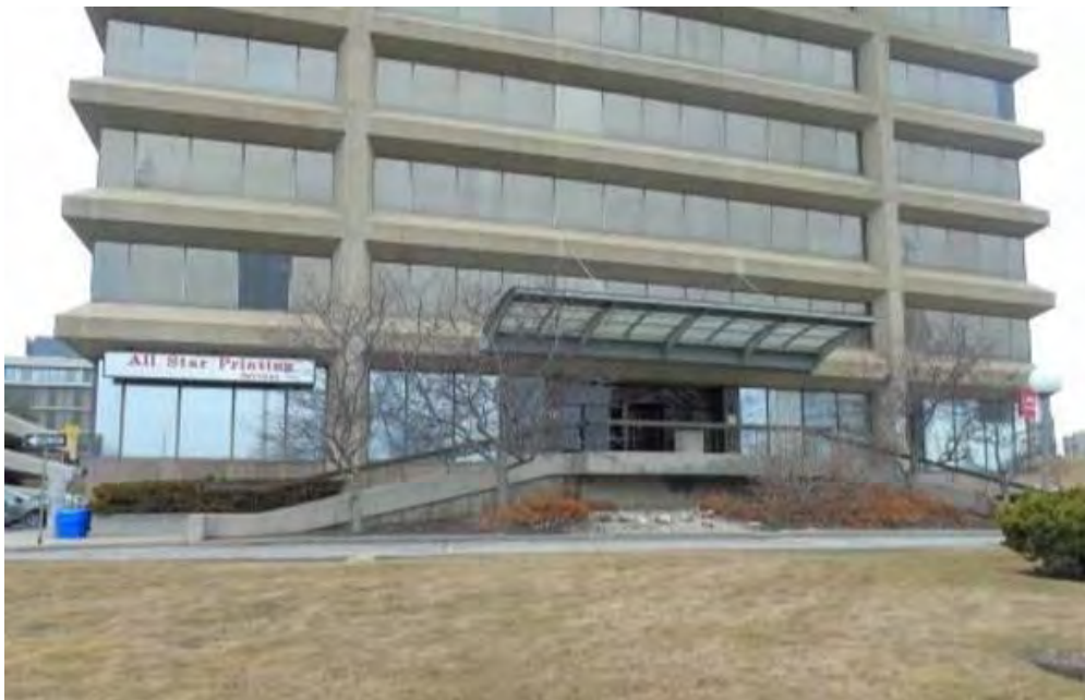
1200 Eglinton Avenue East south elevations with ramps to the main entry and the later entrance canopy (ASI, 2018)
