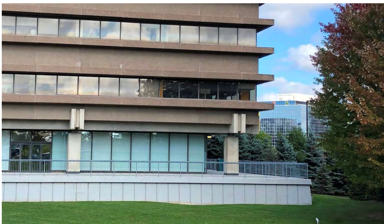
Two views of 100 Wynford Drive showing the steps up to the raised platform at the base of the building and the entrance (top) and a view of the details of the first floor piers and upper walls at the south-east corner of the building (Heritage Planning, 2019)
