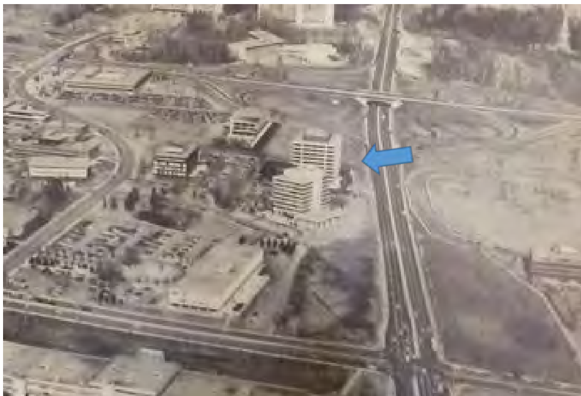
Aerial view 1969, looking east showing 1200 Eglinton Avenue East and adjacent low-rise properties developed along Wynford Drive (ASI)
