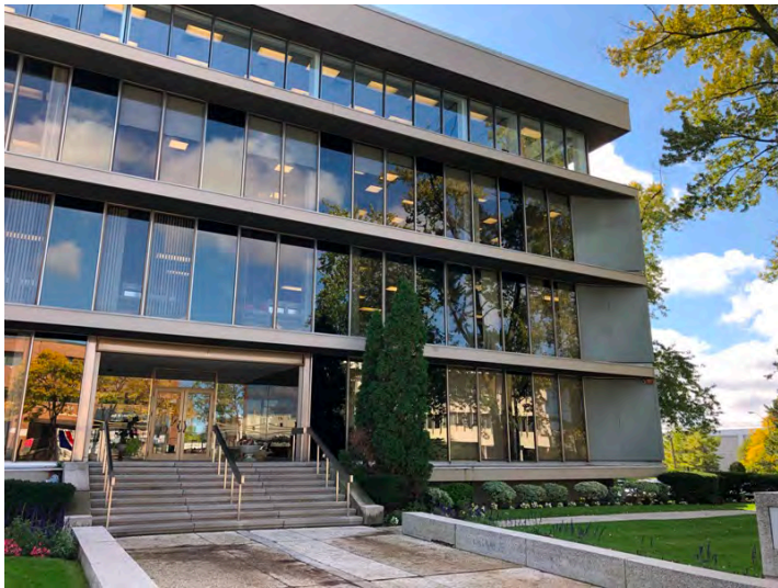
Principal (north) elevation showing the entrance with the canopy removed and the corner detail (HP, 2019)
