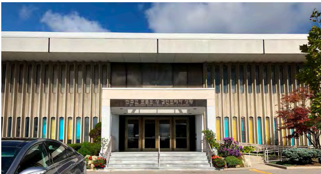
Detail of the south elevation showing the principle entrance with the portico (HP, 2019)
