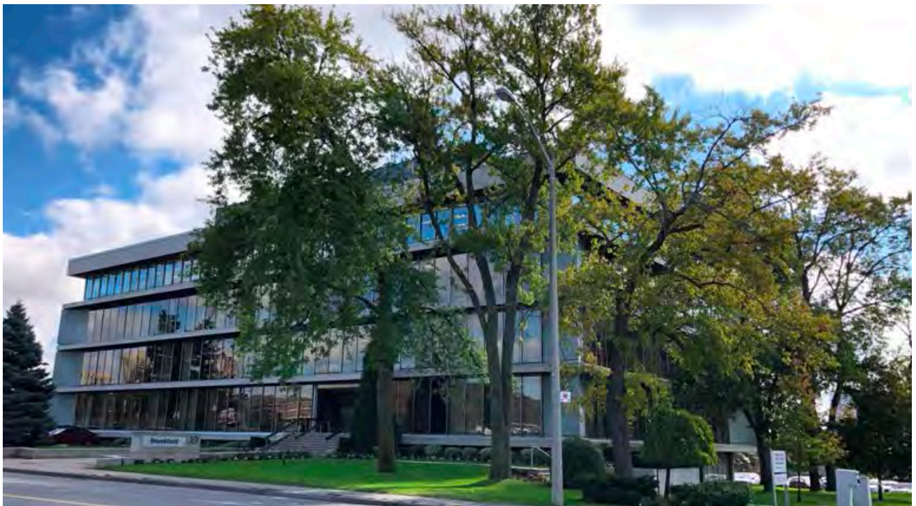
39 Wynford Drive, principal (north) elevation facing Wynford Drive (Heritage Planning [HP], 2019)
