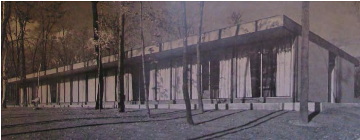
Early photograph showing the building with screen of tall trees on the front (west) side of the property and the original narrow south end wall with single entrance opening (ACO – TO Built, source uncredited)
