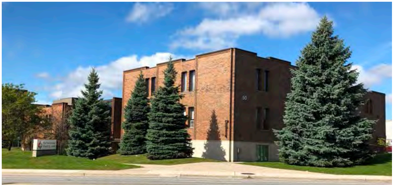
50 Wynford Road, principal (south) and side (east) elevations facing Wynford Road (Heritage Planning, 2019)
