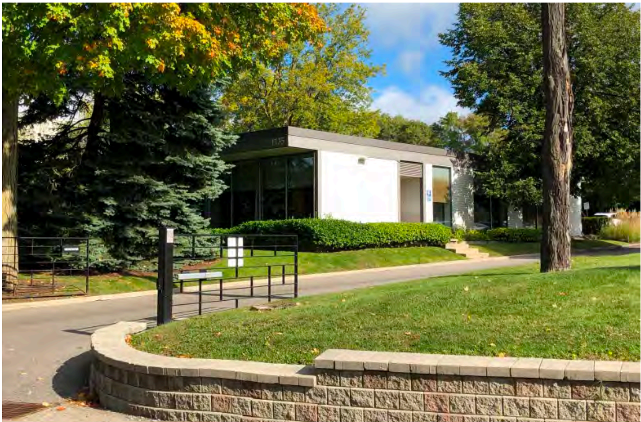
1135 Leslie Street, view of the corner of the principal (west) elevation and the side (south) elevation with its addition to the right. N.B. the gates are a later addition (HP, 2019)
