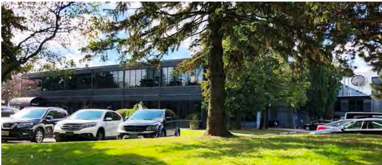
View of the 1957 office component building with the shed beyond showing the north-east (front) elevations and a portion of the 1954 building to the right (HPS, 2019)
