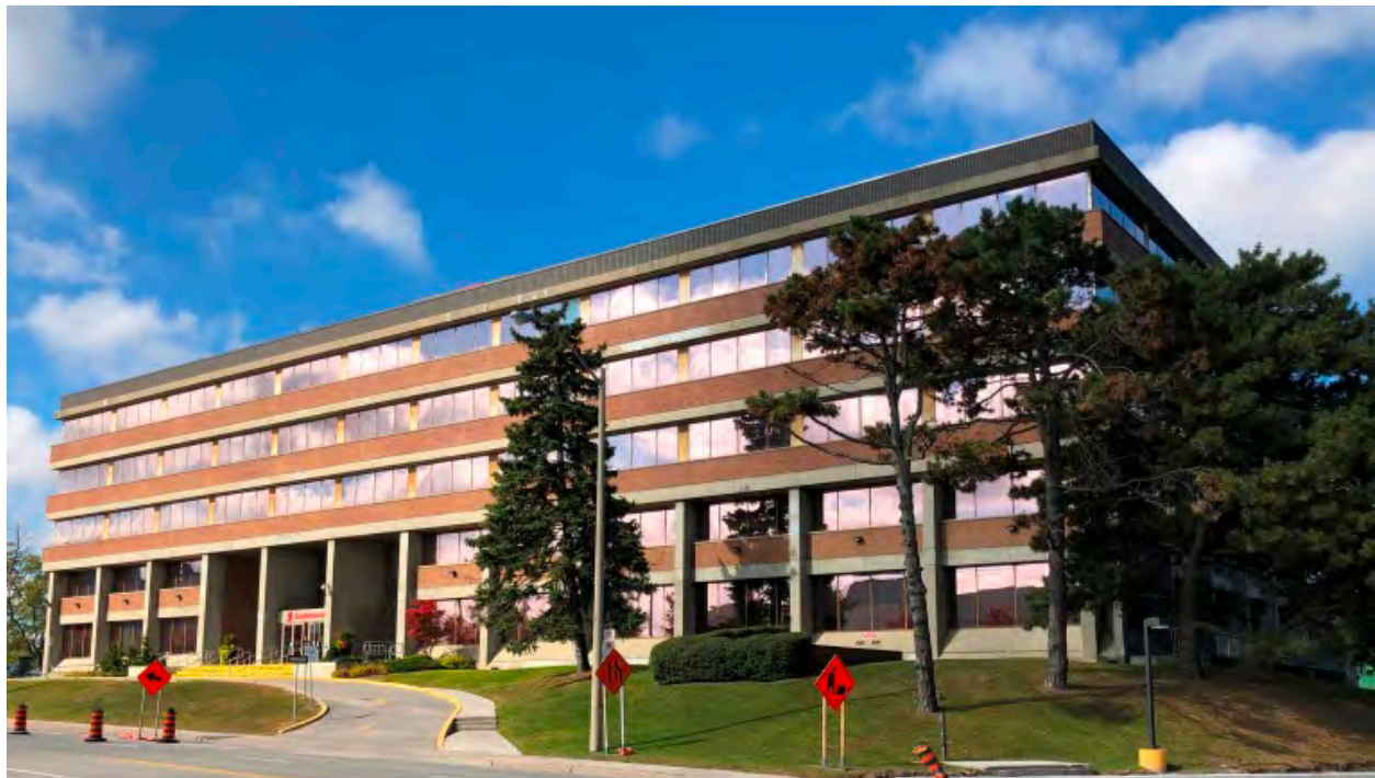
90 Wynford Drive: principal (south) elevation and landscaped setting (Heritage Planning, 2019)
