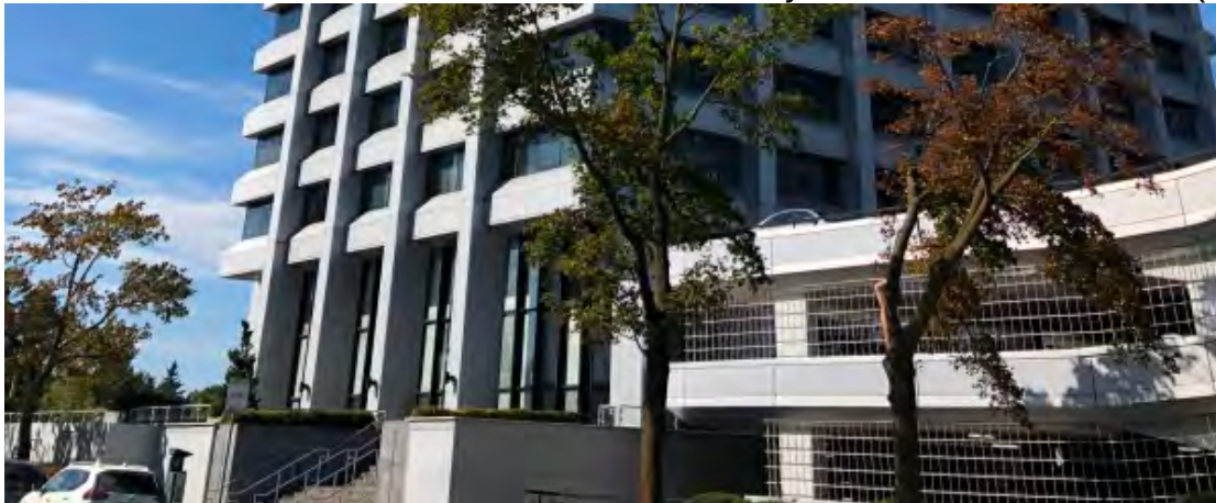
789 Don Mills Road: view of the south elevation of the building from Rochefort Drive showing the raised plaza and the adjacent parking structure (HP, 2019)
