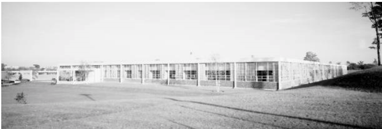
1958 view of the Grand & Toy Ltd. premises showing the principal elevation and the side (west) elevation with the landscaping with the hill on the west side (CAA, 55230-5)
