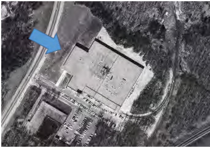
1123 Leslie Street aerial photograph, 1963, showing the original configuration of the premises with the small office volume to the west and large plant behind with parking on the south and access to the CNR line to the east (City of Toronto aerial photography)
