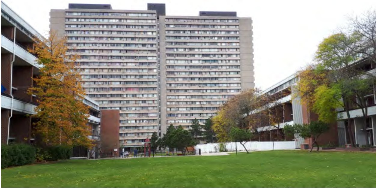
95-155 Leeward Glenway looking west from the open space and play ground to the pair of high-rises (HP, 2019)
