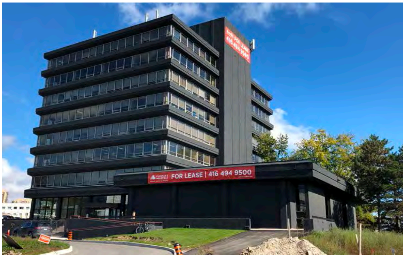
15 Gervais Drive, west and south elevations following the painting of the concrete walls in 2017 (Heritage Planning, 2019)
