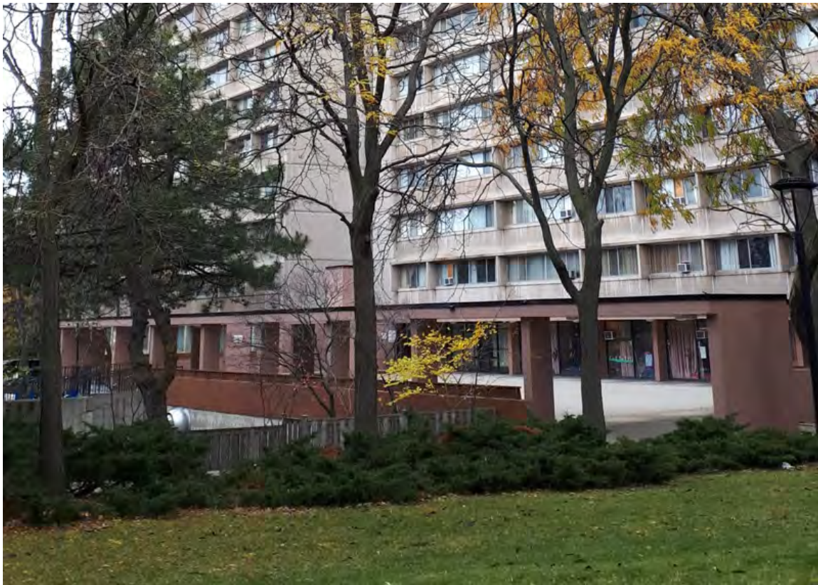
95-155 Leeward Glenway showing the west side of the pair of towers with their landscaped setting and plaza with the enclosing low wall plains and loggia type screening (HP, 2019)
