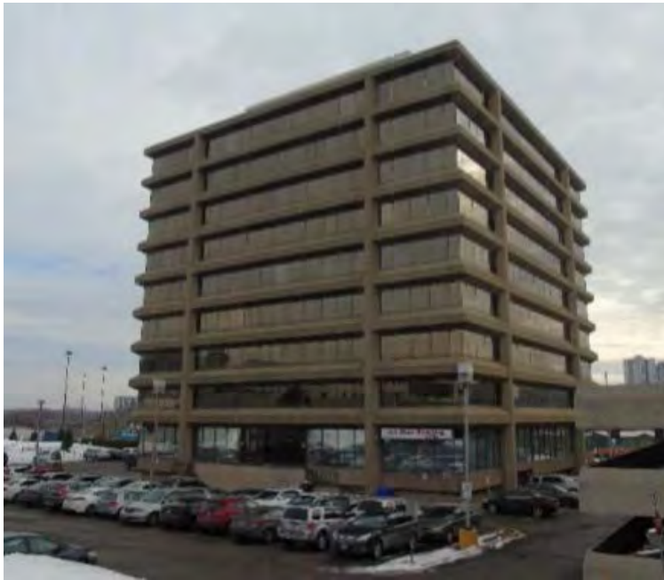
1200 Eglinton Avenue East: view of the north and west elevations (ASI, 2018)
