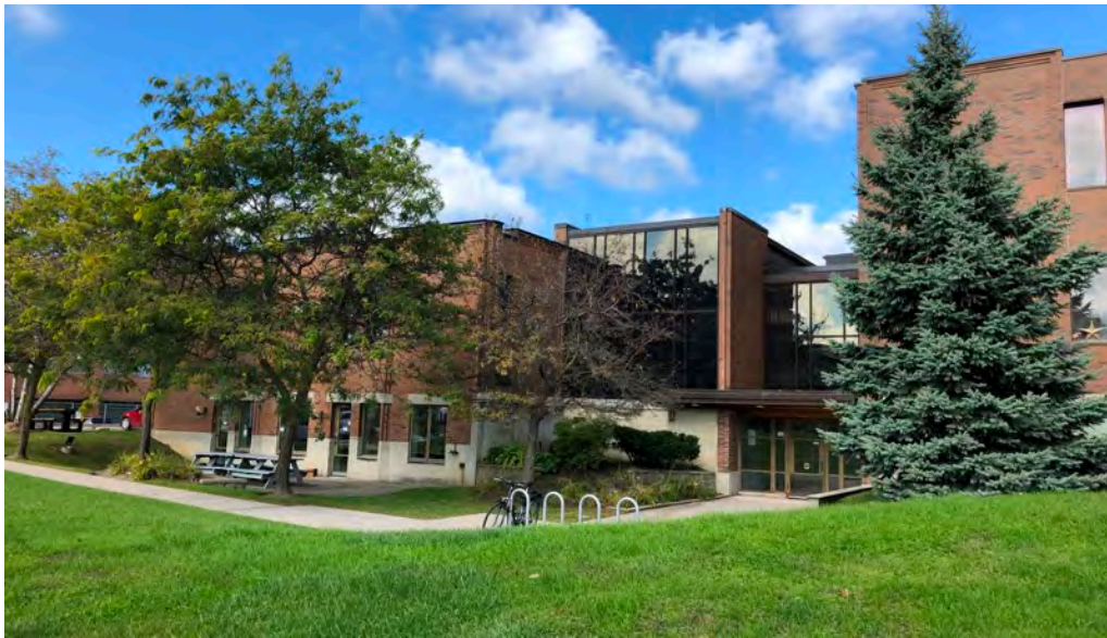
50 Wynford Drive showing the current entrance configuration which is one level lower following the removal of the upper level court originally screened by the perforated brick wall which provided at grade access and revealed the basement level (Heritage Planning [HP], 2019)
