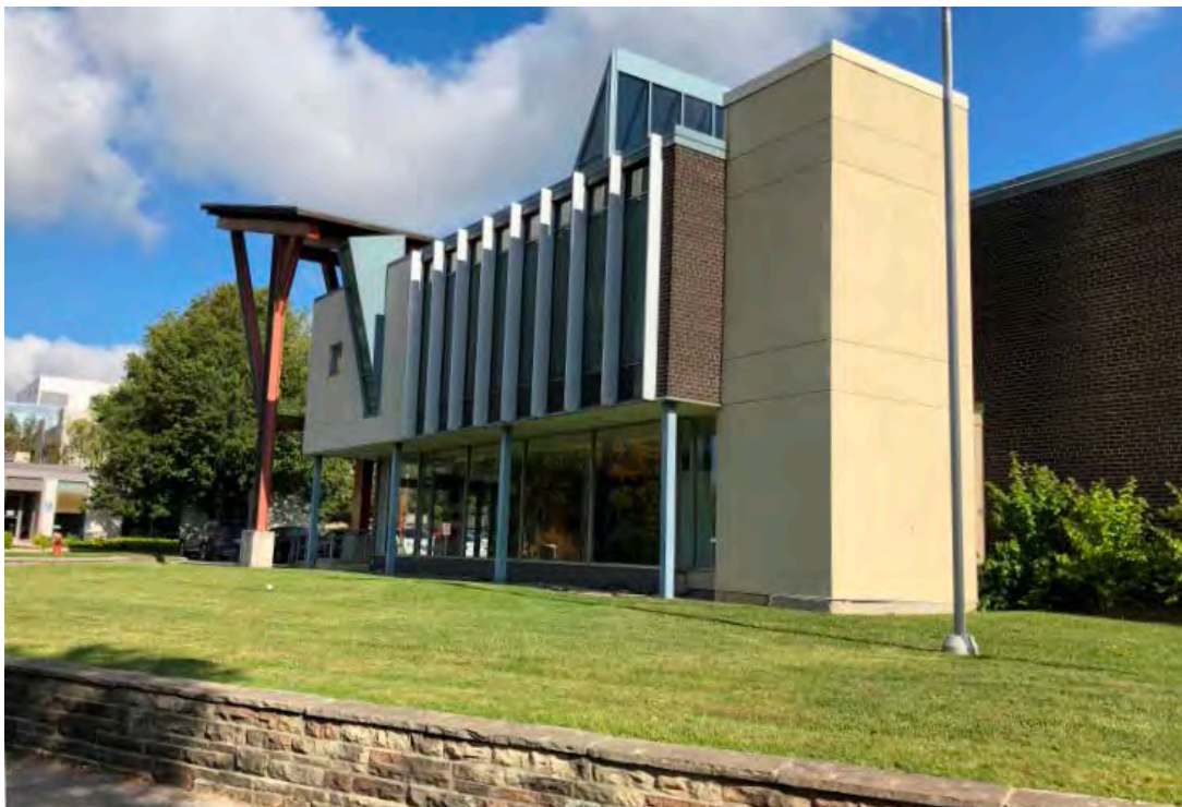
1133 Leslie Street showing the principal (south) elevation with the new elevator in the light cladding at the right (HP, 2019)
