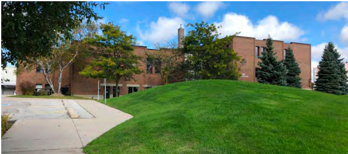
50 Wynford Drive, principal (south) elevation viewed from the west (HP, 2019)
