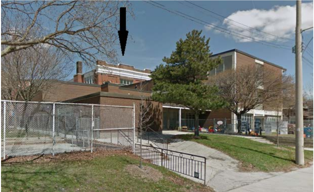
Original south elevation of Kent School at 90 Croatia Street (980 Dufferin Street) behind addition
