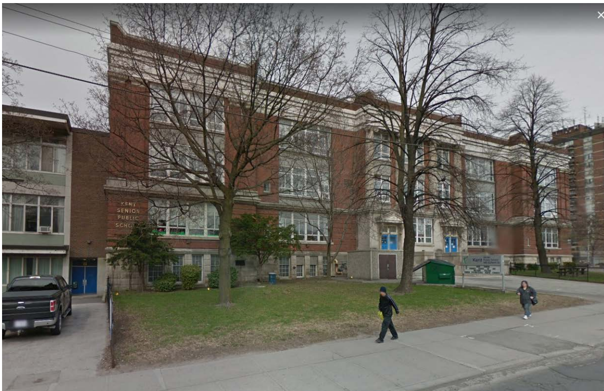
East elevation of Kent School at 90 Croatia Street (980 Dufferin Street)
