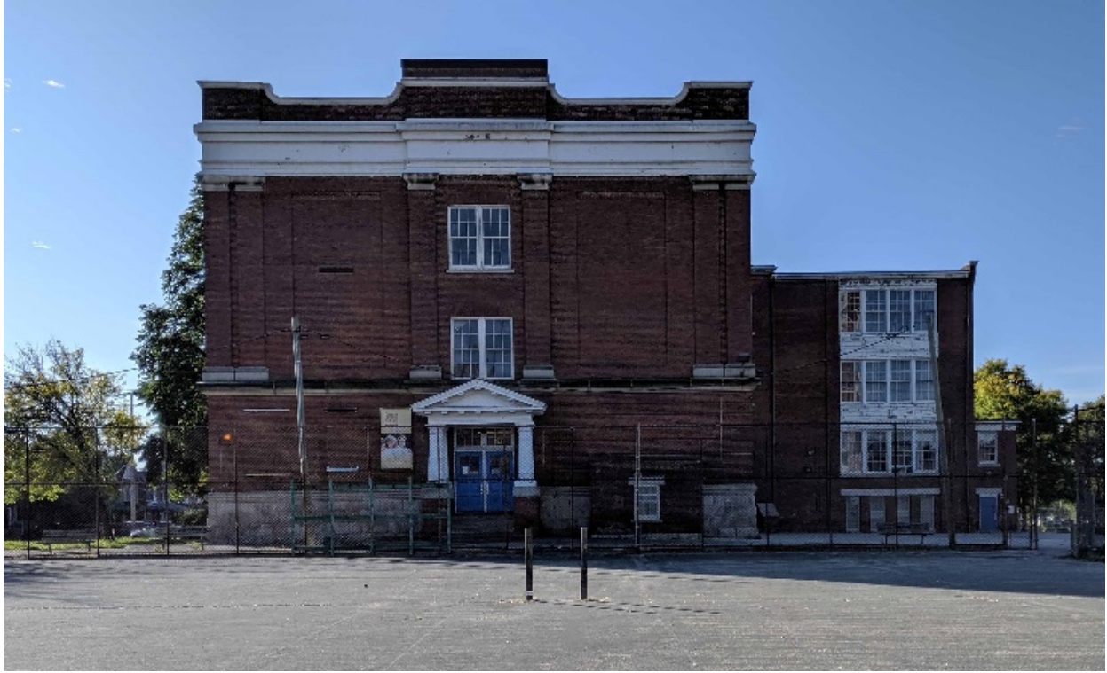
North elevation of Kent School at 90 Croatia Street (980 Dufferin Street)
