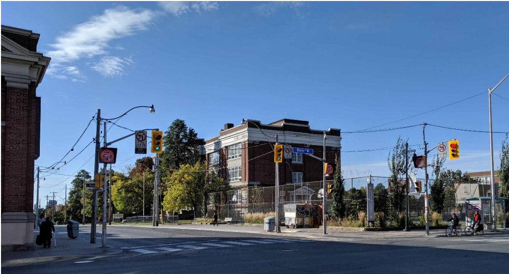
5a. Contextual view of the Kent School looking south from the intersection of Bloor and Dufferin streets, with the principal (east) elevation on the left
