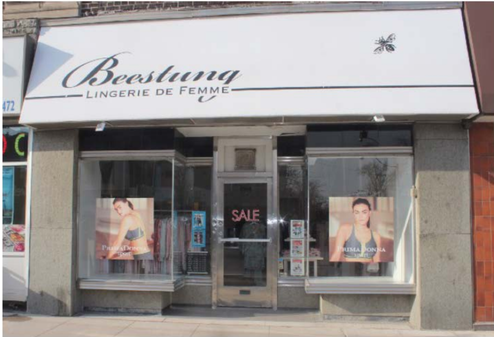
View (facing west) of the primary east elevation of the existing property, including the Art Deco-style storefront at 2504 Yonge Street
