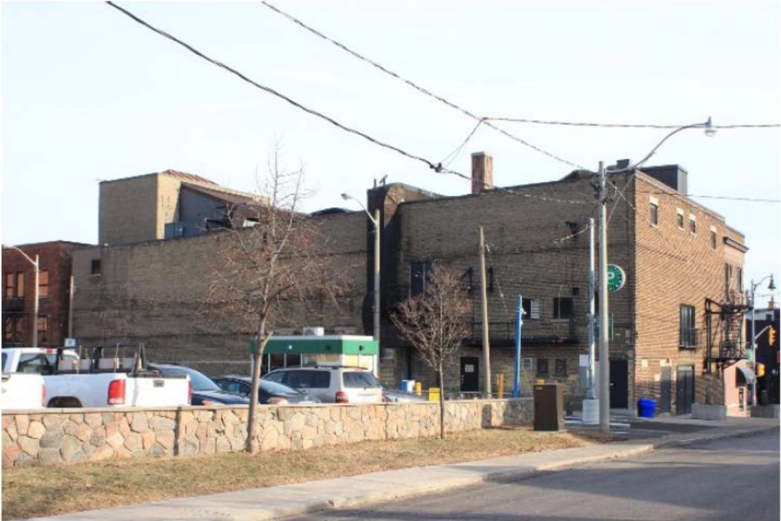
View (facing east) of the existing property's west (rear) elevation
