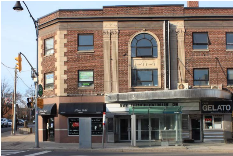
View (facing west) of the primary east elevation of the existing property, including the Art Deco-style theatre marquee and entrance
