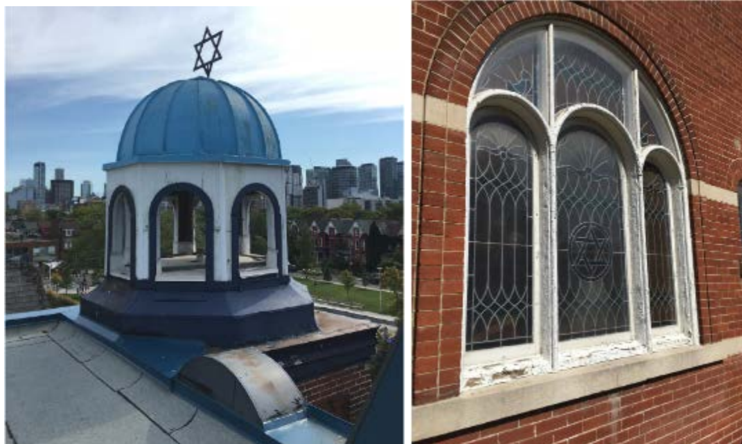
Cupola (left) and south elevation window showing typical signs of deterioration.
