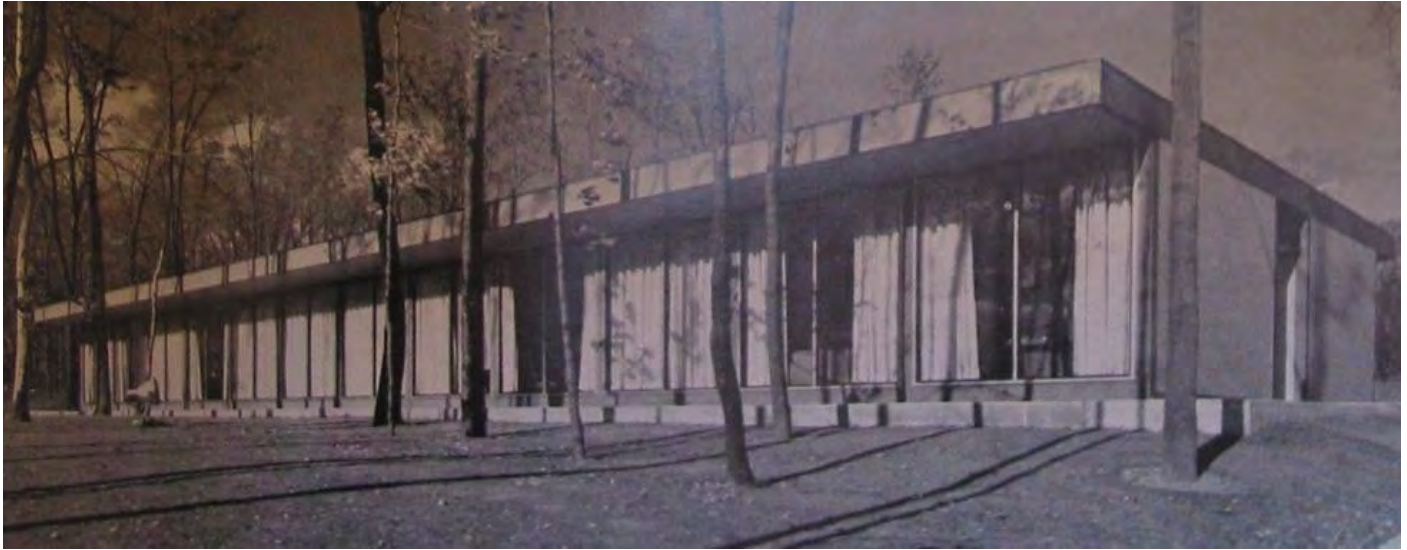
4. West elevation from the south end of the building showing deep overhanging eaves, glazing and surrounding deck, undated (A.C.O. T.O. Built, source uncredited).
