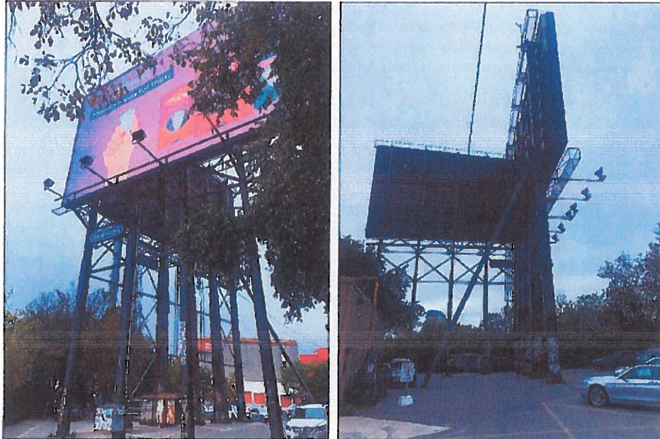
Figure 1 – Existing third party ground sign at 2 Atlantic Avenue
