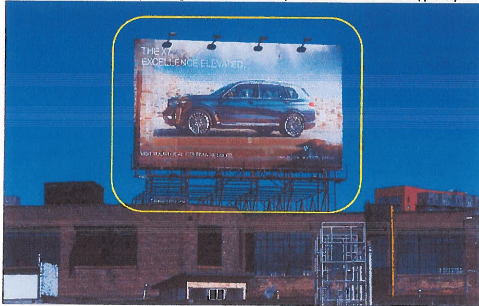
Figure 3 – Existing Third Party Roof Sign at 7 Fraser Avenue (removed as a condition of approval)
