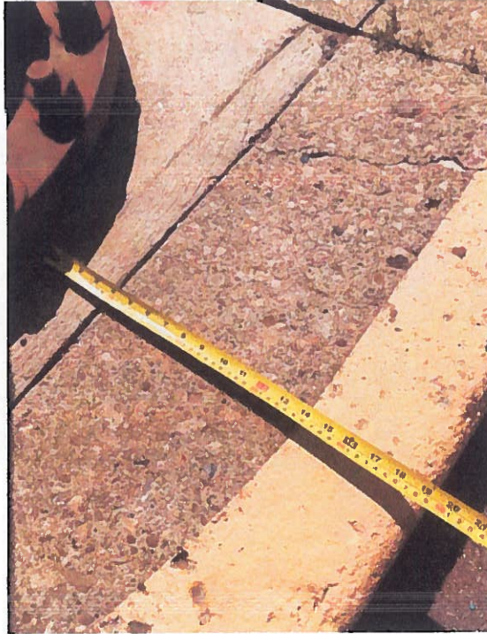
Image #14: A Picture Of The Measured 19 Inches (0.48 meter) Setback From The "Accessible Parking Spot"
