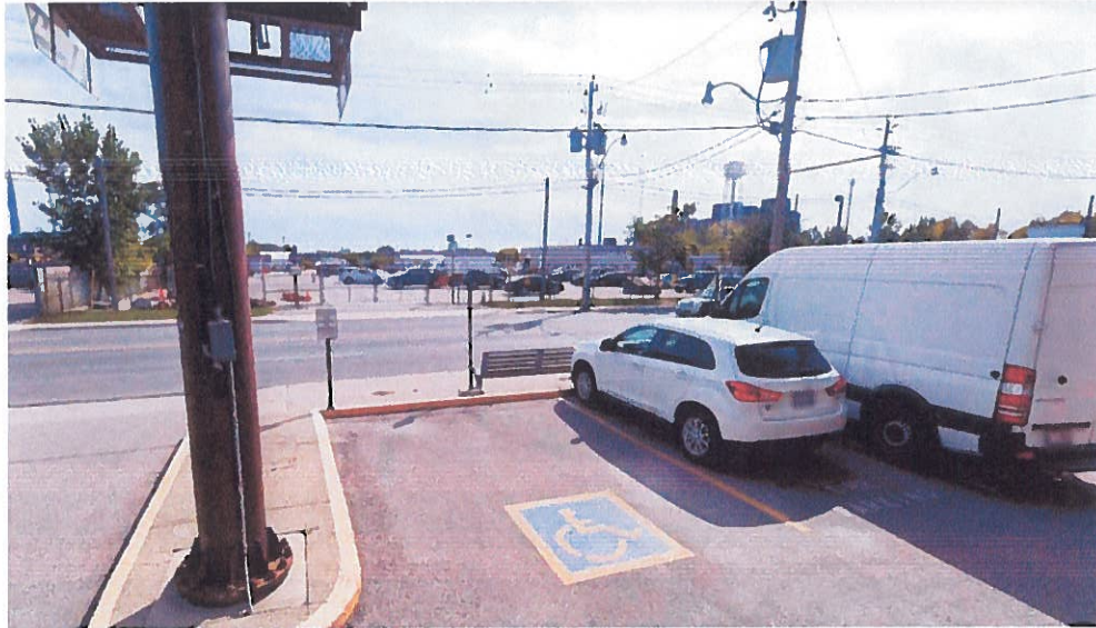
Image #13: A Picture of “Accessible Parking Spot” Relative To Our Sign Support Column.
