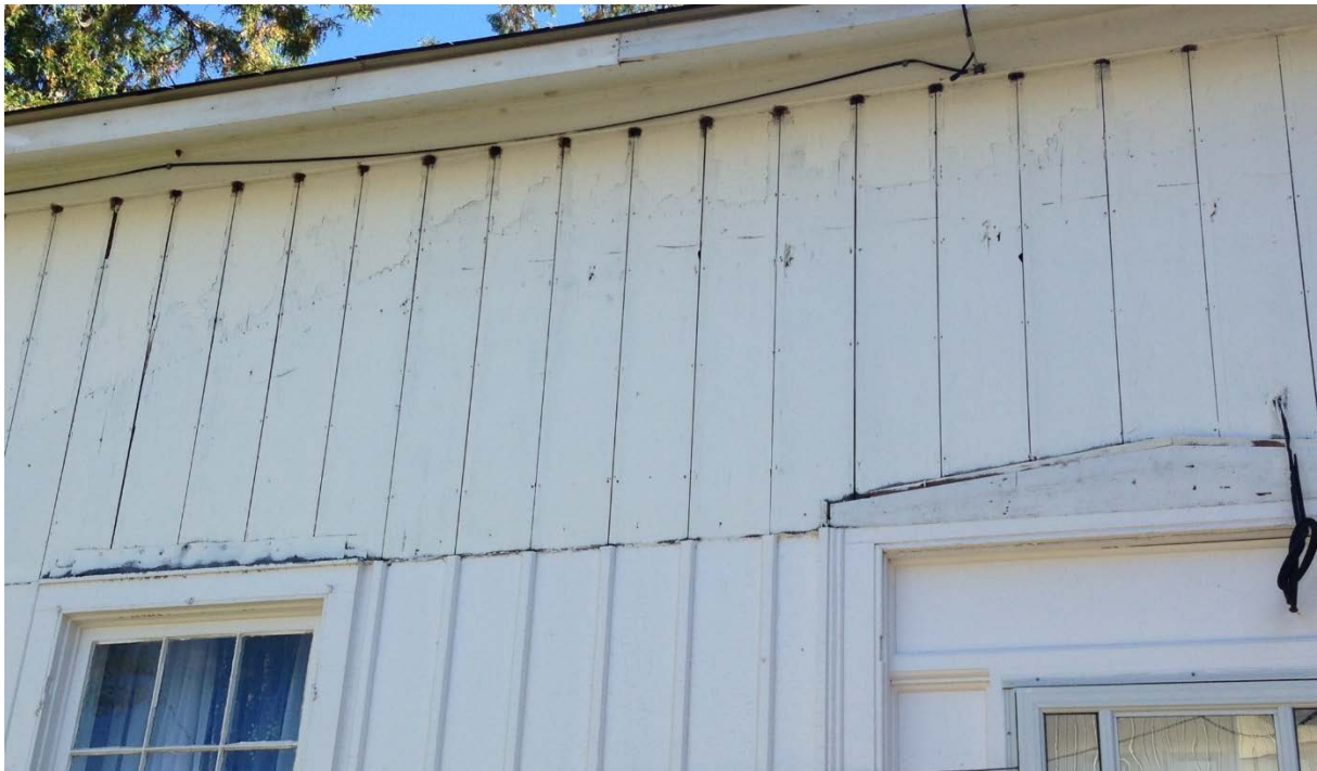
19. West elevation, showing the angled line of different paint indicating the roof line of the verandah and the missing board and battens above (HPS, 2017)
