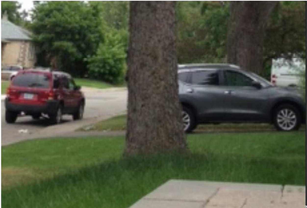
Figure 3: July 12, 2019 Staff photograph showing the root flare of the Colorado blue spruce tree measuring 51 cm in diameter.
