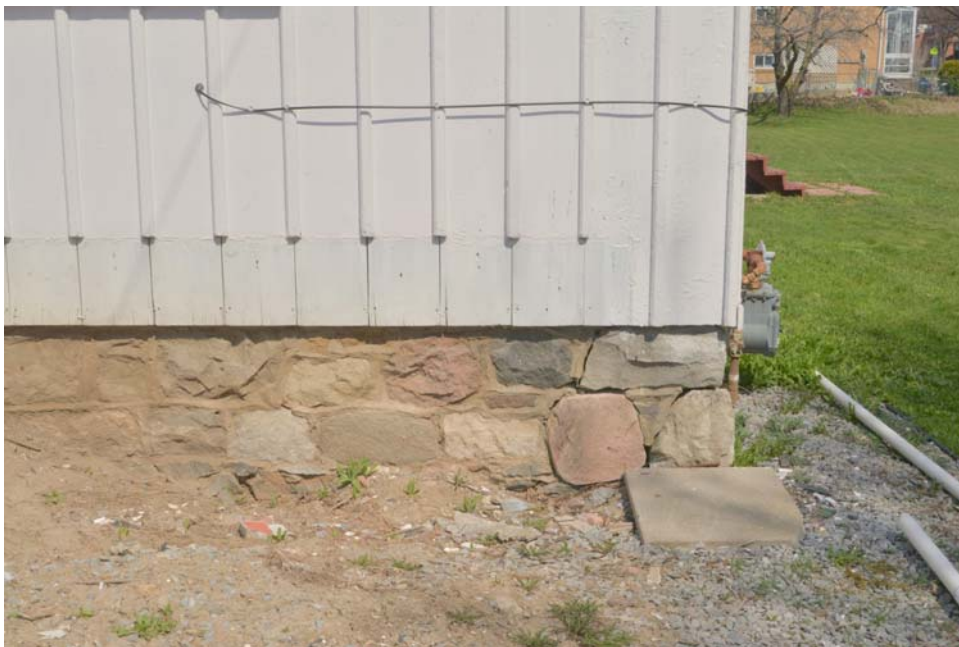
Fig. 20 Rubble stone foundation and evidence of former verandah
