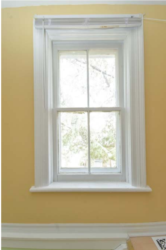
Fig. 60 North-facing window at top of stairs
