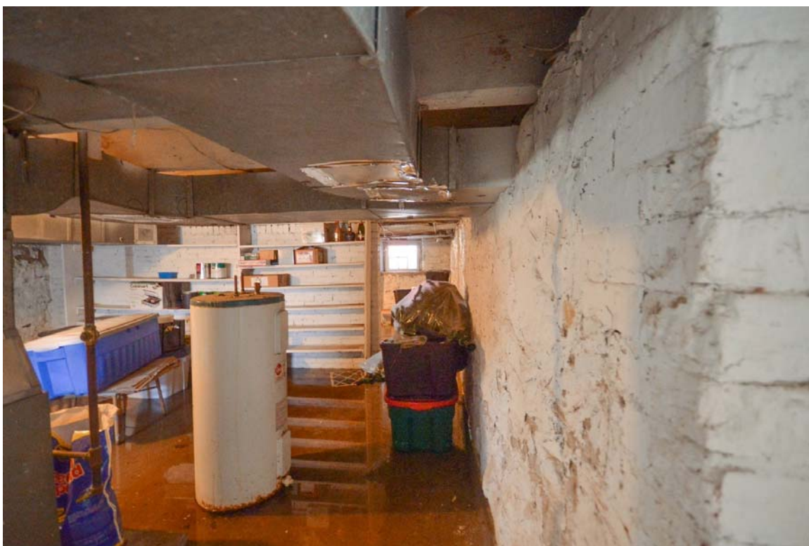
Fig. 68 Cellar, looking north
