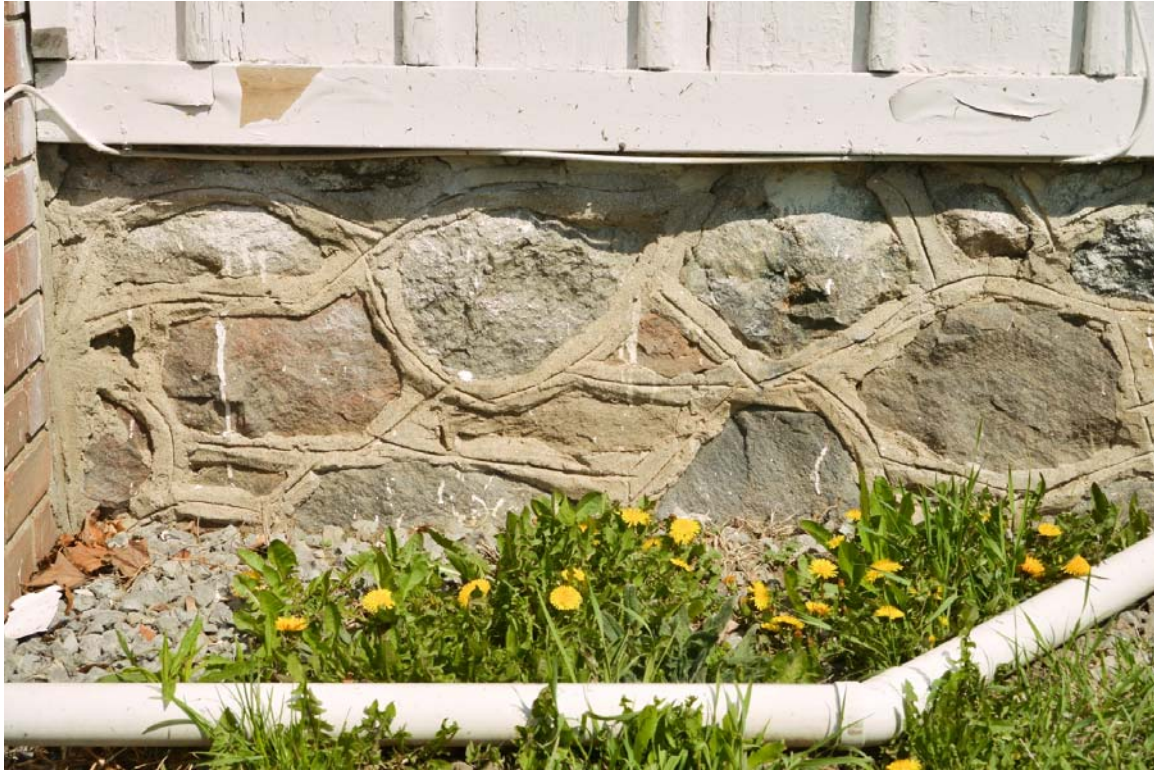
Fig. 42 South elevation rubble stone foundation wall beside chimney
