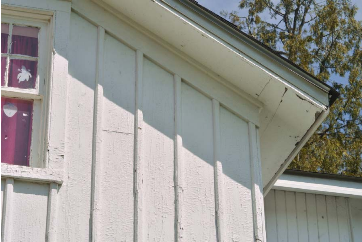
Fig. 46 South elevation detail of board-and-batten siding, plain cornice and simple eaves
