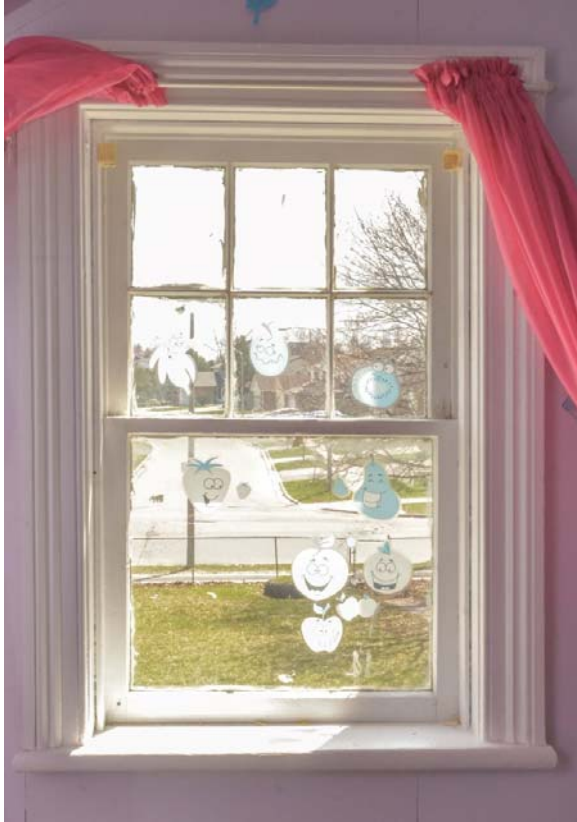
Fig. 64 South-facing window in southwest bedroom
