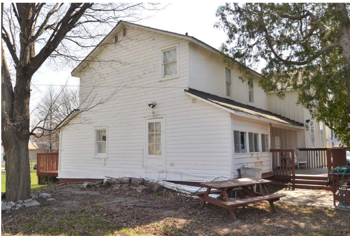
Fig. 32 Corner view, showing east and north elevations
