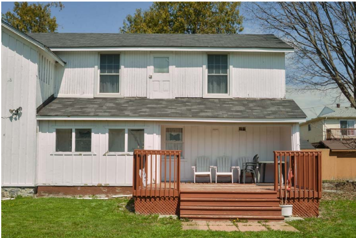
Fig. 47 Back wing's south elevation
