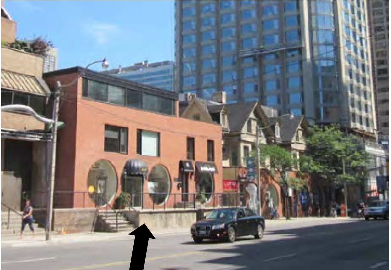
At Avenue Road frontage, 1960s buildings to be demolished.
