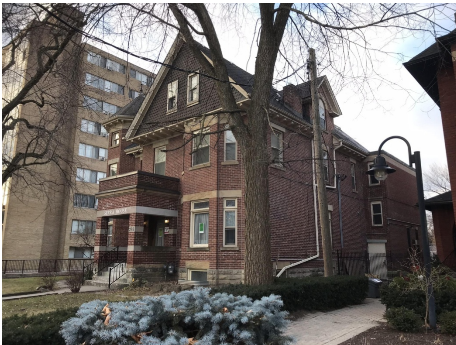
Photograph showing the principal (east) and north elevations of the George Gooderham House at 226 St. George Street, looking southwest (Heritage Preservation Services, 2018)
