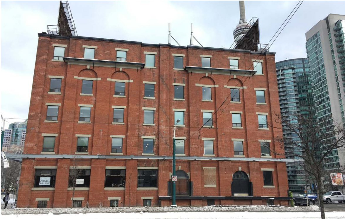
View of the west (Spadina Avenue) facade of the Steele Briggs Building (ERA Architects)
