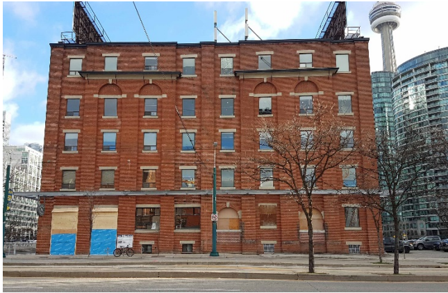
5a. West elevation on Spadina Avenue;
