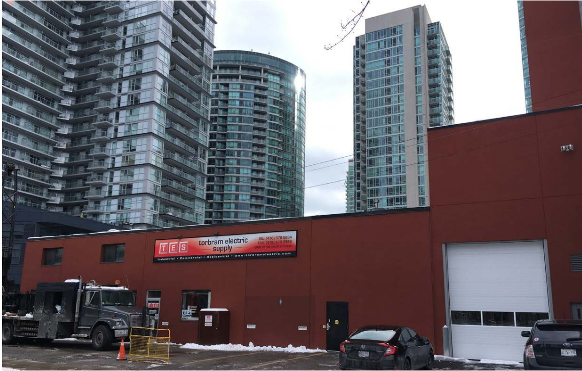
View of the north wall of the low scale addition on the eastern edge of the Steele Briggs Building (ERA Architects)
