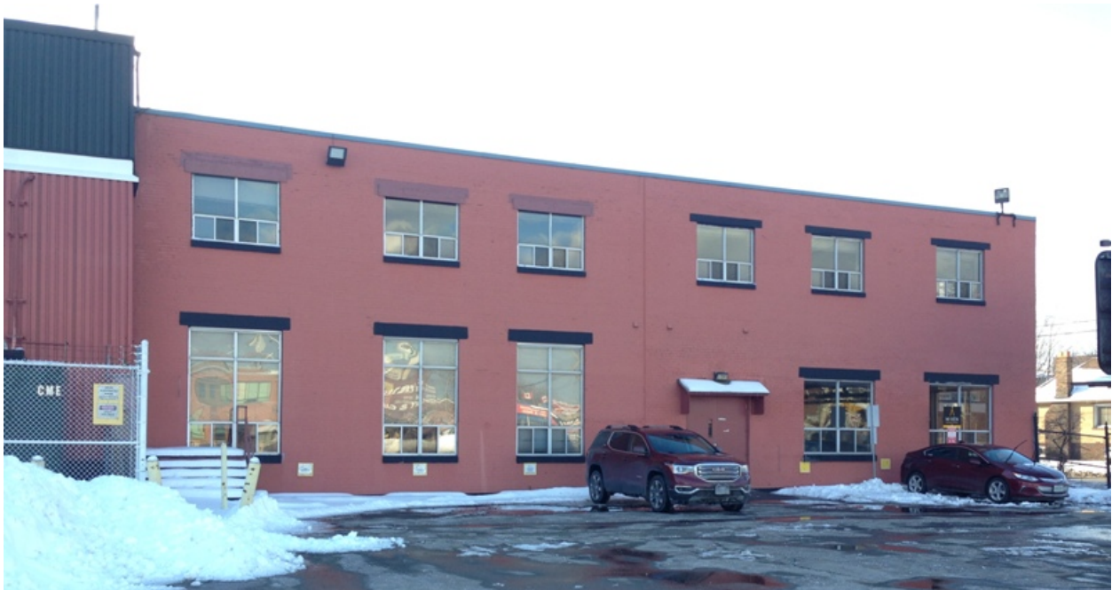
26. Comfort Building (E), east elevation, showing the original 1930 one-story building (bottom right), the 1946 upper story (top right) and the 1949 two-storey extension (left) (HPS, 2018)
