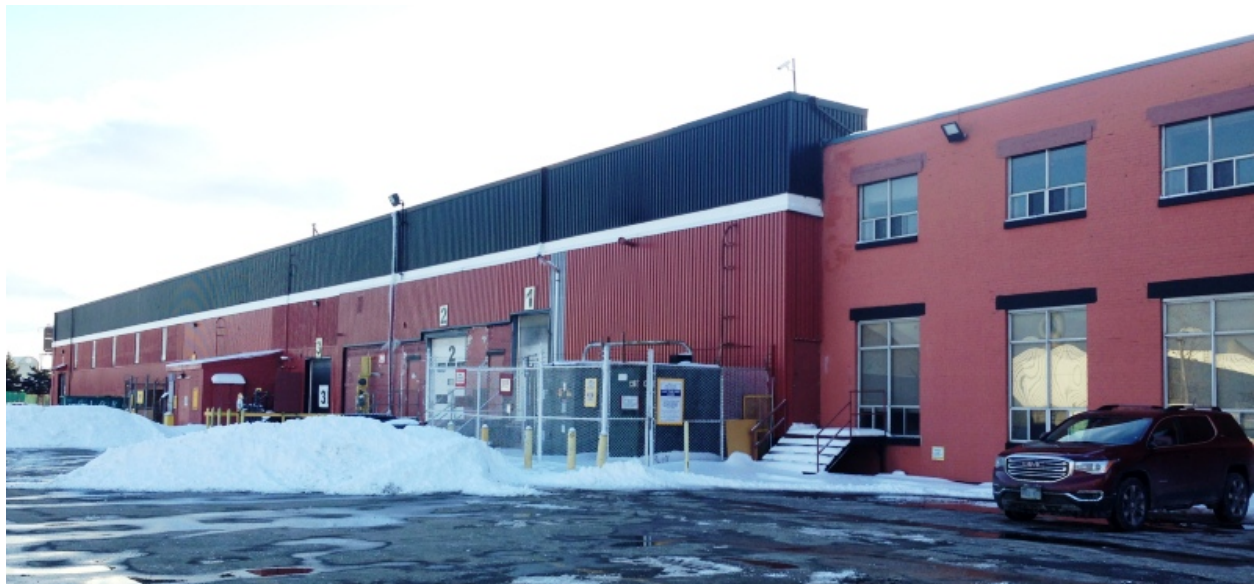
38. Building D: photograph showing the east elevations of Building D (left) and the Comfort Building (E) (right) (HPS, 2018)
