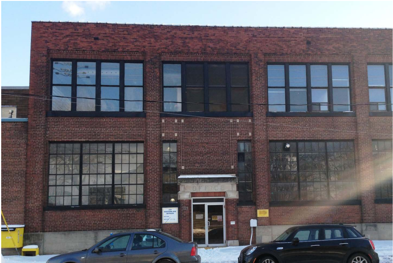
40. Main Building (A), principal (north) elevation, east end with entrance showing the factory sash glazing at the ground floor and double paned sash above (HPS, 2018)
