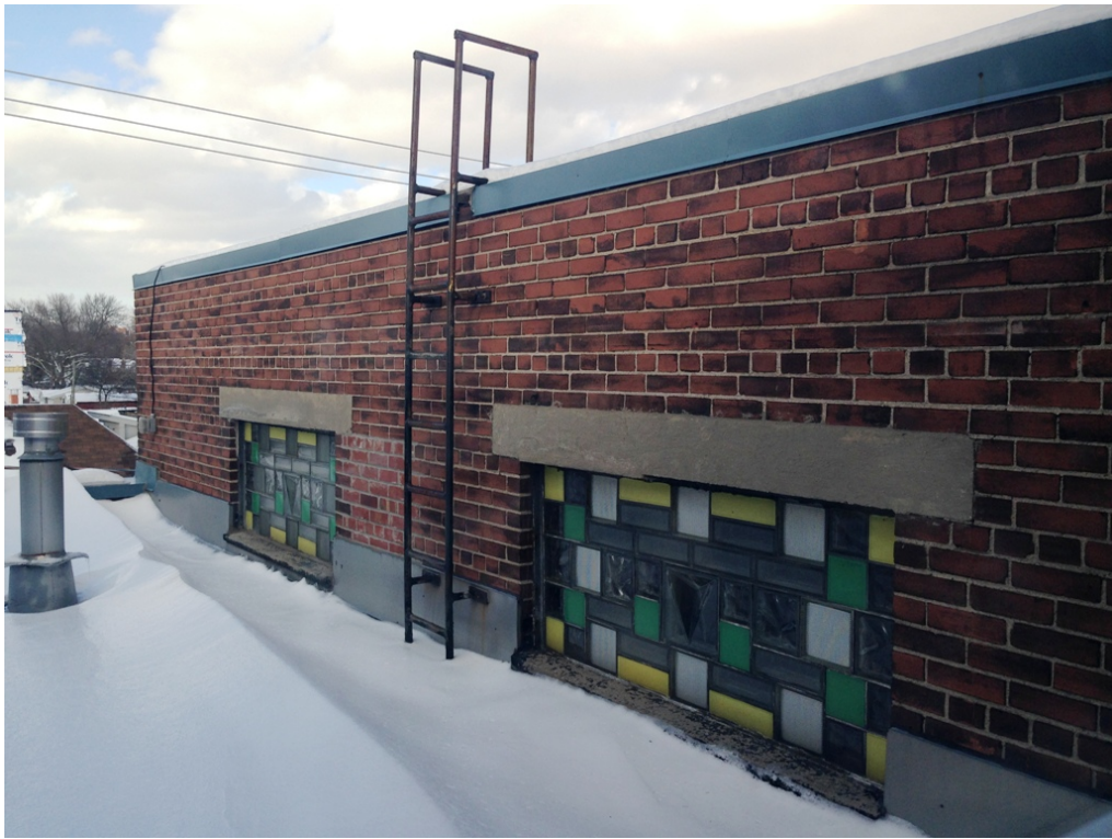
28. Exterior View of the upper side (west) elevation of Building E showing the location of the coloured glass block panels (HPS, 2018)
