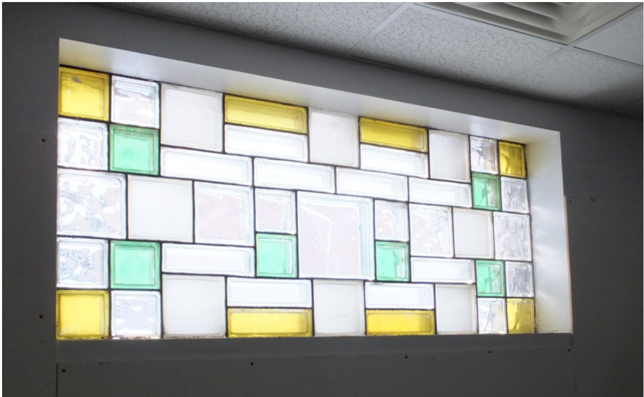
27. Comfort Building E, interior second floor showing one of two glass block panels (HPS, 2018)
