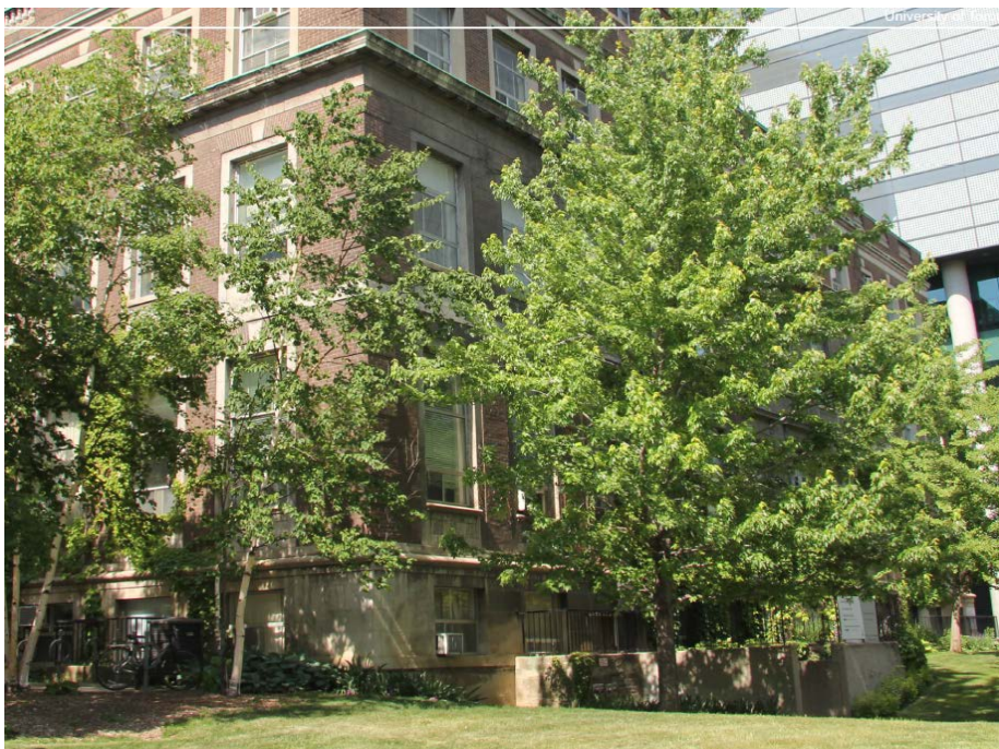
South West corner of building, proposed location of new plinth entrance.
