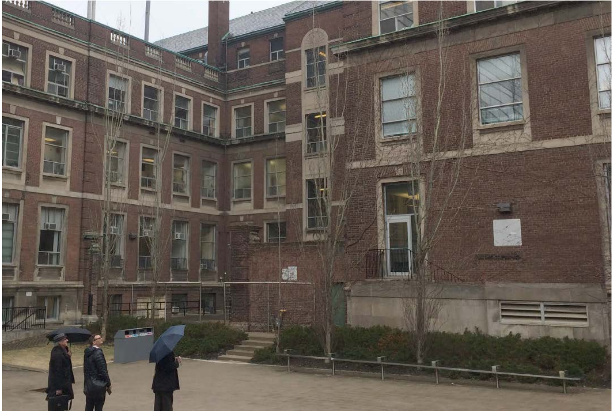
East elevation, location of infilled courtyard. Elevation faces west elevation of Pharmacy Building
