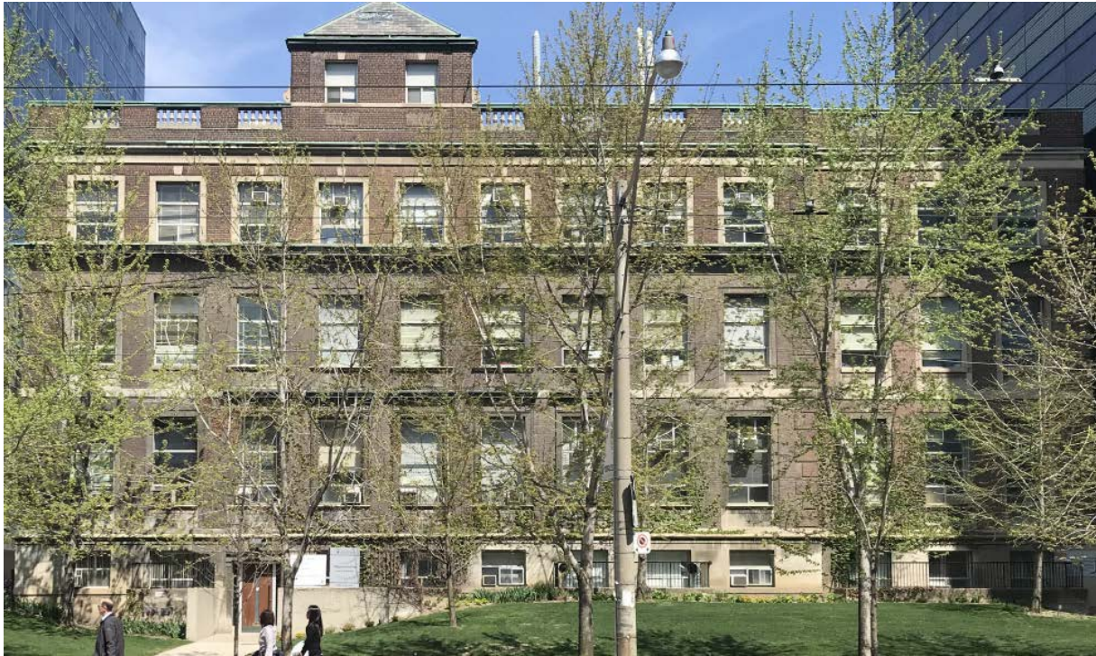
South Elevation of 150 College Street
