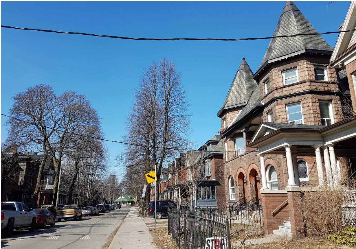
3c. Contextual view, looking west on Langley Avenue from 28-30 Langley (right) to Broadview Avenue where the St. Matthew's Lawn Bowling Clubhouse (a designated heritage building relocated from Gerrard Street East) terminates the vista
