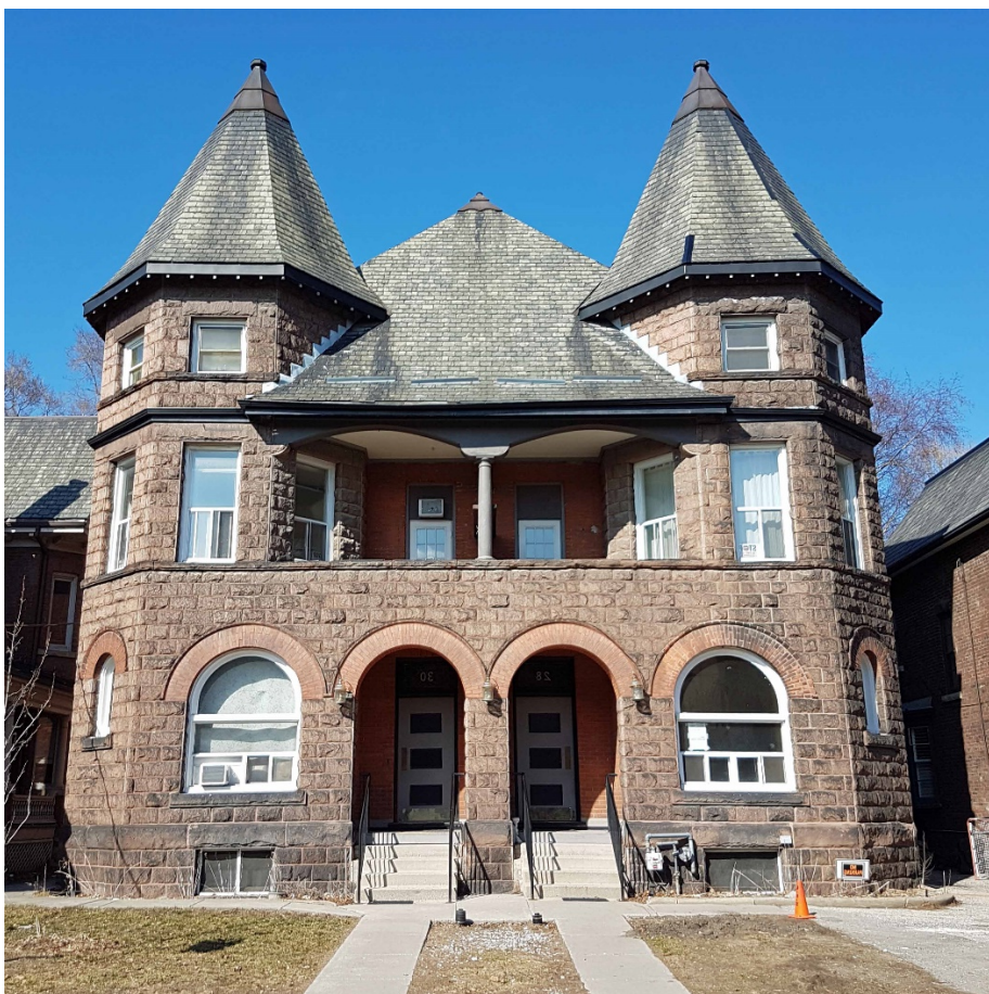
Principal (south) elevations of the William C. Jones Houses (Heritage Preservation Services, March 2019).
