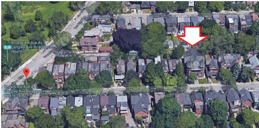
Aerial photograph showing the location of the property at 28-30 Langley Avenue, east of Broadview Avenue ( www.google.ca/maps )
