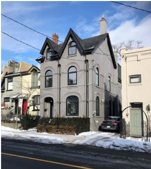
28 Belmont Street, principal (south) and side (east) elevation [HPS, March 2019]
