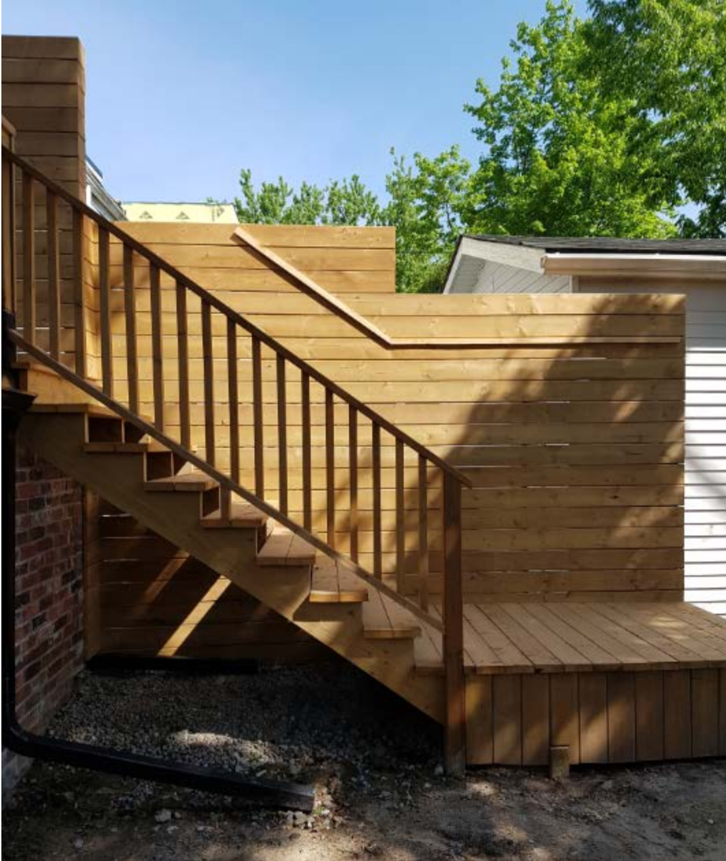
Existing fence taken from the property of 75 Alton Avenue, showing the fence was built from grade
