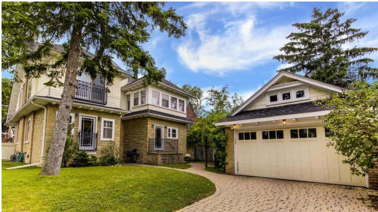
10. Photograph showing the garage and the side (east) and rear (north) elevations, with the two rear additions. The one to the right, towards the western edge of the north elevation is likely an original element of the Hill House as it includes the distinctive roof skirt and would typically have been built over an open verandah accessed from the kitchen. See also Images 15 and 16. (Richard Koroll, 2015)
